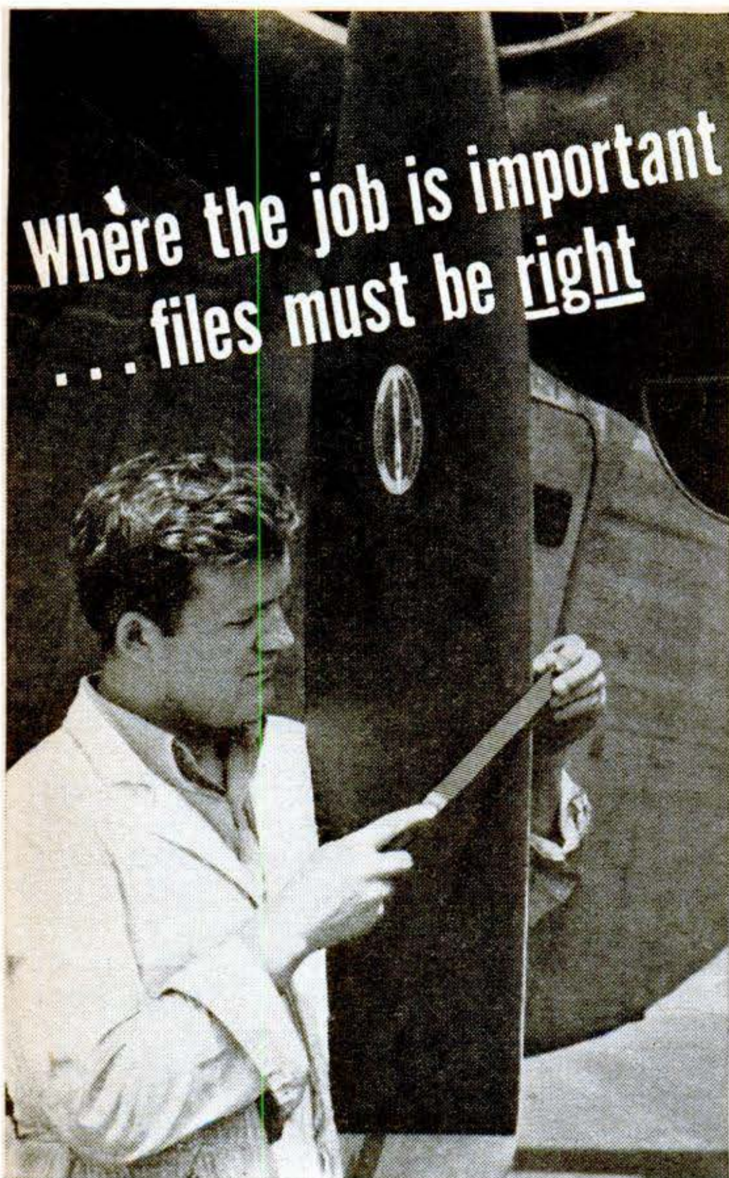
Filing nicks out of propeller blade of Budd-built RB-1 transport plane.
