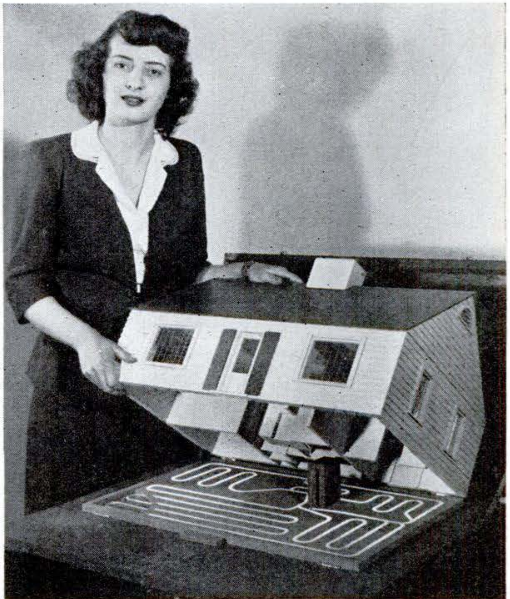
Panel or radiant heating of a home is done through a system of heat-conveying pipes under the floor, as shown by this demonstration model. Heat is uniform in all parts of a room
