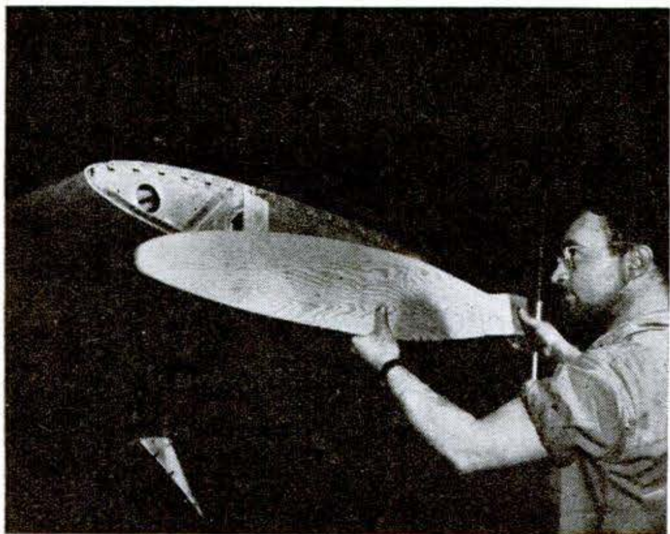
5 After wing tips are removed, openings are covered with plywood. Other openings left by removal of protruding parts are similarly protected
