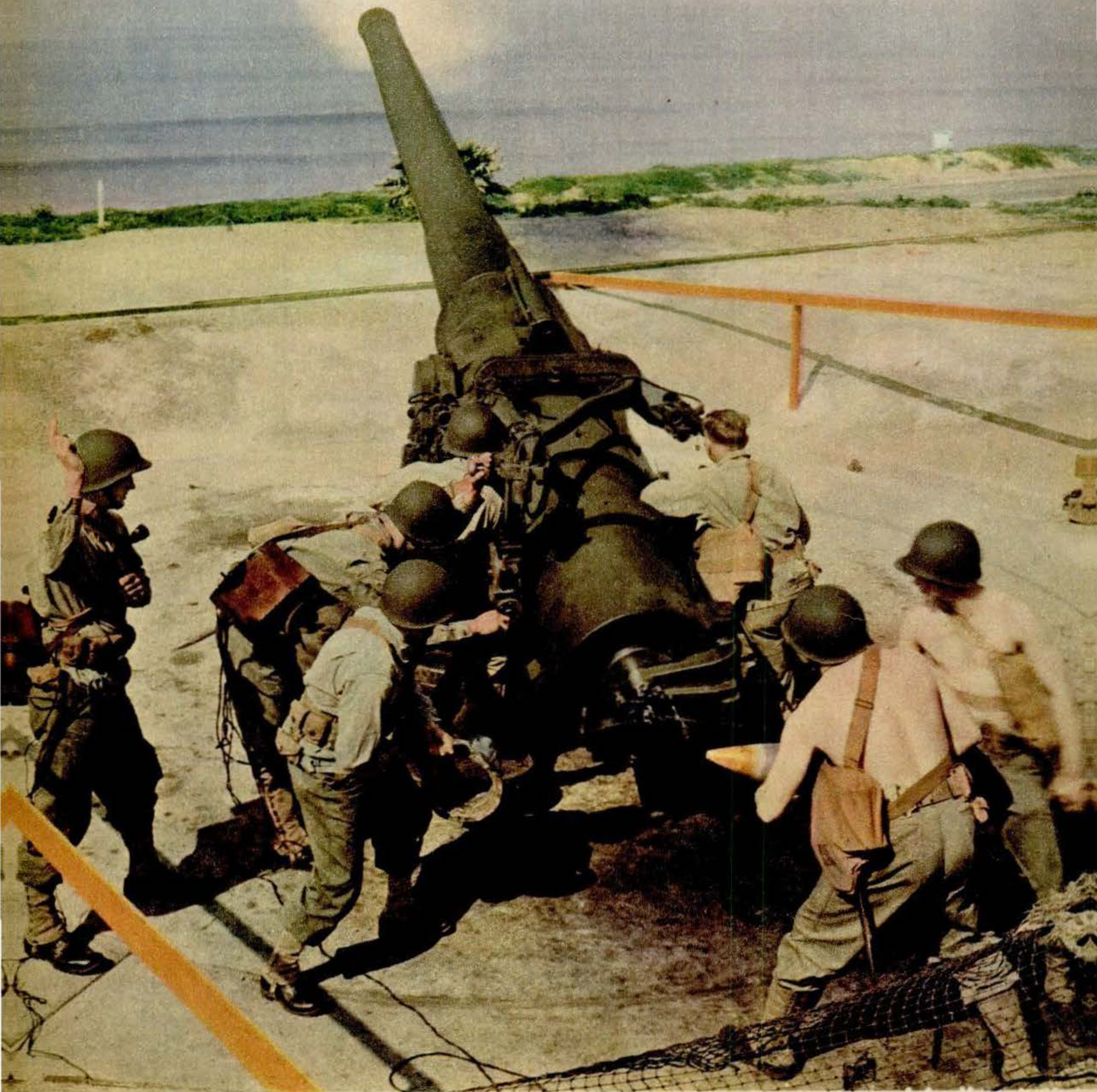
A six-inch harbor-defense rifle sends a 105-pound projectile hurtling nearly 13 miles out to sea from its pedestal mount. Firing either high-explosive or armor-piercing shells, such guns not only protect our own shores but also guard the foreign bases for our offensive drives
