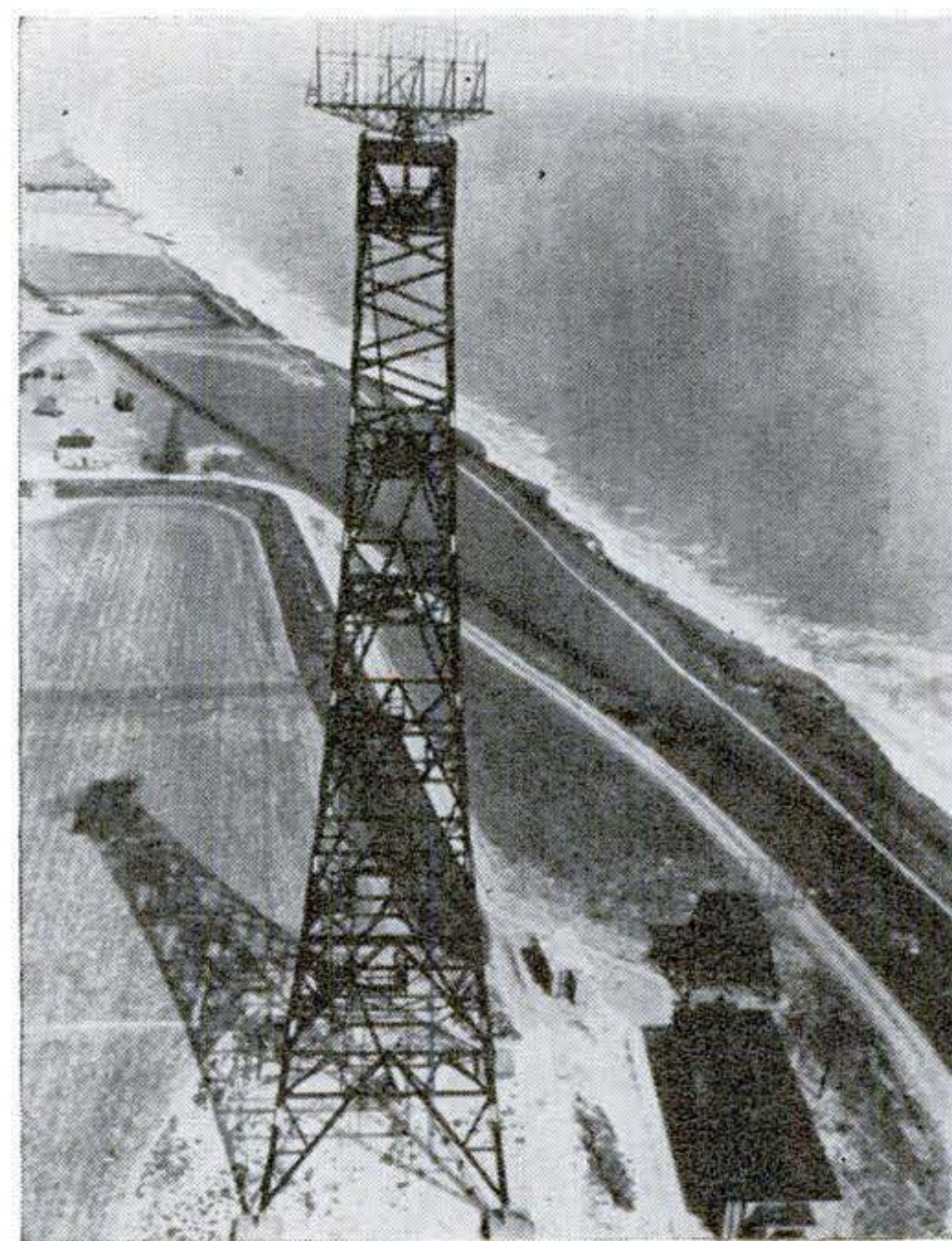
England had complete radar coverage along her channel coast in 1938 with 15 of these 360-foot towers.
