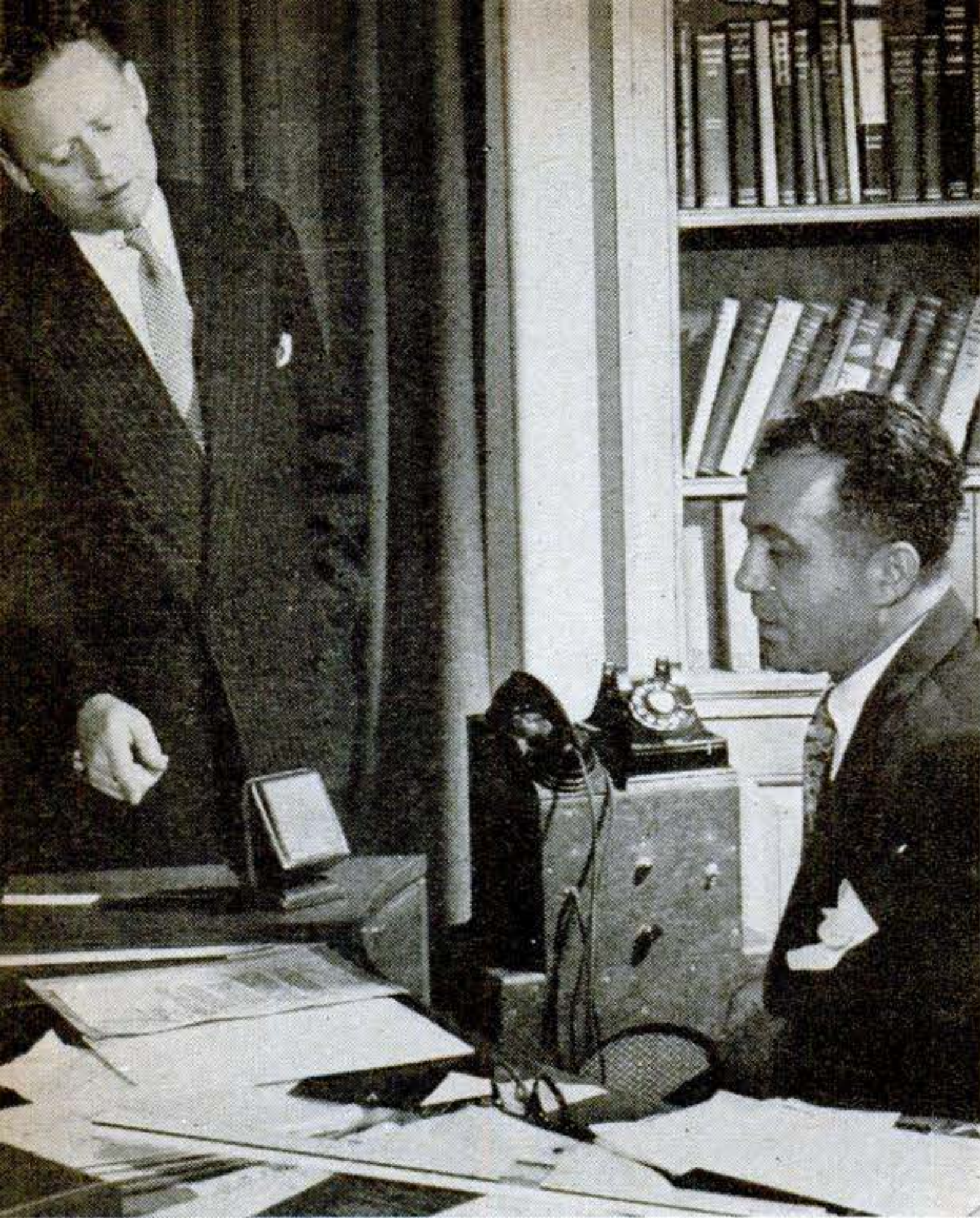
Assen Jordanoff (seated) listens to an associate in his office while a third party may join in the conversation through Jordanoff's Jerryphone. The microphone on the desk feeds to the telephone mouthpiece; incoming voice comes via the loudspeaker.
