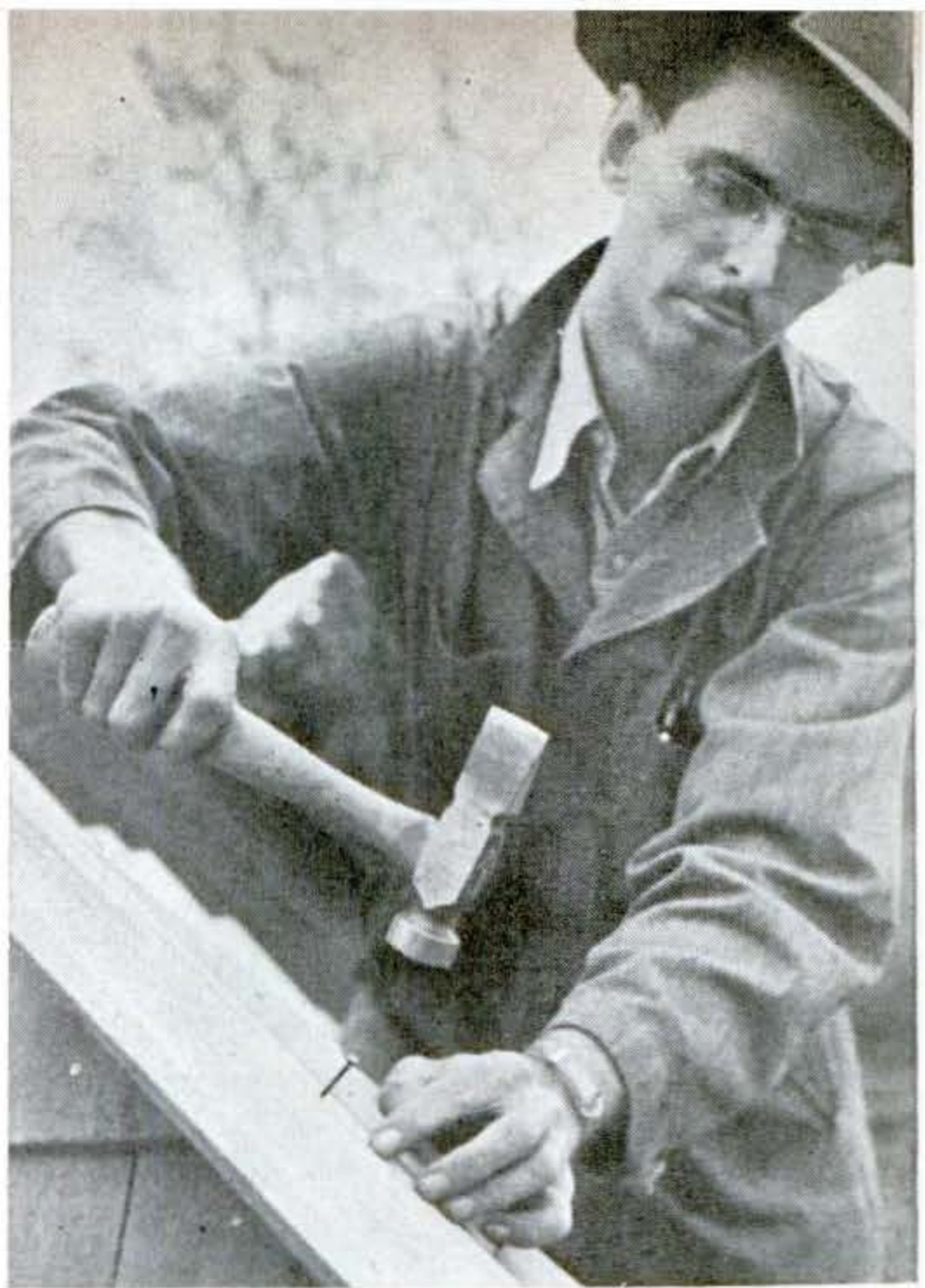
Using the machined shingling hammer. The hatchet edge splits bad shingles to make removal easier.
