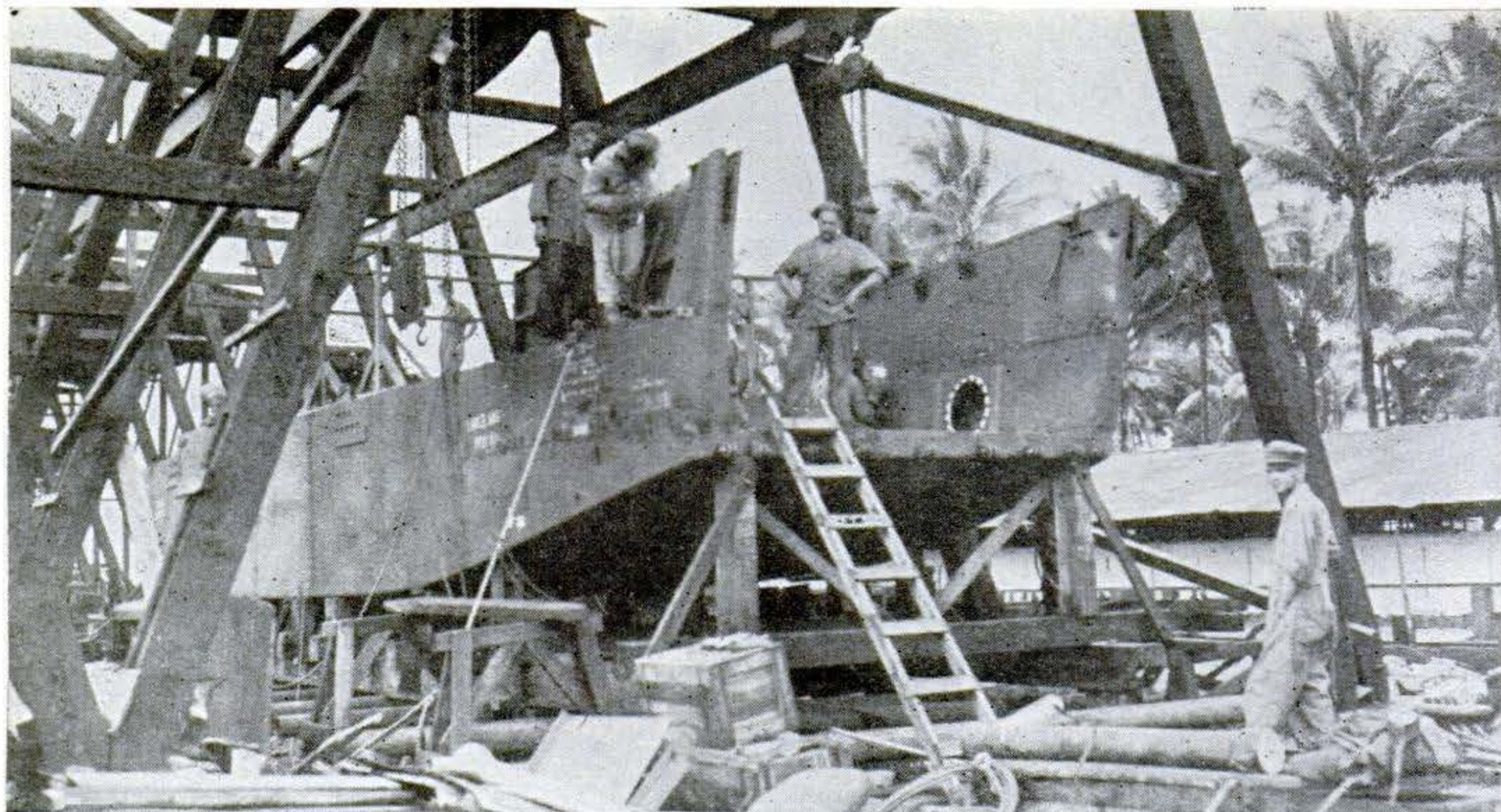
At Milne Bay, New Guinea, Army engineers weld together sections of a landing craft shipped knocked down to conserve space. Such craft as this are used to invade Jap-held islands. The strange vehicle shown below was welded together from locomotive and truck parts and served as a switch engine in North Africa.
