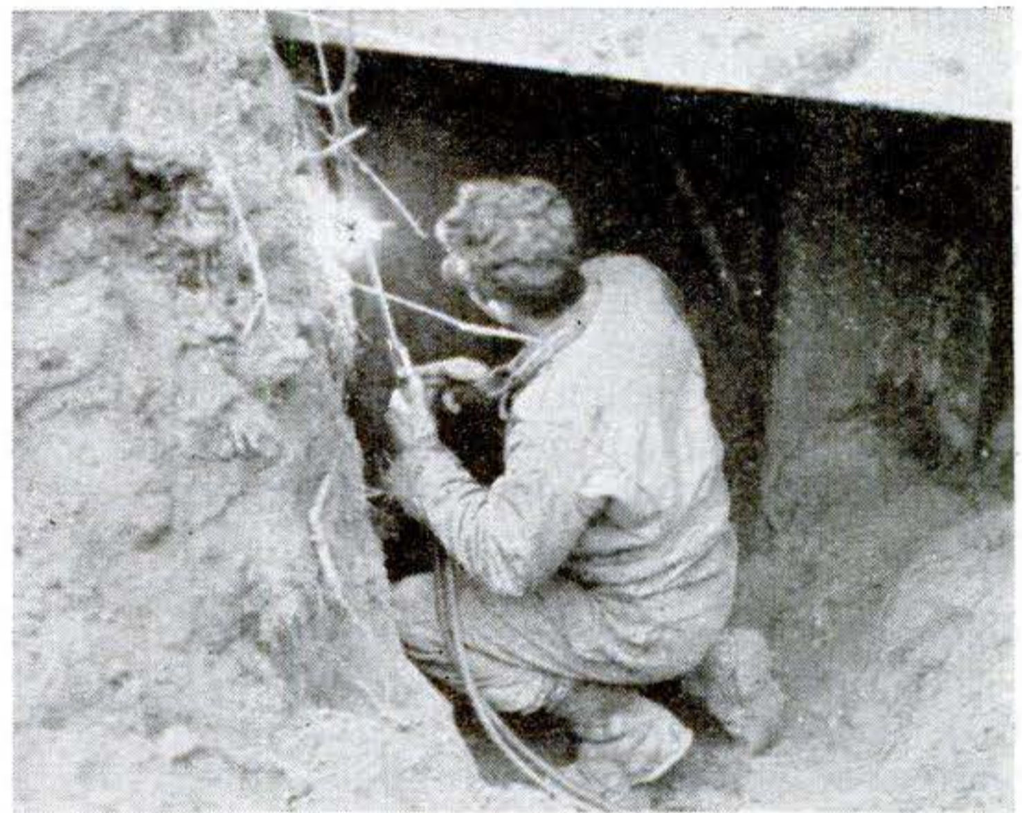
This remarkable photo by T/5 George W. Herold, of the Army Signal Corps, shows a fighting engineer cutting away the door of a Siegfried Line pillbox.
