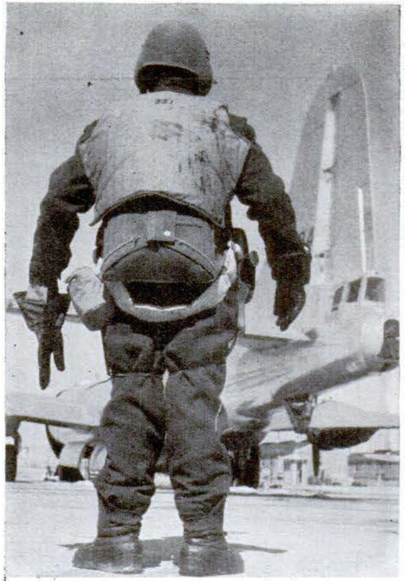
This combat dress (front and rear views) of a B-29 crewman would be far more bulky if it were not scientifically designed. The inner layer is electrically warmed with the correct amount of heat going to each part.
