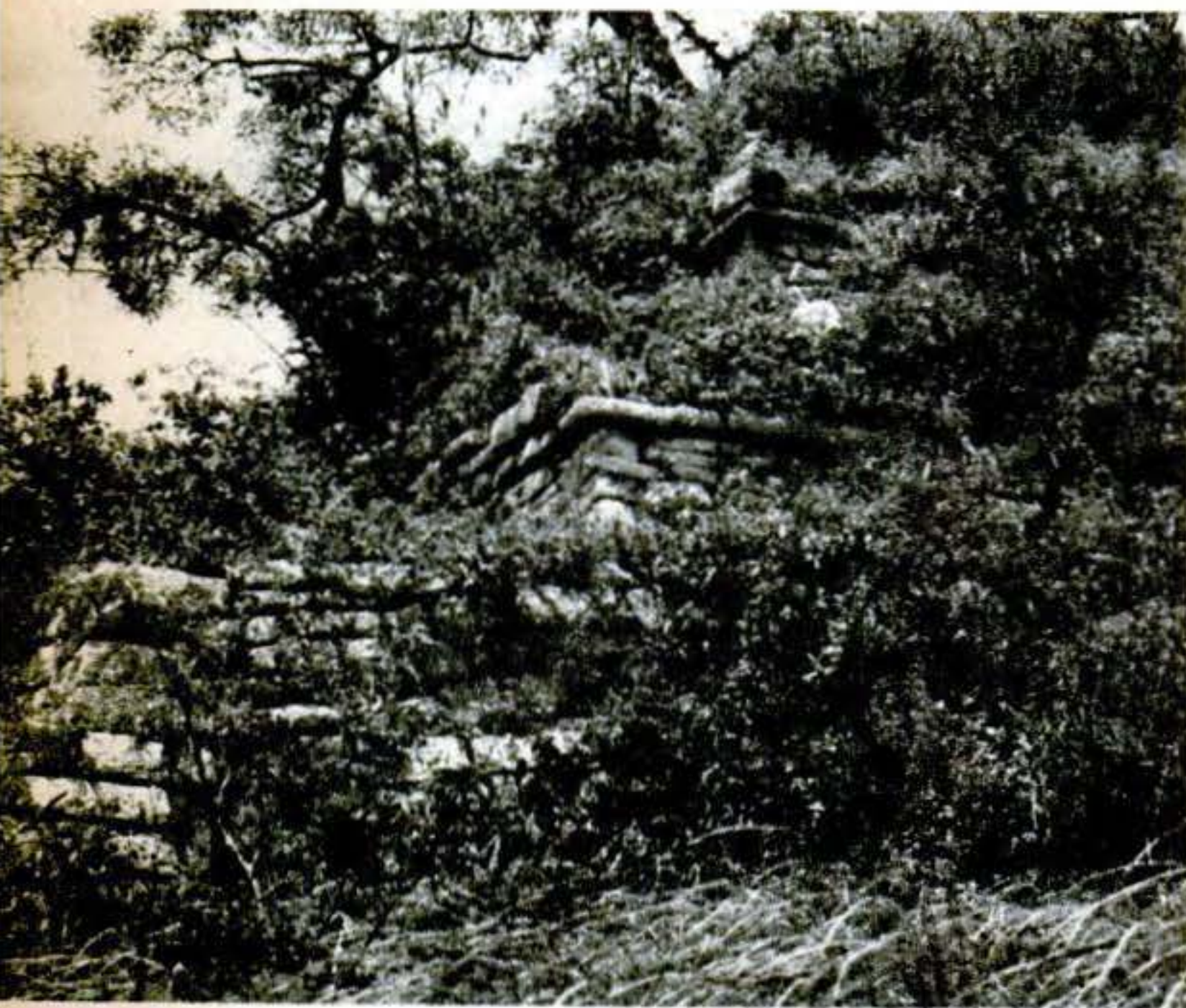
The southwest corner of the upper pyramid at Agua Azul as it is today after about 15 centuries. There is evidence that stones were joined with hard cement.
