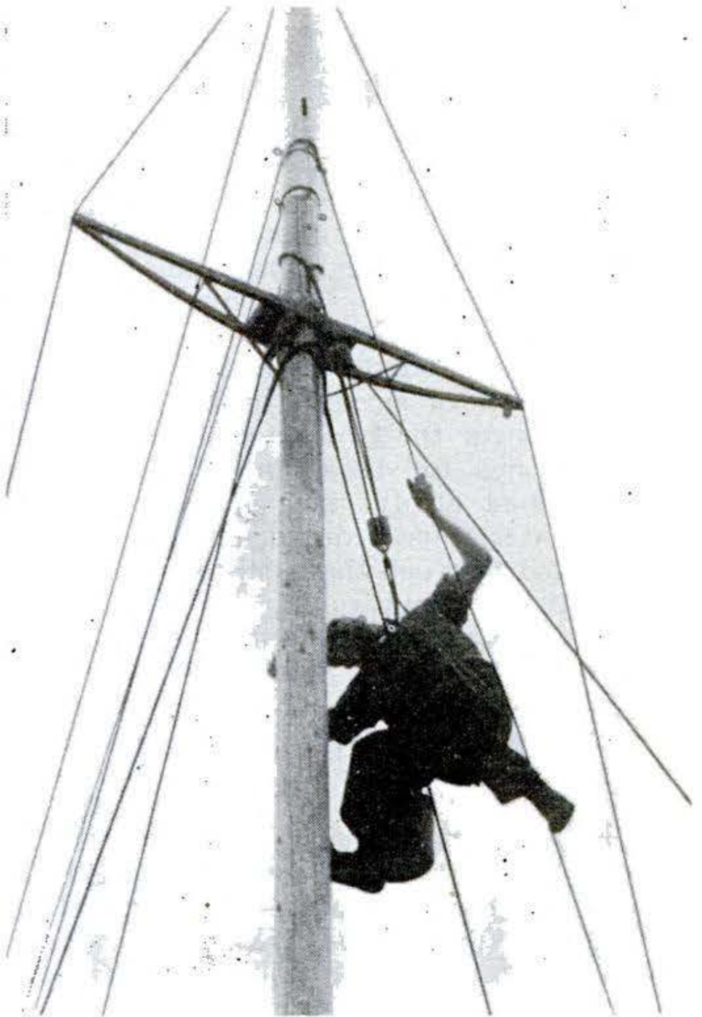
Aloft in a bosun's chair belayed to the deck, the seaman here employs one hand in work on the mast while keeping the other on a shroud for safety.
