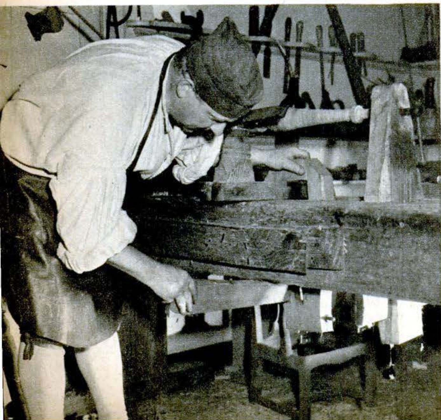
THE OLD-TIME LATHE , used for turning, grinding, polishing, etc., was made of heavy timbers and other pieces, and was a difficult device to adjust. The tool rest, a strip of iron fastened to sturdy wooden pieces, could be moved only by loosening a wooden wedge, then sliding the assembly into the desired position and tightening the wedge again. Above, the cabinetmaker adjusts the piece on which the tool rest is fixed. Below, he inserts the wedge to secure the piece.
