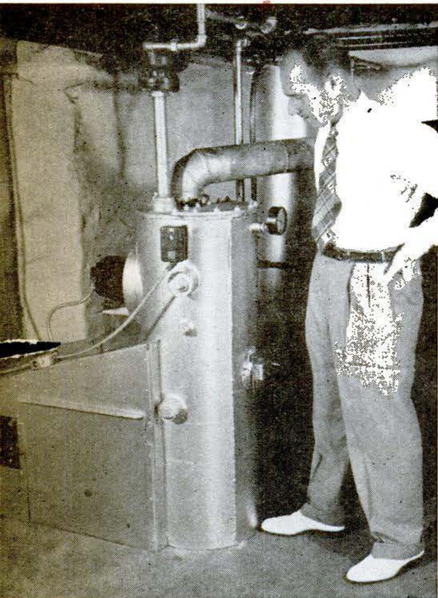
This midget furnace burns hard coal in a fire chamber only 8" in diameter. It was developed from the Anthratube, a pipelike, experimental heater announced two years ago. Fuel is fed by an Archimedes screw.
