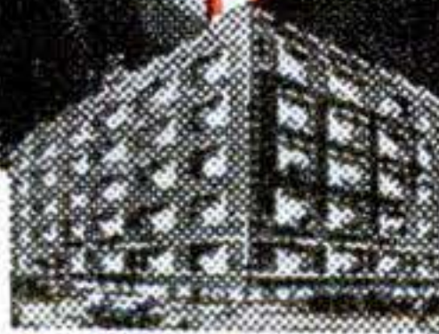
This big fire-proof building is occupied entirely by the Coyne Electrical School.
