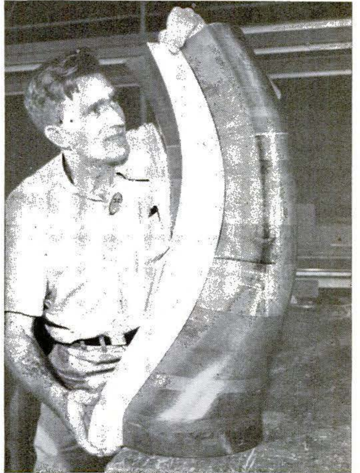
Gladwell checks a mahogany model of large air duct with metal template to insure accuracy. Mahogany holds its shape well, with little shrinkage, and is easier to work than pine despite its toughness.
