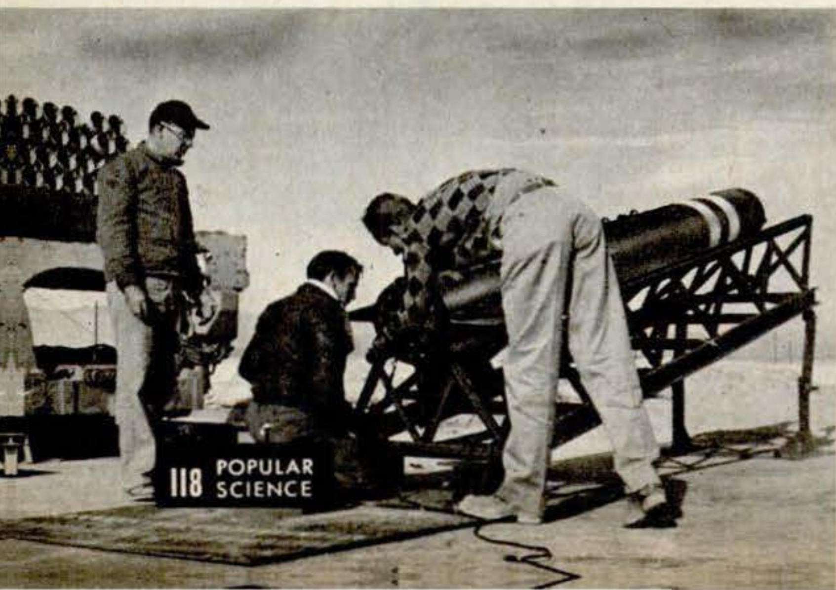
Biggest U. S. artillery rocket built for aircraft launching is Big Dick, shown below in a ground test. It is 14 inches in diameter, 150 inches long.
