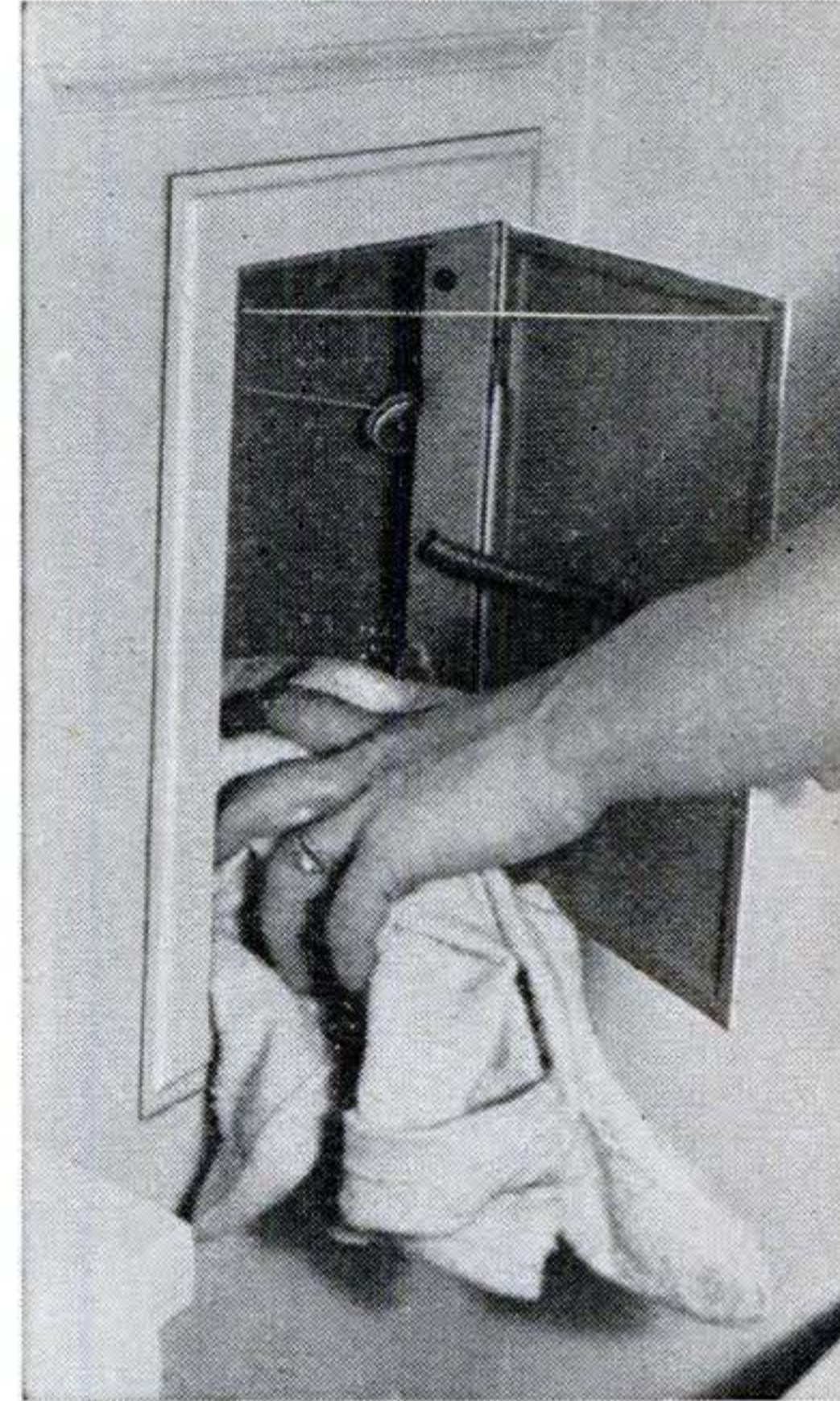
Kept open, the door holds the trough up; closed, it drops the trough down.
