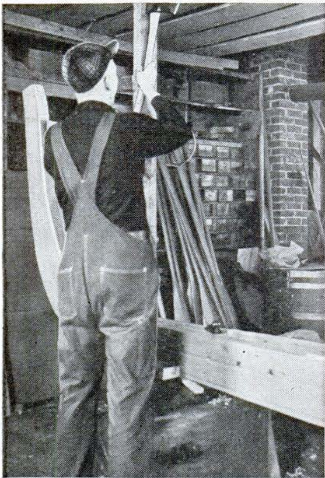
At left, a two-by-four is forced in between the topside of the keel and the overhead beam. After it is checked with a spirit level, it is toenailed in place. More diagonals are fitted in as above. The best system is to alternate from one side to the other to avoid one-sided pressure.
