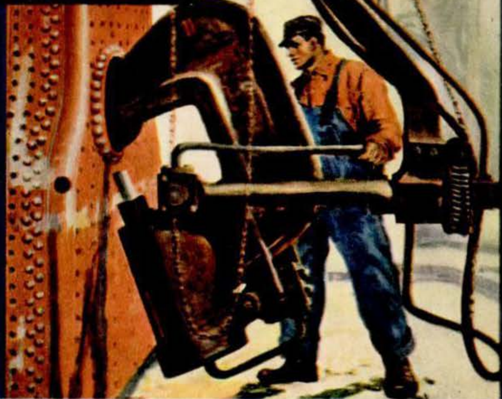
This tremendous rivet squeezer was a good idea when it was shown on the cover for June 1920. In February 1947, PSM showed a hydraulic riveter that puts a 50-ton squeeze on railroad cars.
