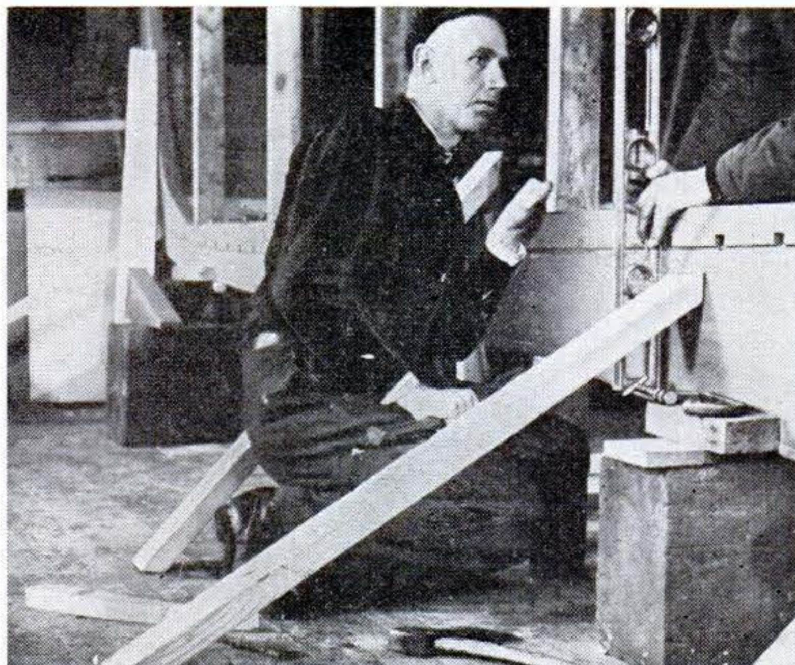
At left, a two-by-four is forced in between the topside of the keel and the overhead beam. After it is checked with a spirit level, it is toenailed in place. More diagonals are fitted in as above. The best system is to alternate from one side to the other to avoid one-sided pressure.
