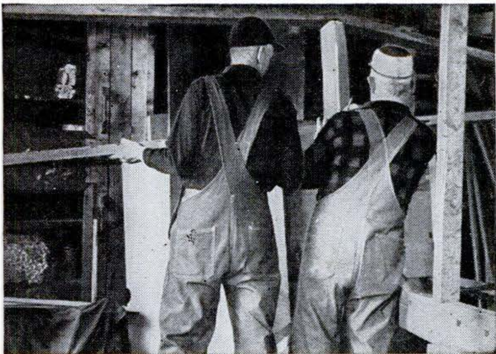
Time and pressure true up a warped stem. Two two-by-fours are braced against it, one above the other, pressing in opposite directions.
