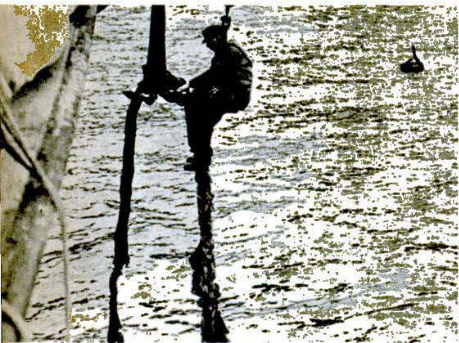
7. A damaged cable, crushed by an iceberg, is lifted up by grapnel off St. Johns, Newfoundland. Man over the side is putting on a "stopper" to permit one end of smashed cable to be brought into ship for repairs.
