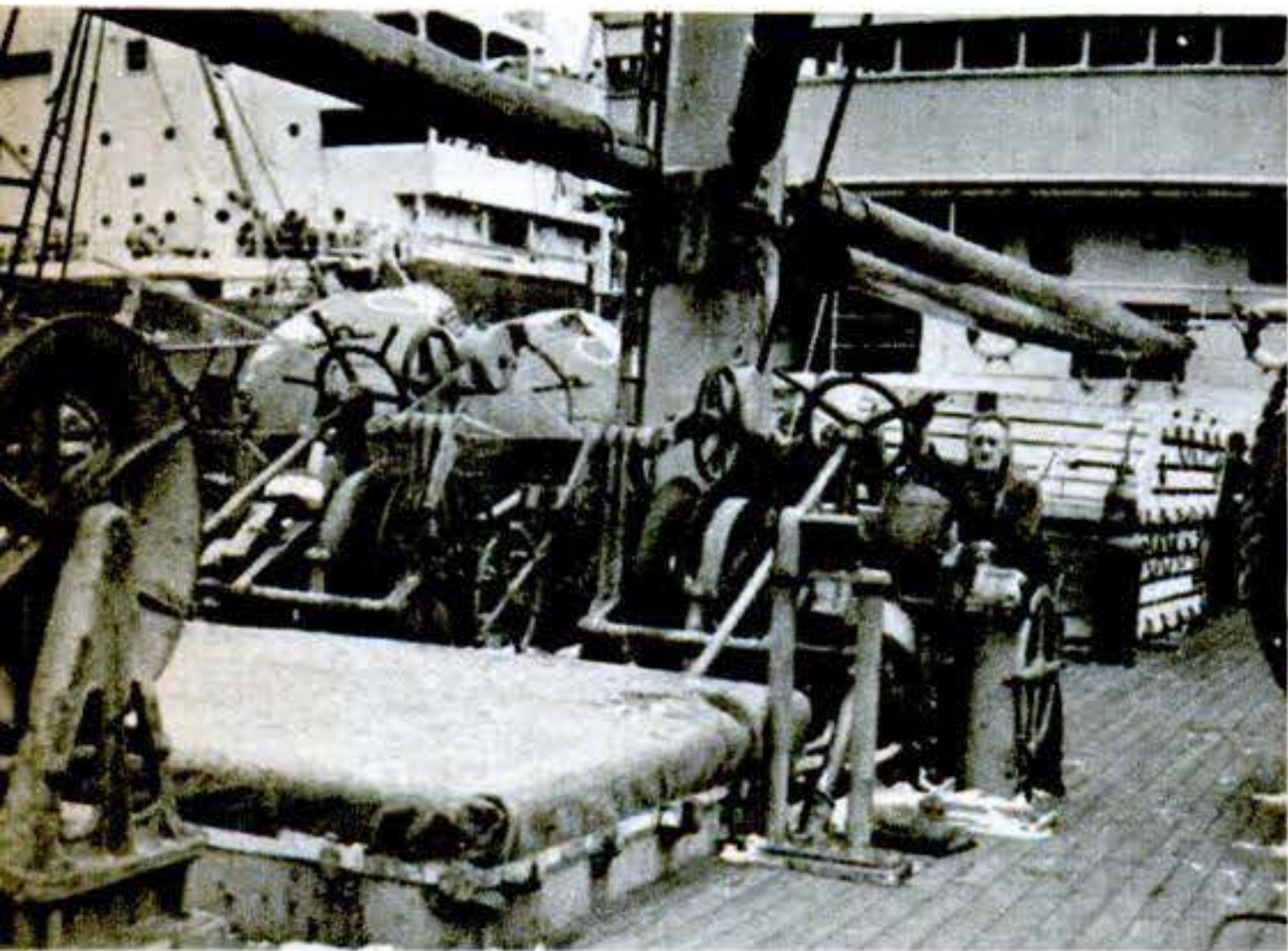
3. On the ship's foredeck is the machinery that picks up and pays out cable as desired. Accuracy in controlling speeds under all sea conditions requires the steam-operated machines to be manned by experts.
