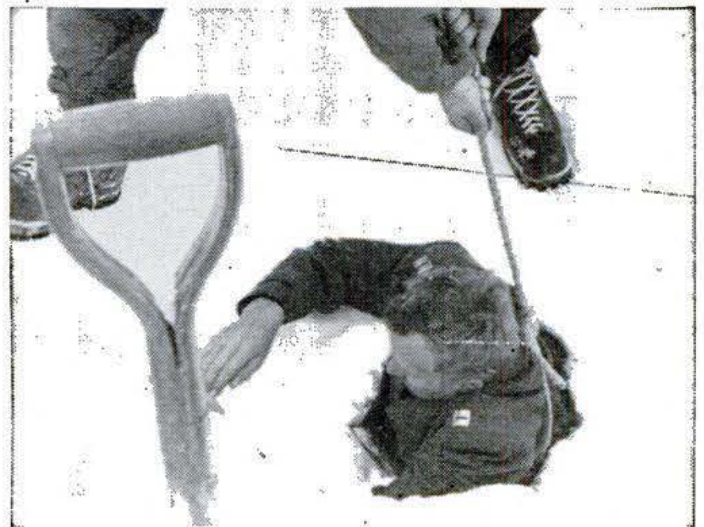
These men have dug out the skylight of Byrd's old snow melter and are lowering in Captain Vernon Boyd. Polar snows bury a house in a few days, so roofs must bear a load of 50 lb. per sq. ft.
