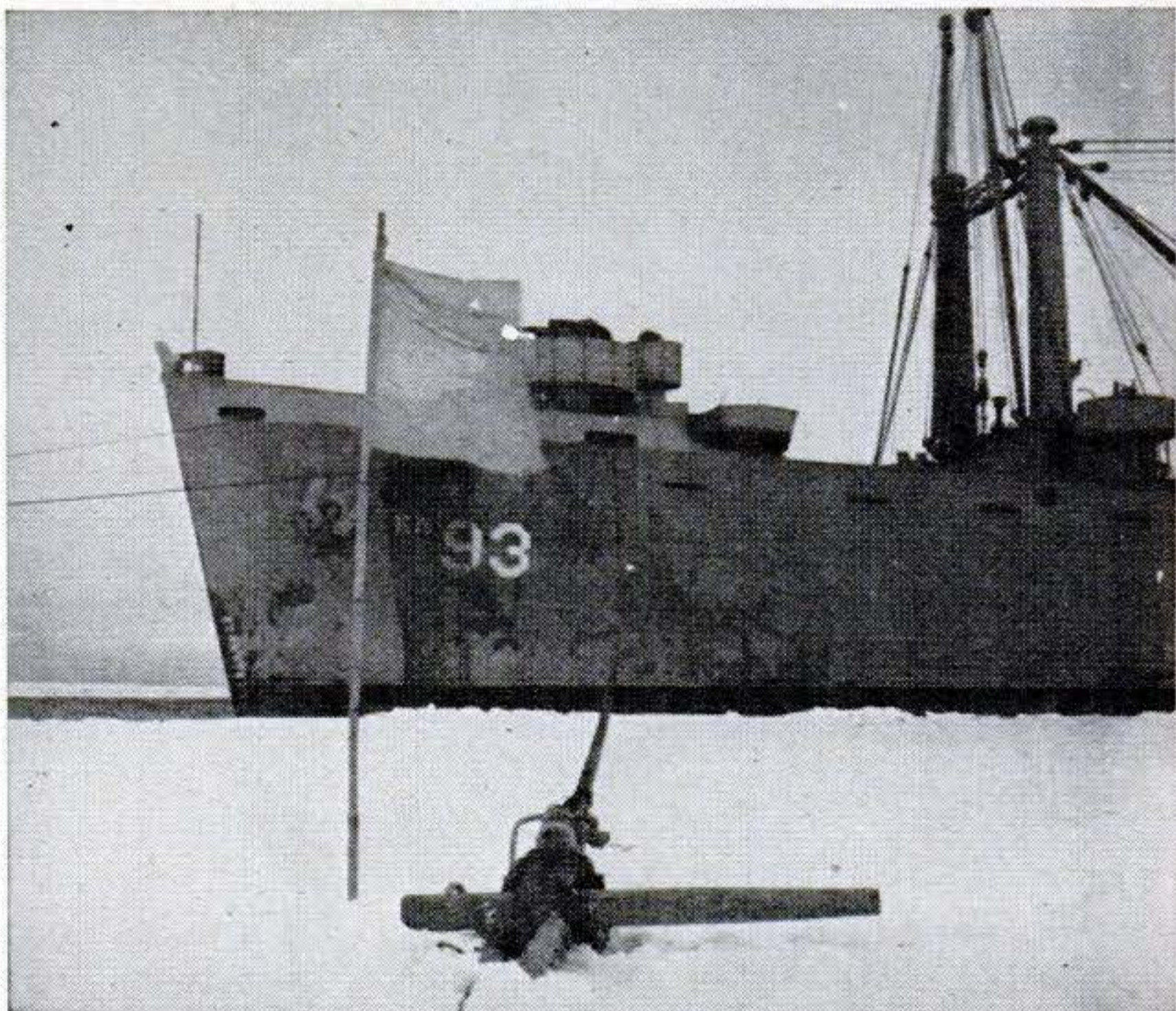
This ship is moored to the ice by a "dead man"—an eight- by eight-inch timber placed in a hole chopped in the ice and secured by pouring in sea water, which freezes immediately.
