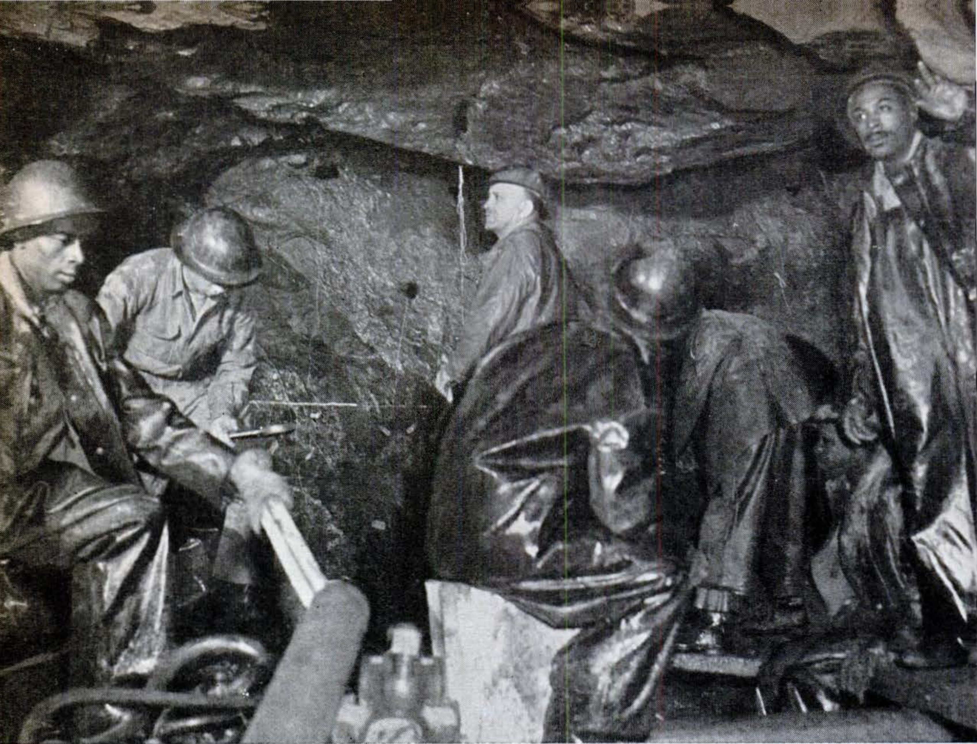
Drill holes are loaded and men atop the Jumbo check electric wires that will fire the blast.
