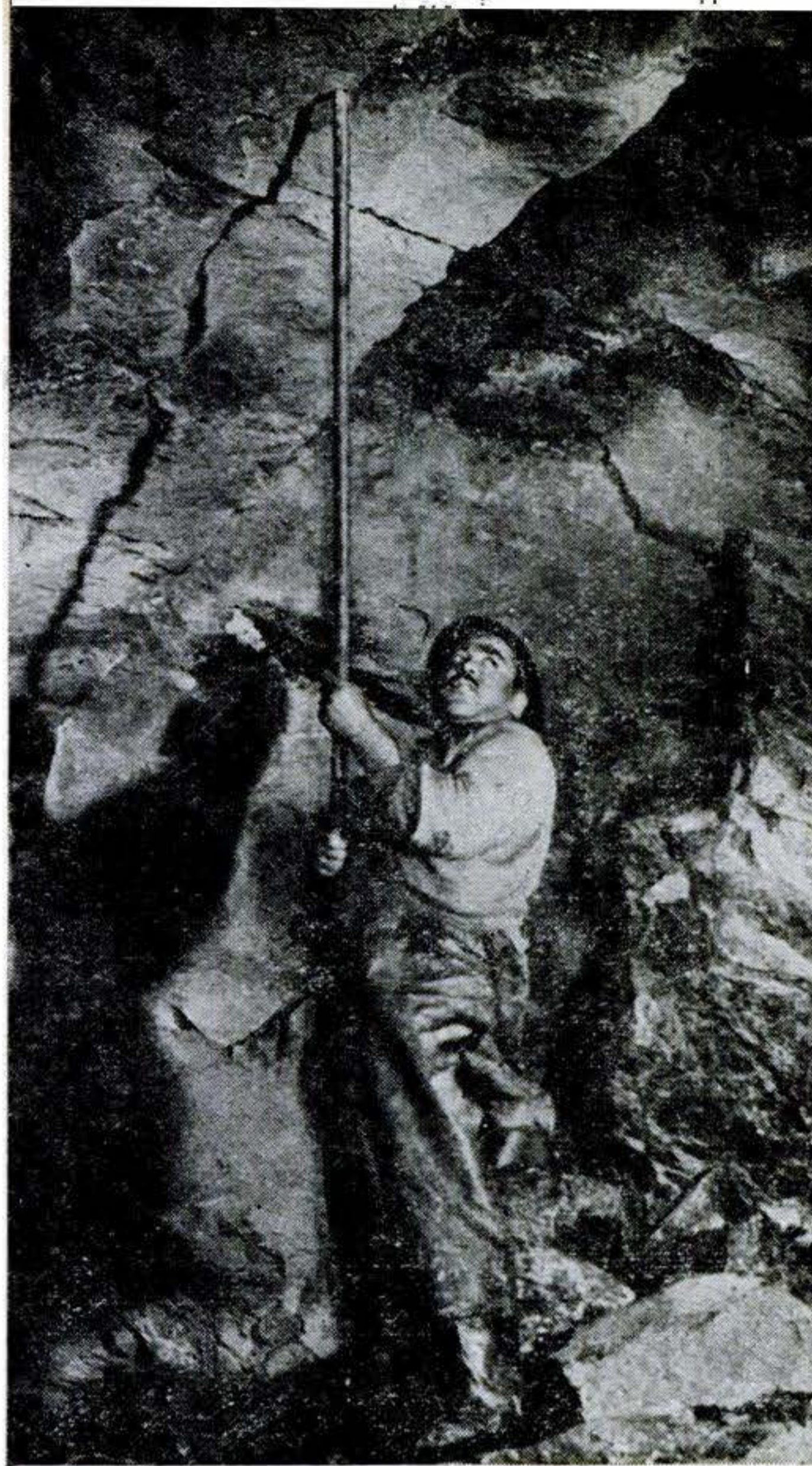
Scaler pries down loose rocks after a blast. His job looks deceptively unexciting, but tunnel men consider it the riskiest of all.
