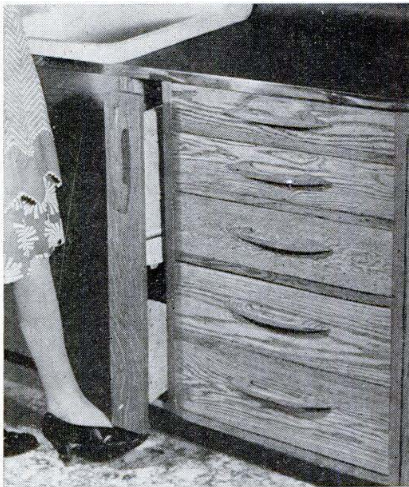
Toe operation saves time when the hands are full. The rubber guard prevents scratches on your shoe.
