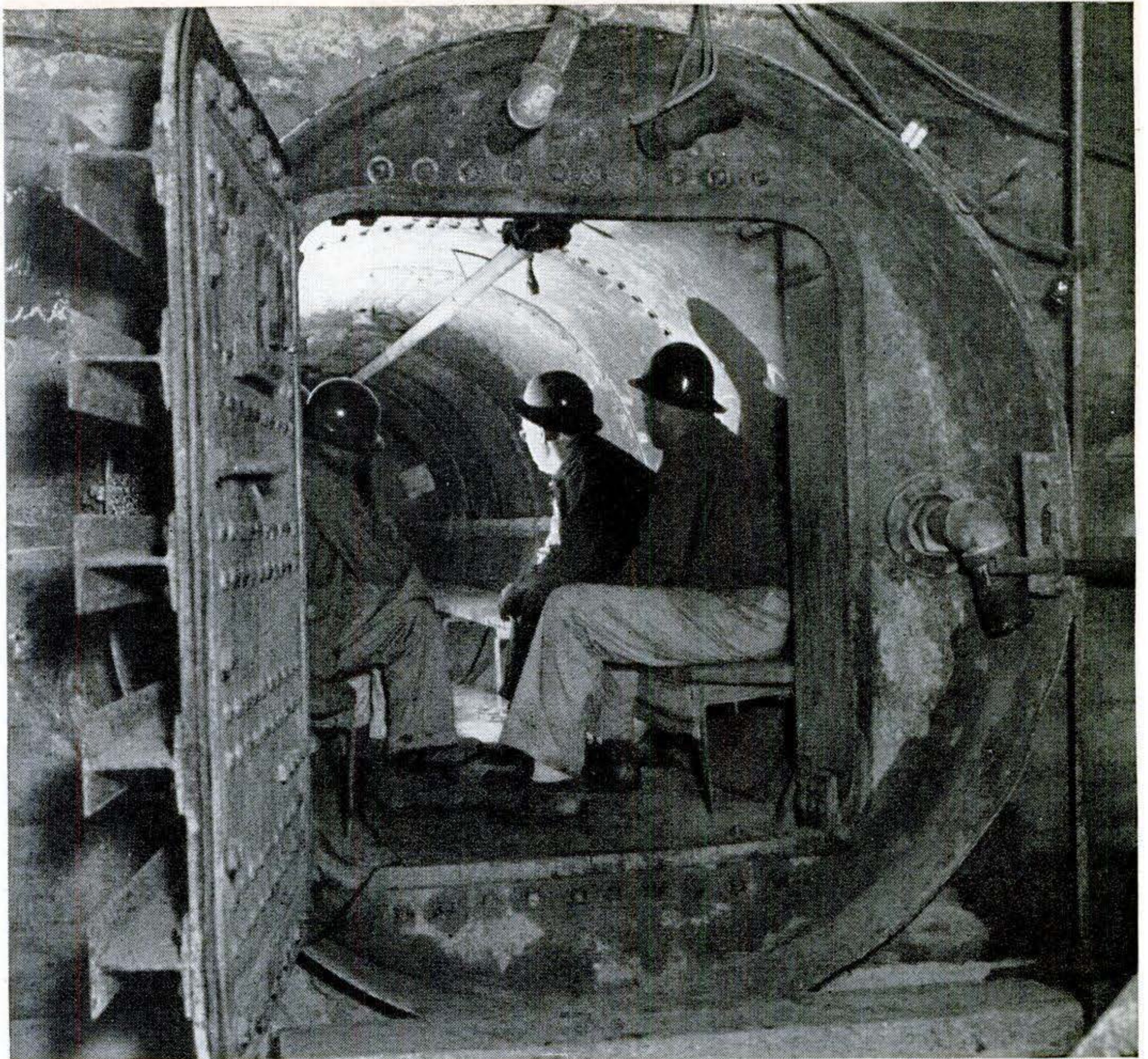
Man lock in concrete bulkhead admitted sandhogs to section of tunnel under compressed air.
