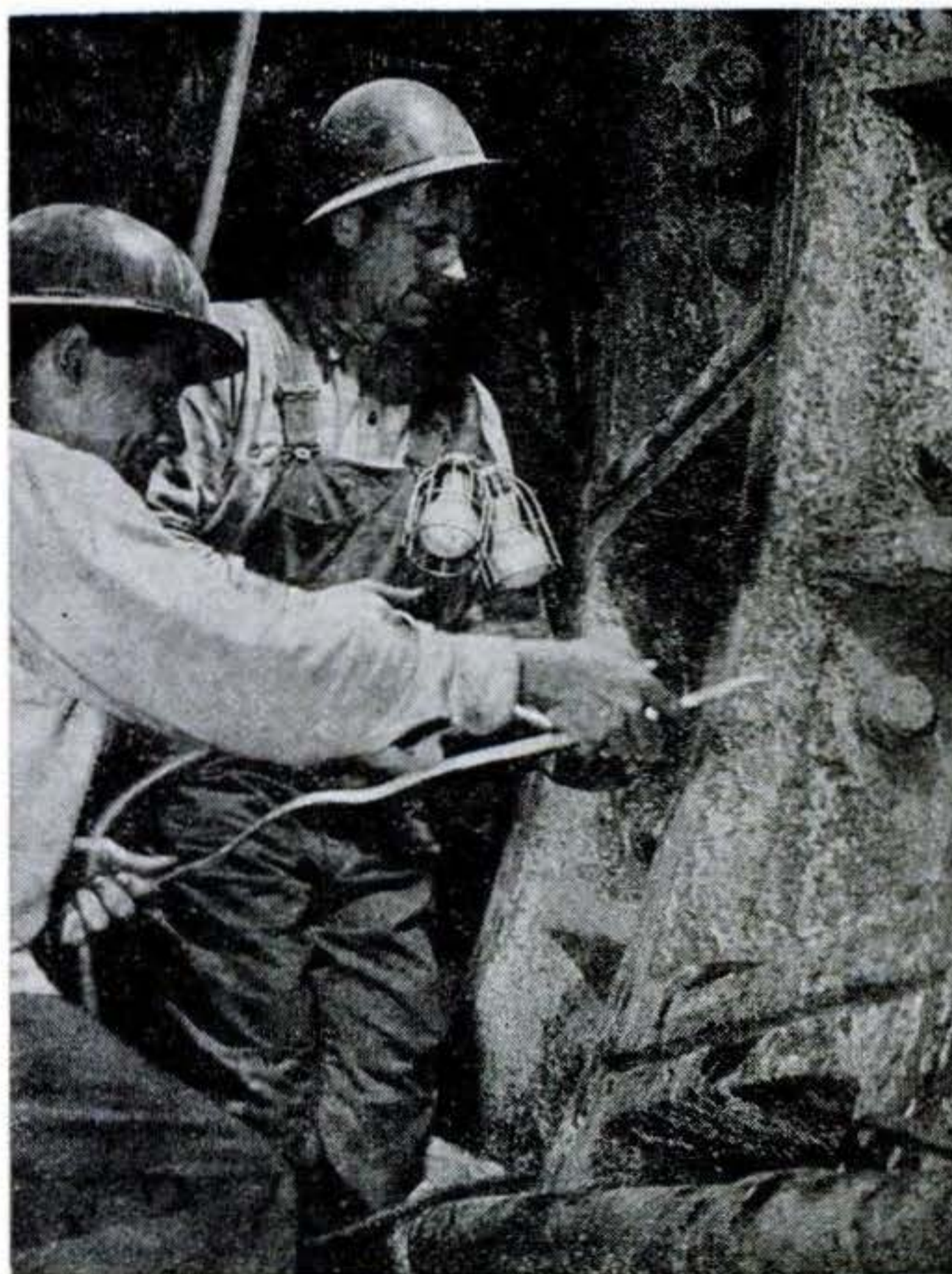
Sealing ring joints with waterproof calking of solid lead marks end of victorious battle to keep out the tons of water overhead.
