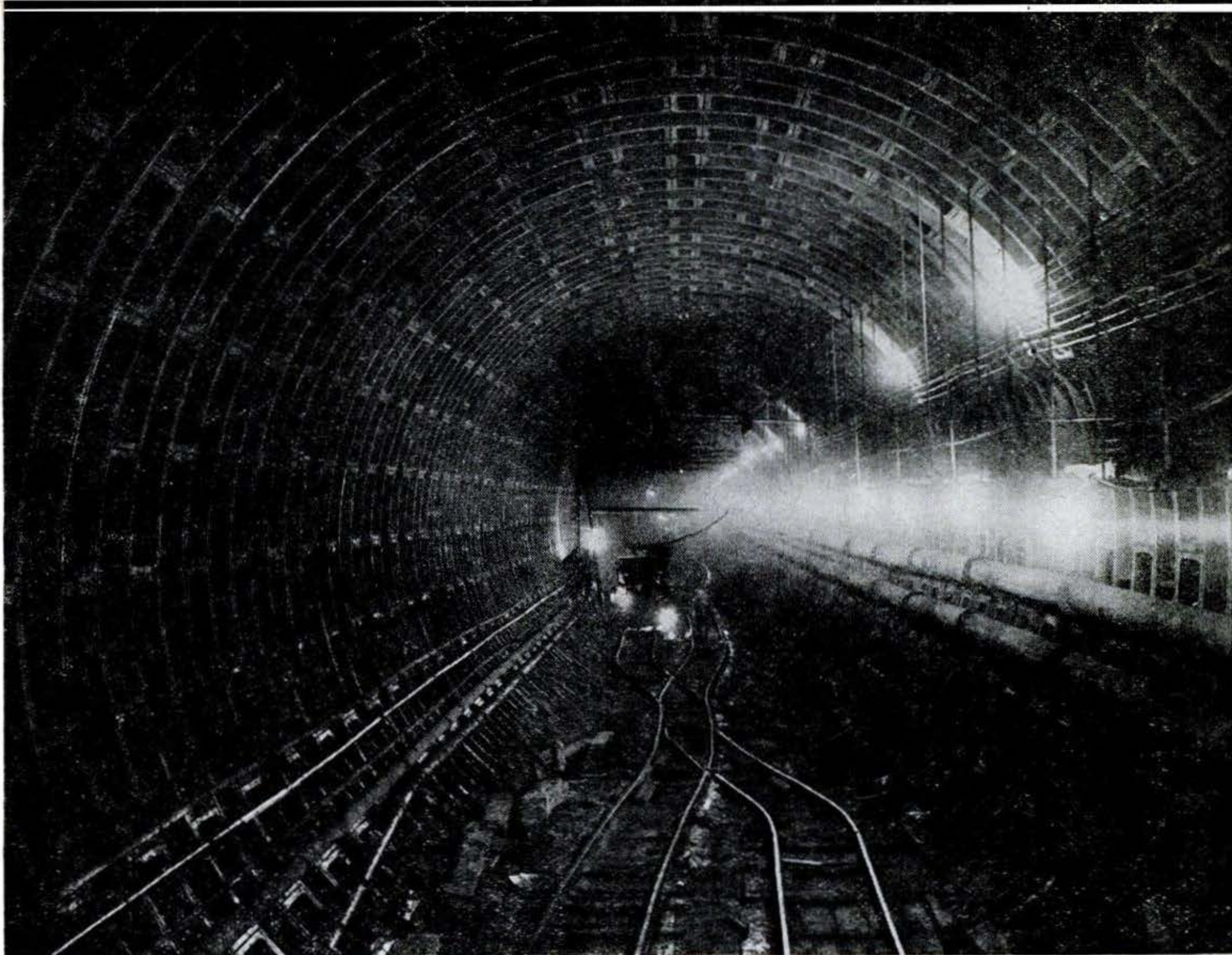
Iron rings consolidate sandhogs' possession of the shaft they wrested from the river bed.
