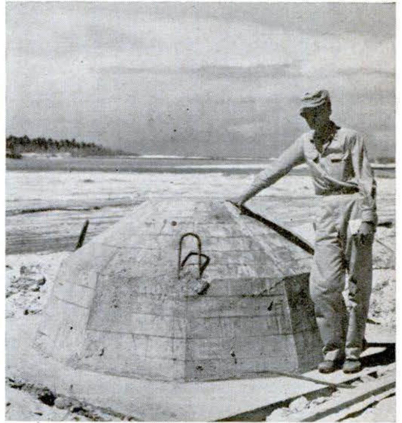
Concrete "igloo," near detonation point, contained instruments to record data during blast.
