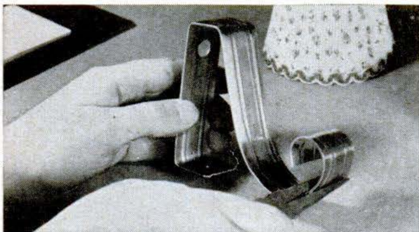
Bracket for wall lamp is bent of 1¼" flat decorative strip. Socket is attached through a ⅜" hole at the top of the straight section.
