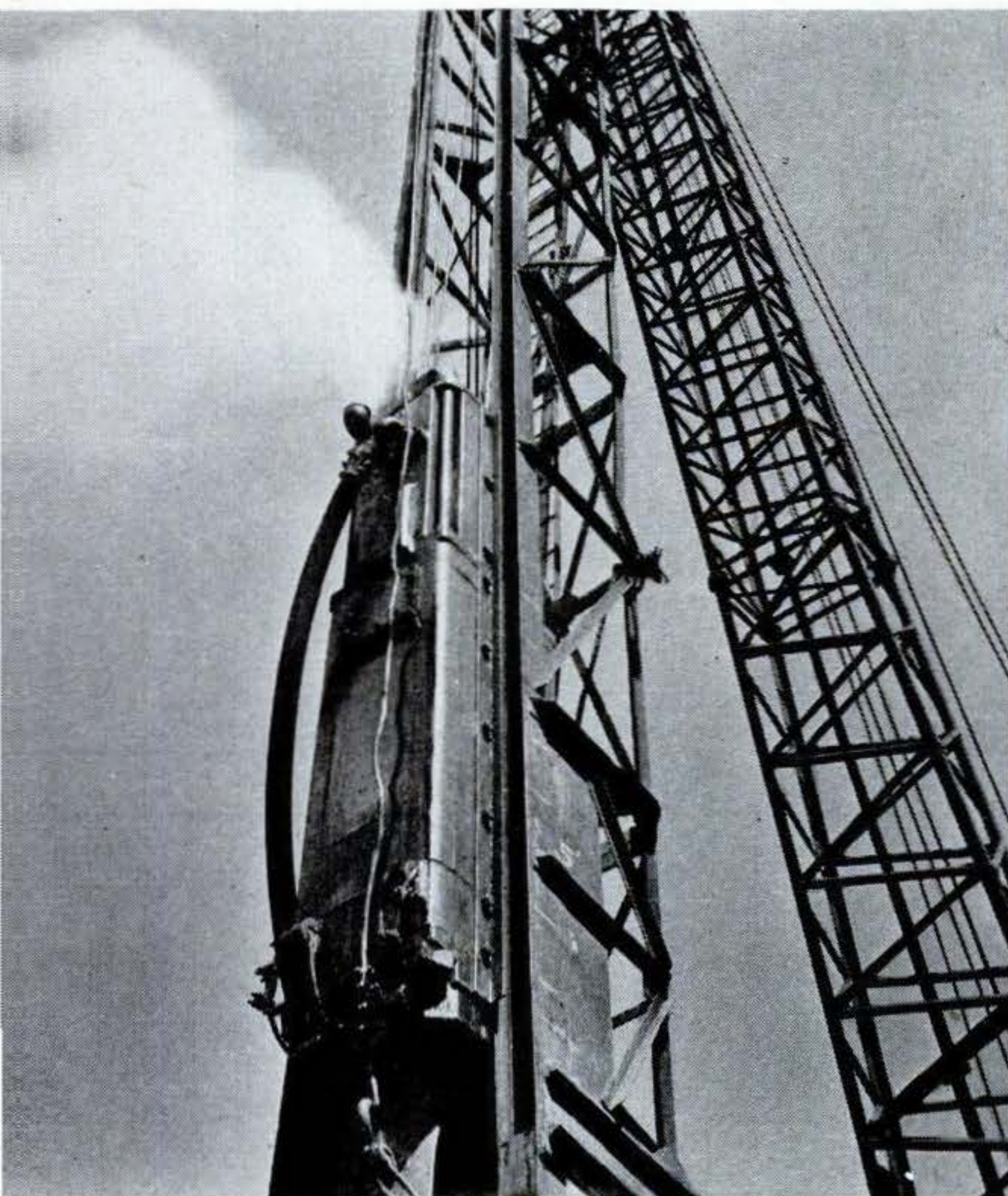
5. Fifty-five clanging blows a minute from four-ton ram of steam-spouting hammer drive pile home. Rapid at first, progress gradually slows, ending when pile reaches bedrock.
