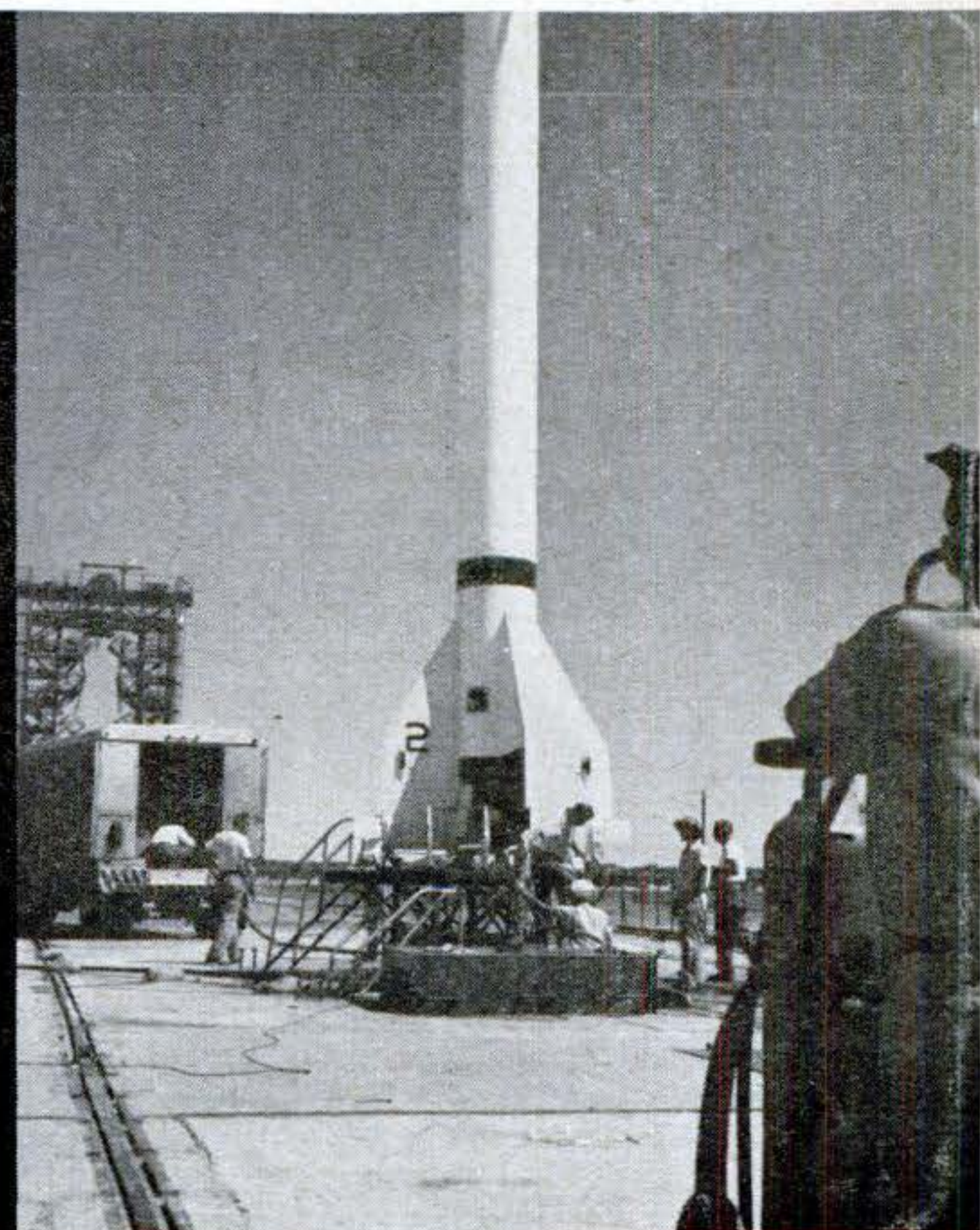
6 Gantry is rolled away as rocket is readied for firing. One of the last jobs is being done by the refrigerator truck at left, which is pumping in 3,700 pounds of liquid oxygen. ➤
