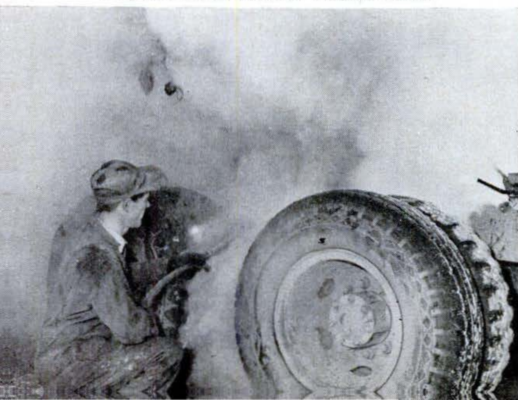
7 Using steam, driver cleans frozen mud and ice from trailer. Rolling through two winters, the trucks covered 400,000 miles.
