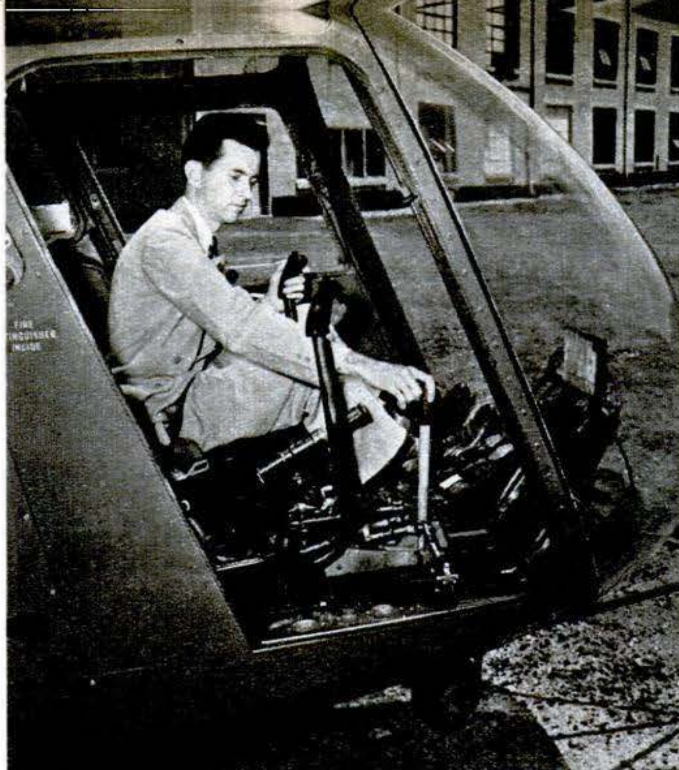
Inventor shows additional control for balancing 'copter fore and aft. Lever works vestigial tail-plane. Behind right-hand stick is pitch-control lever and throttle. Craft's ceiling is 14,000 ft.
