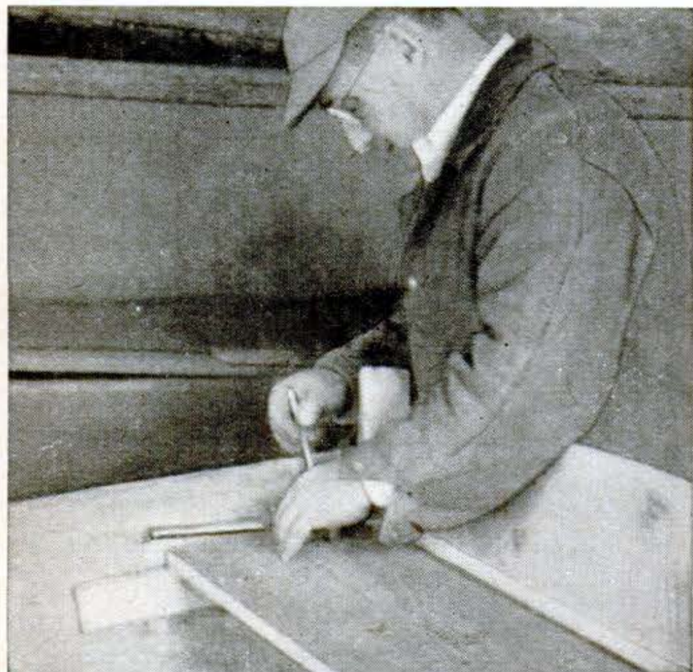
New stern seat of two planks is being installed. Notch two corners of the aft plank to fit around the two supports at the stern.
