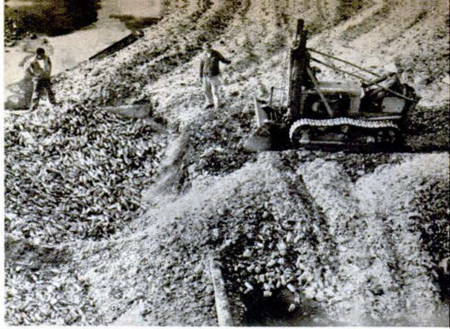
From mountain of discarded glass, bulldozer starts material on its way to becoming cullet by shoving it into pair of 500-ton-capacity concrete hoppers that feed the crushing plant.
