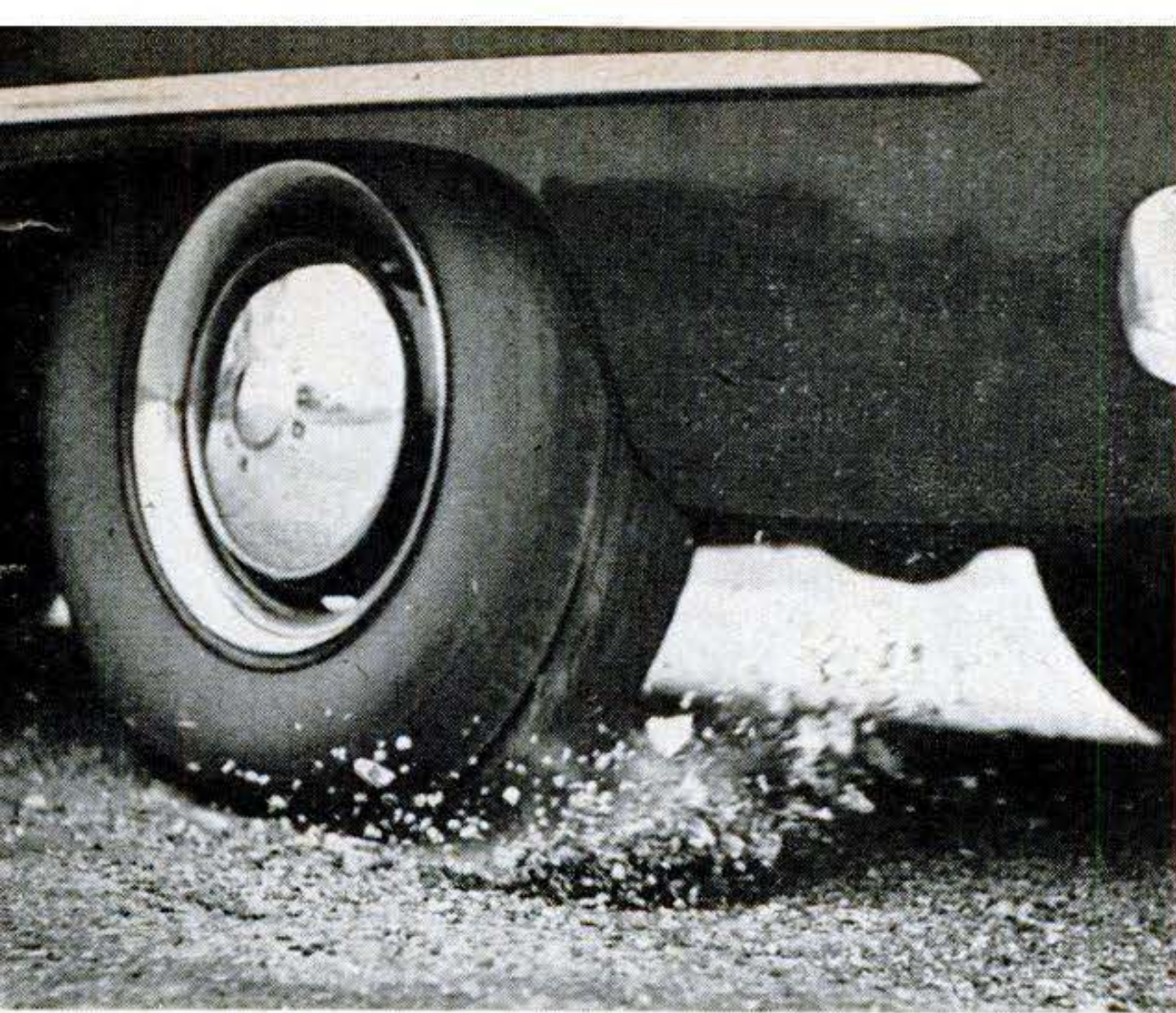
Faulty asphalt mixture may shed stones as above, leaving potholes, or acquire "washboard" surface by yielding under pressure.
