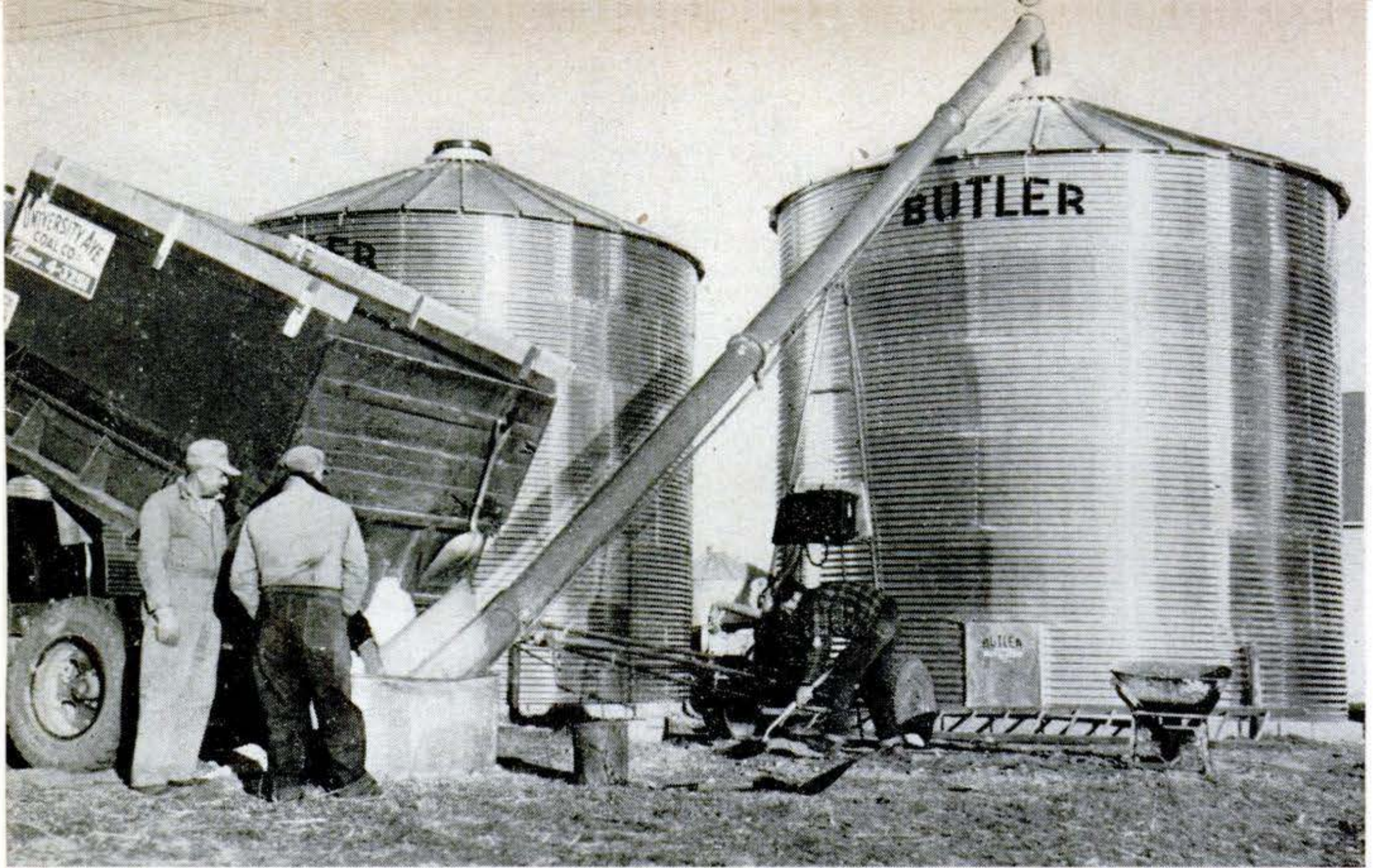
With these quickly erected aluminum tanks, surplus grain was saved from weather damage.
