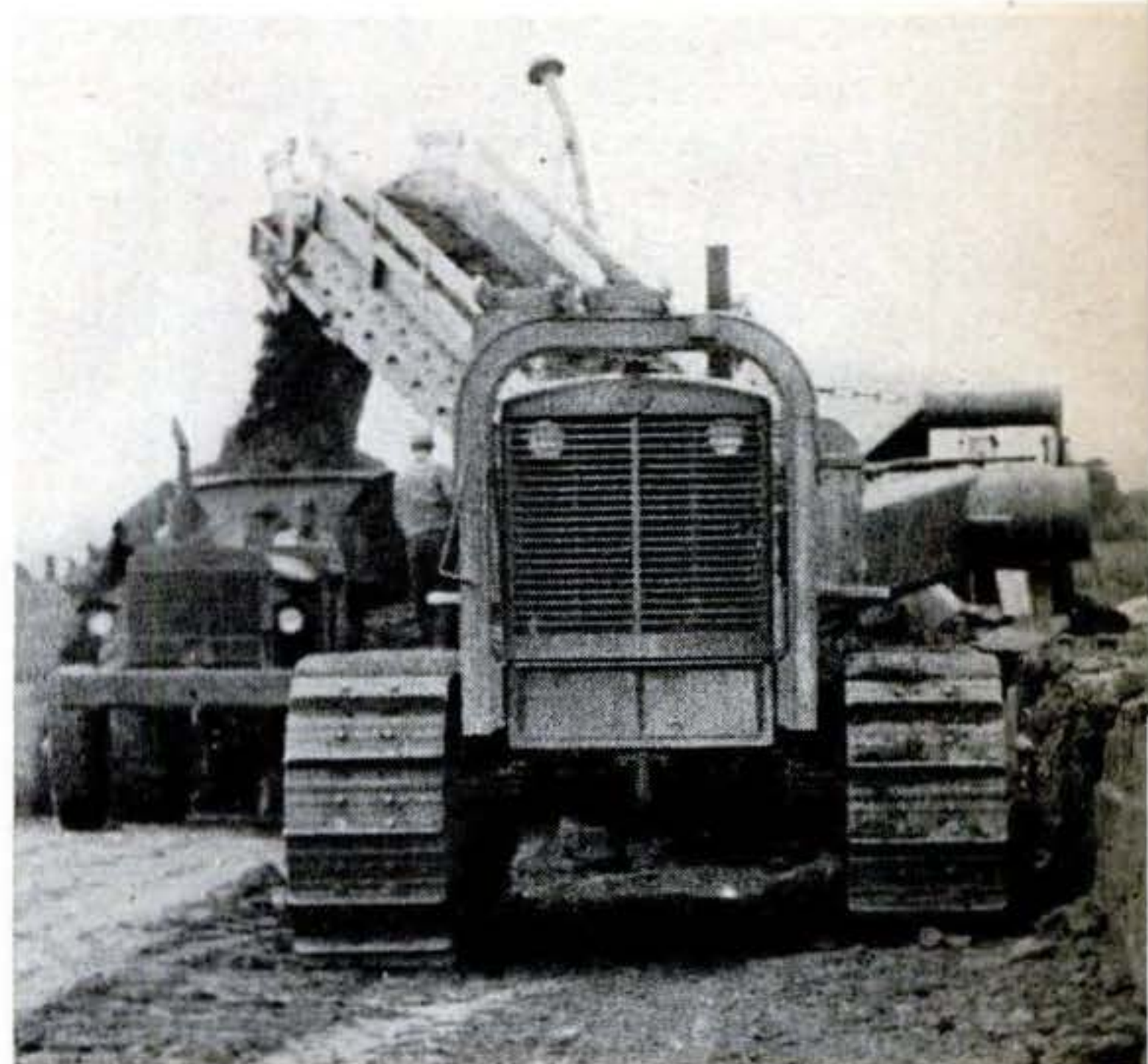
Above, tractor pulls loader along at brisk 3-m.p.h. pace when cutting. Note the depth of the cut as shown by the high bank at the right. Below, a General Motors Diesel mounted on the rear end of the loader powers the conveyer. Tiny figure of truck driver shows giant's size.
