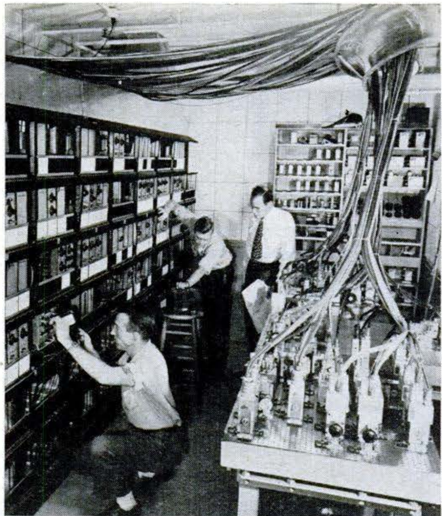
Bundle of wires connects Bemac's mechanical section, at right, with electronic section.
