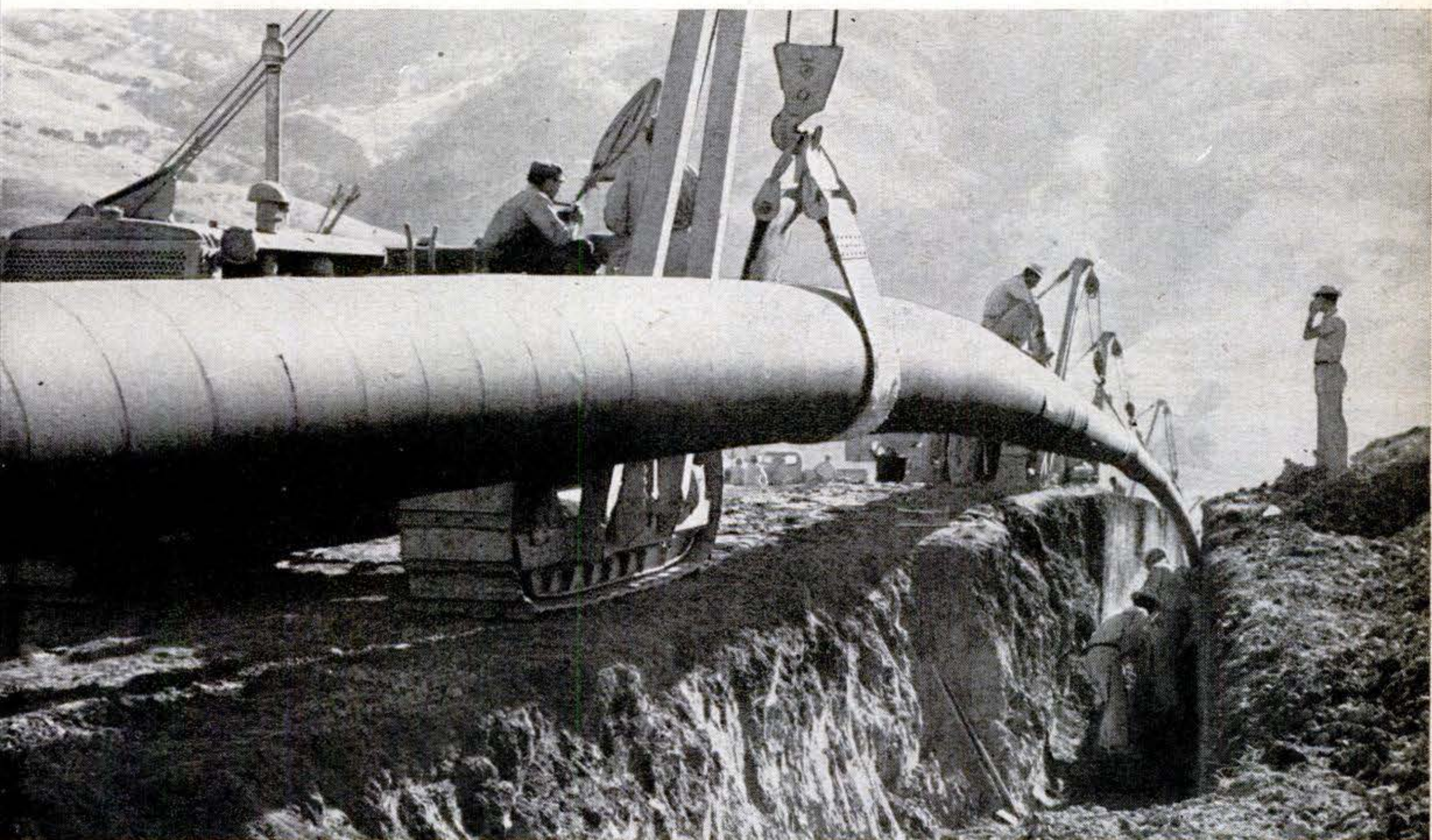
Side-boom tractors gently lower big pipe, with its preservative coating of asphalt and paper,
