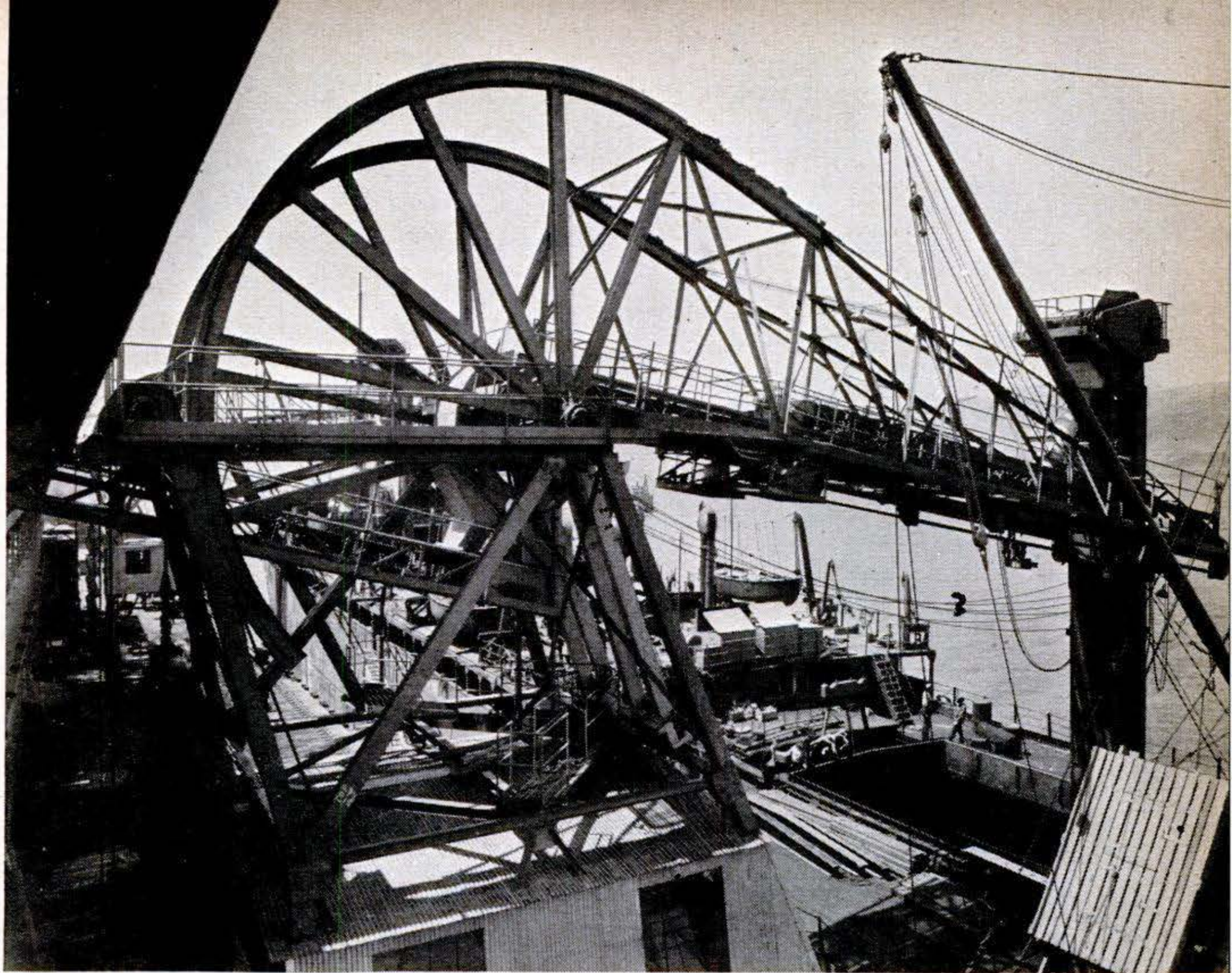
When ship with cargo of raw sugar docks at refinery above, a crane moves into place over the ship's hold, lowering its bucket conveyor to unload the sugar. The bucket lifts sugar onto conveyer belts that carry it to silos in refinery. ➤
