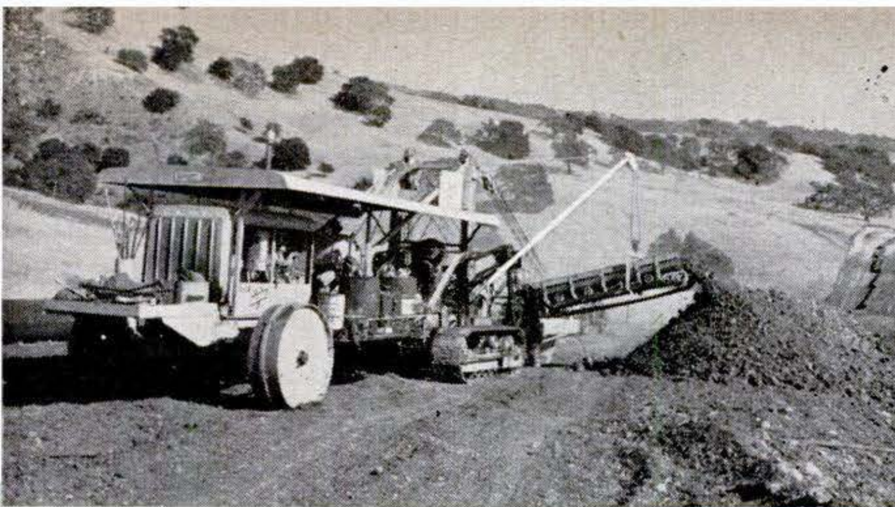
Above-ground part of trencher is seen in these front and rear views. The 32½-ton, self-propelled machine travels on crawler treads at any one of 32 different speeds, obtained by various
