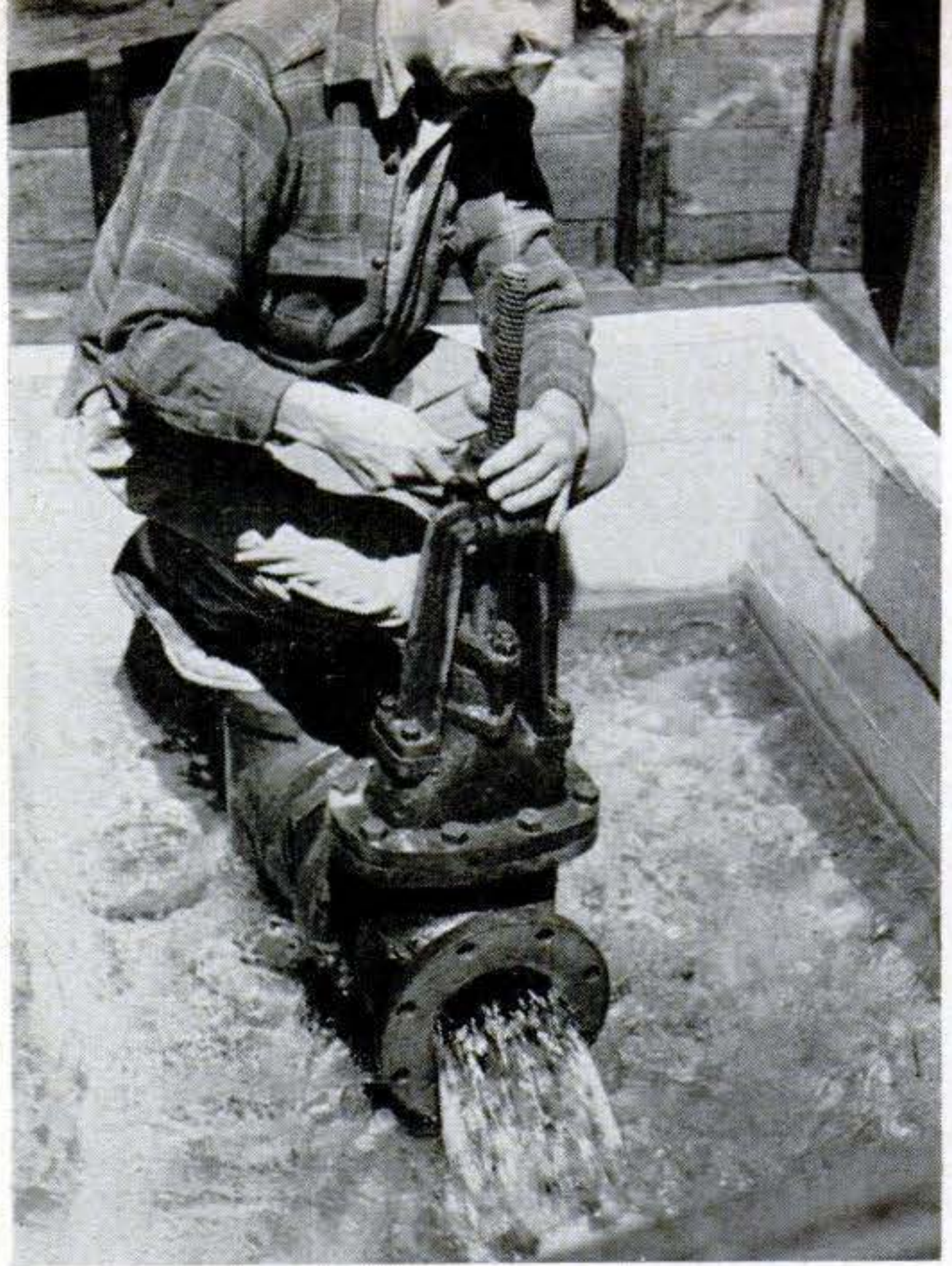
Nature does her own pumping in true artesian well like this one at the Vermont State trout hatchery near Bennington. It delivers a steady 250 gallons a minute from depth of 110 feet.
