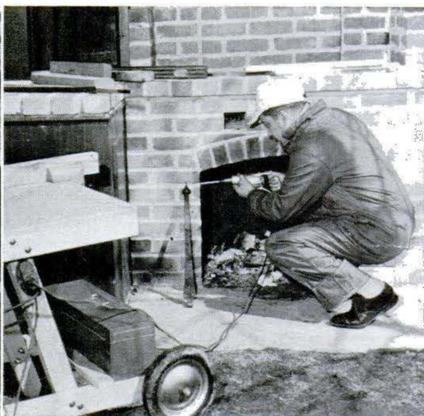
Triple outlet on leg of jointercart saves trouble of disconnecting and connecting main extension cord when drill is used.
