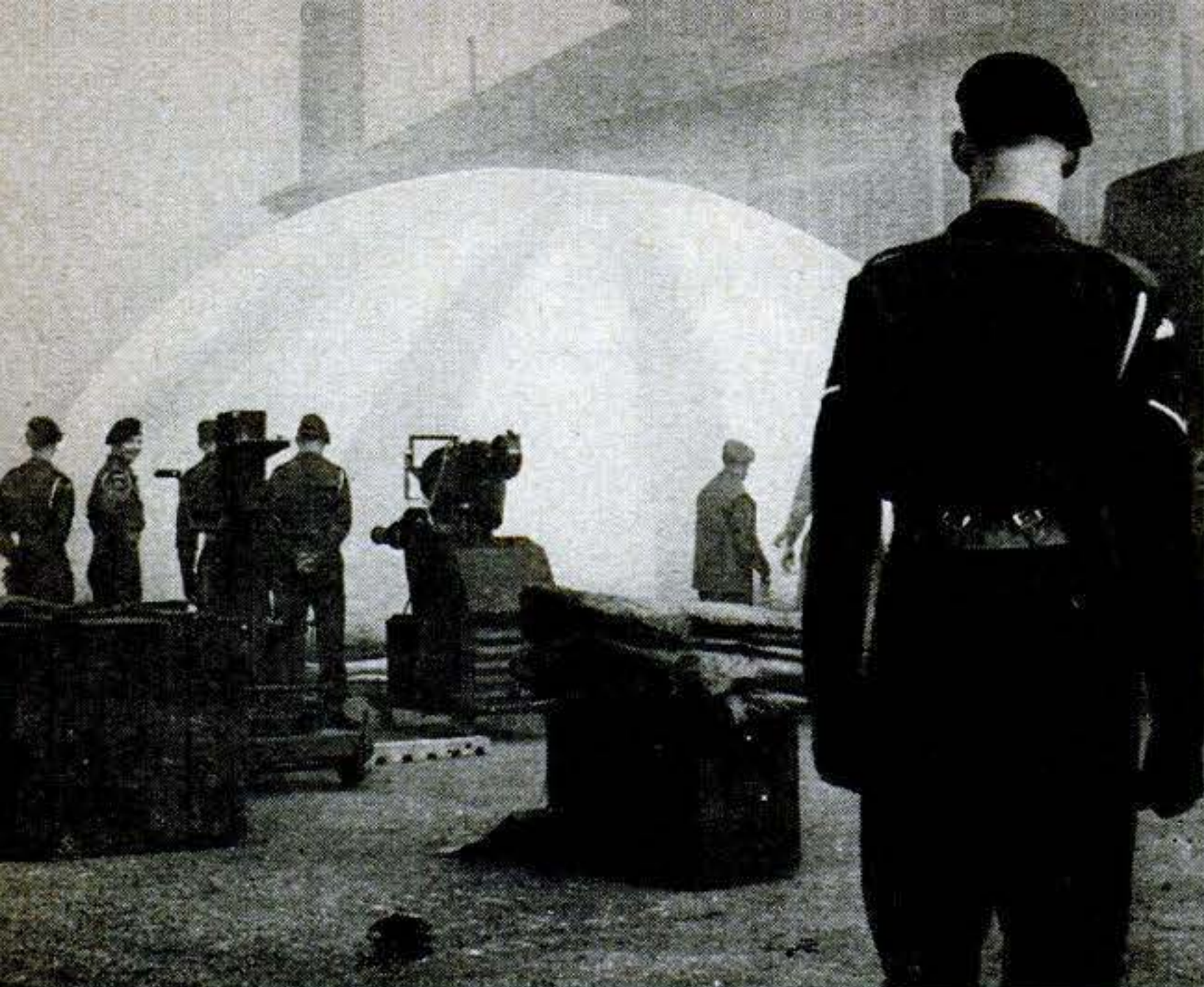
Fabric dome , 20 feet high and 30 feet across at base, is kept inflated by compressor. In center is large movie projector, ready to be moved in. Dome recently withstood 75-m.p.h. gale.
