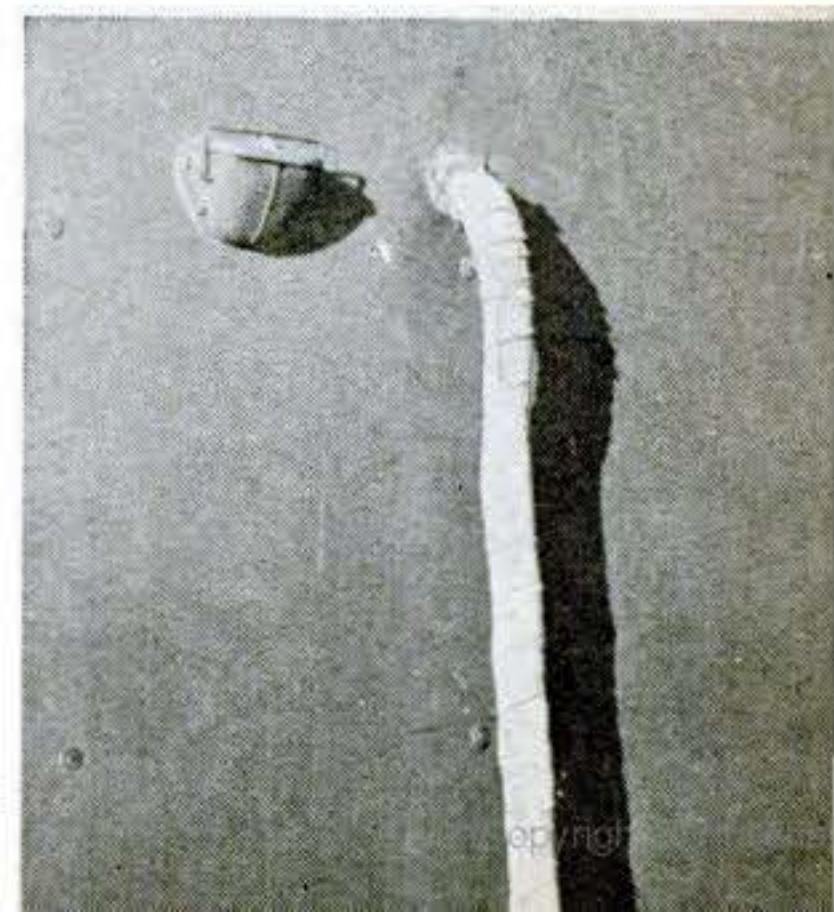
Insulate water pipe by wrapping with several layers of cloth and paper, right. Better yet, run pipe through trailer floor and box insulation around it, above. For long absences, install a shut-off valve.
