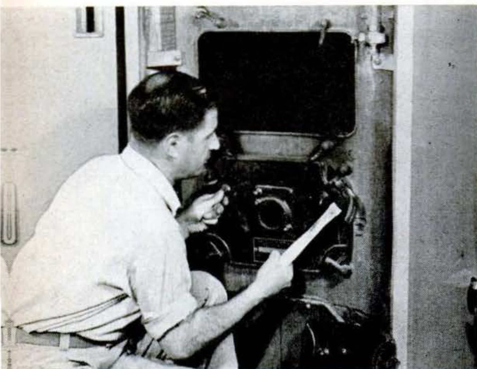
Water-heating operation left my furnace hot, so I allowed it to cool first. Drop-off type doors shown must be held while dogs are turned.
