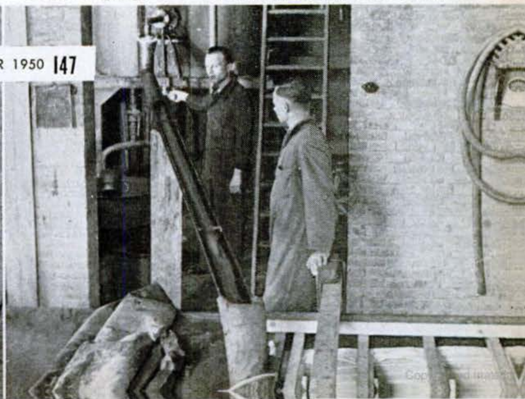
6 HOT PARAFFIN WAX flows through tube into after end of mold. It cools in about 24 hours, forming ship model, which then is ready for final shaping. [Continued on next page]
