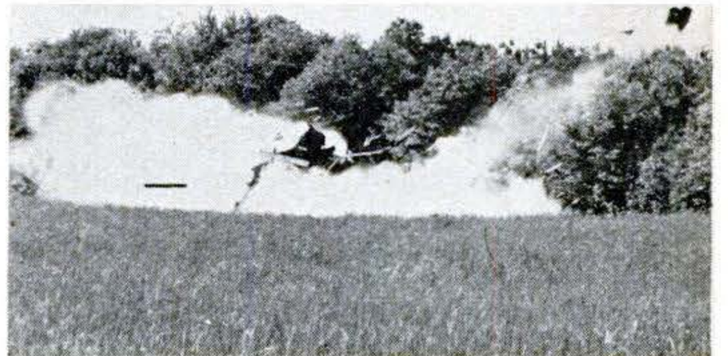
Building is blasted to kindling as overheated water hurls shell of storage tank 400 feet into the air and 100 yards across country.
