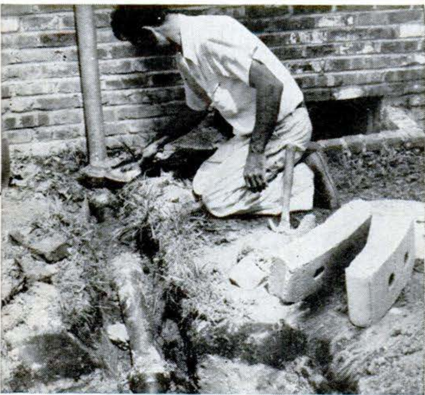
Cement the tile joints , using mortar made of one part cement to three of fine sand. Pack oakum into bell before working in the mortar.
