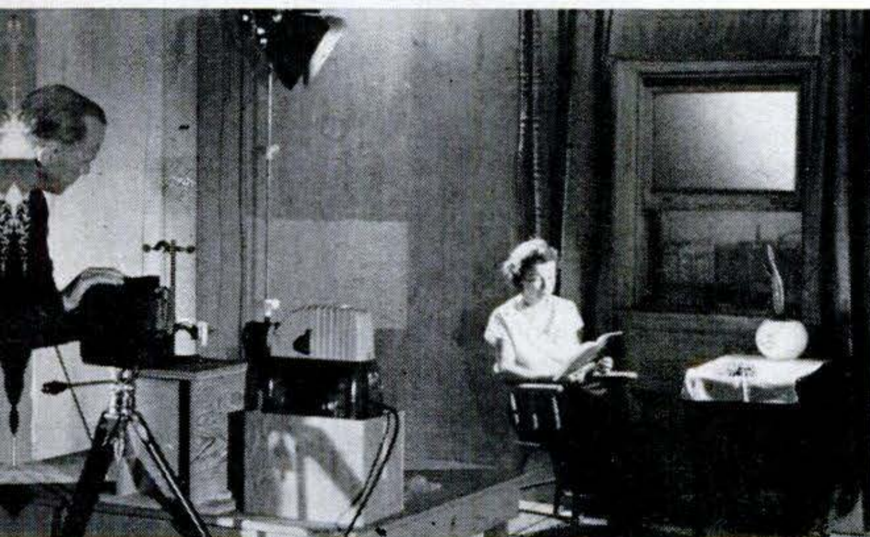
Front projection to provide more realistic backgrounds is still experimental. Method may save costs over conventional rear projection.
