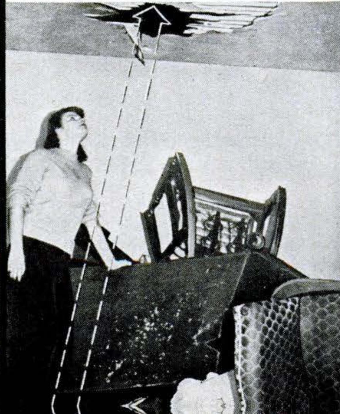
Arrow shows tank's path from cellar through roof.
