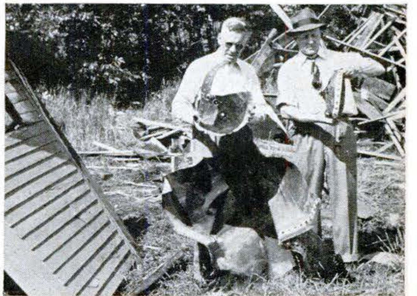
Here are remains of 30-gal. tank in which water under only 80 lb. pressure was heated to 290° F.—78° over normal boiling point.
