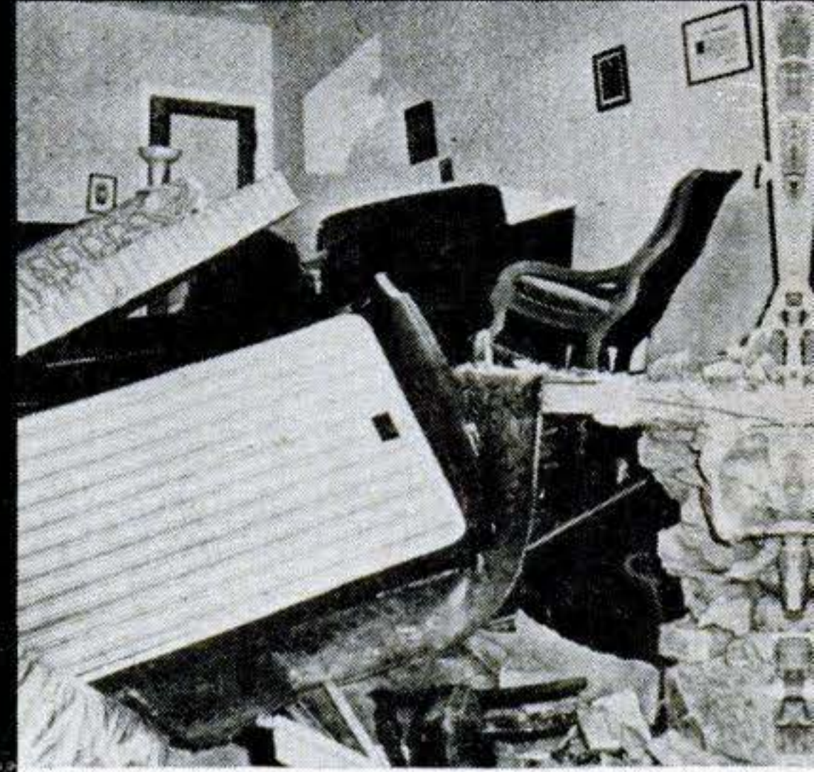
Overheated water tank wrecked brick house.
