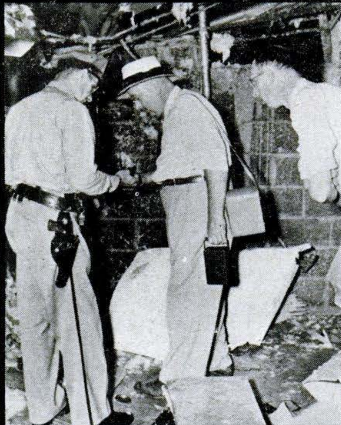
Investigators say missing tank had no safety valve.
