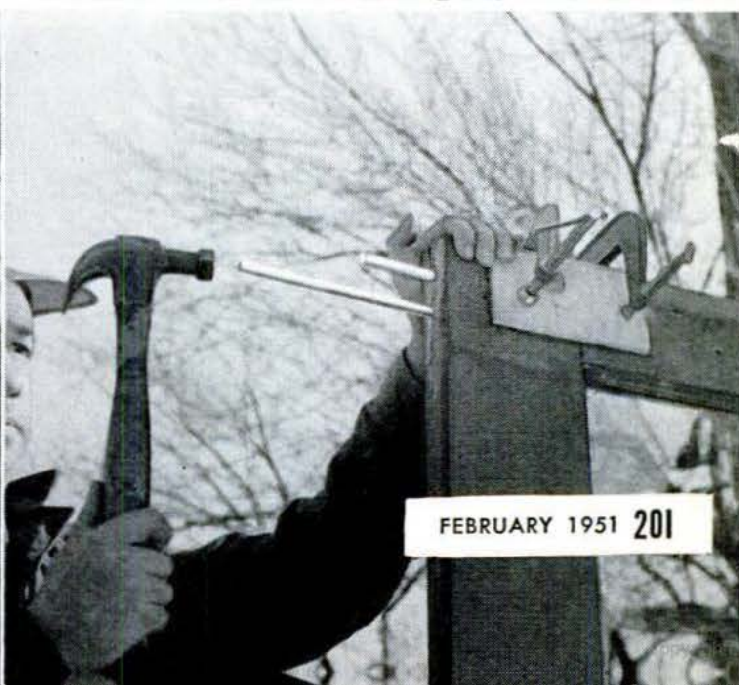
the bottom. Then holes were bored, and hardwood dowels, coated with glue, were driven in.
