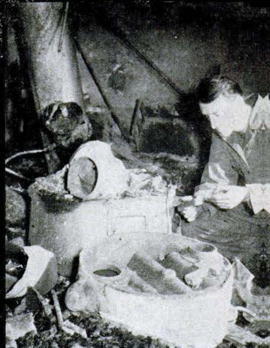
Pennsylvania homeowner and ex-furnace.
