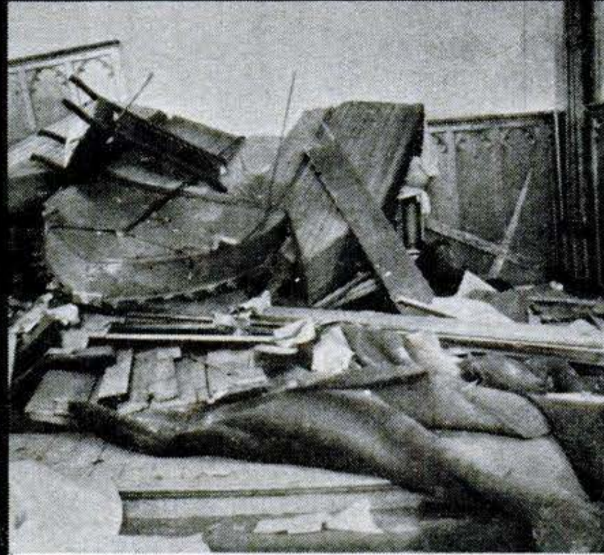
Someone left gas on after supper in church basement.
