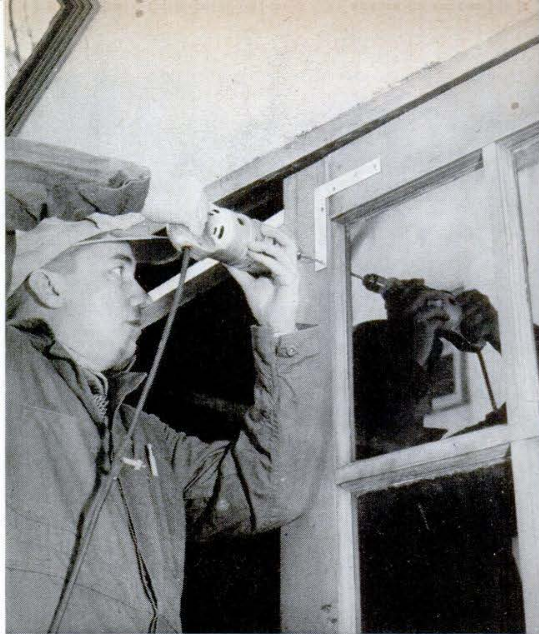
Right-angle mending plate , mounted with wood screws or through bolts, is another means of tying together a re-glued joint. Use the biggest plate you can. A second plate inside the door can be held by the same bolts.
