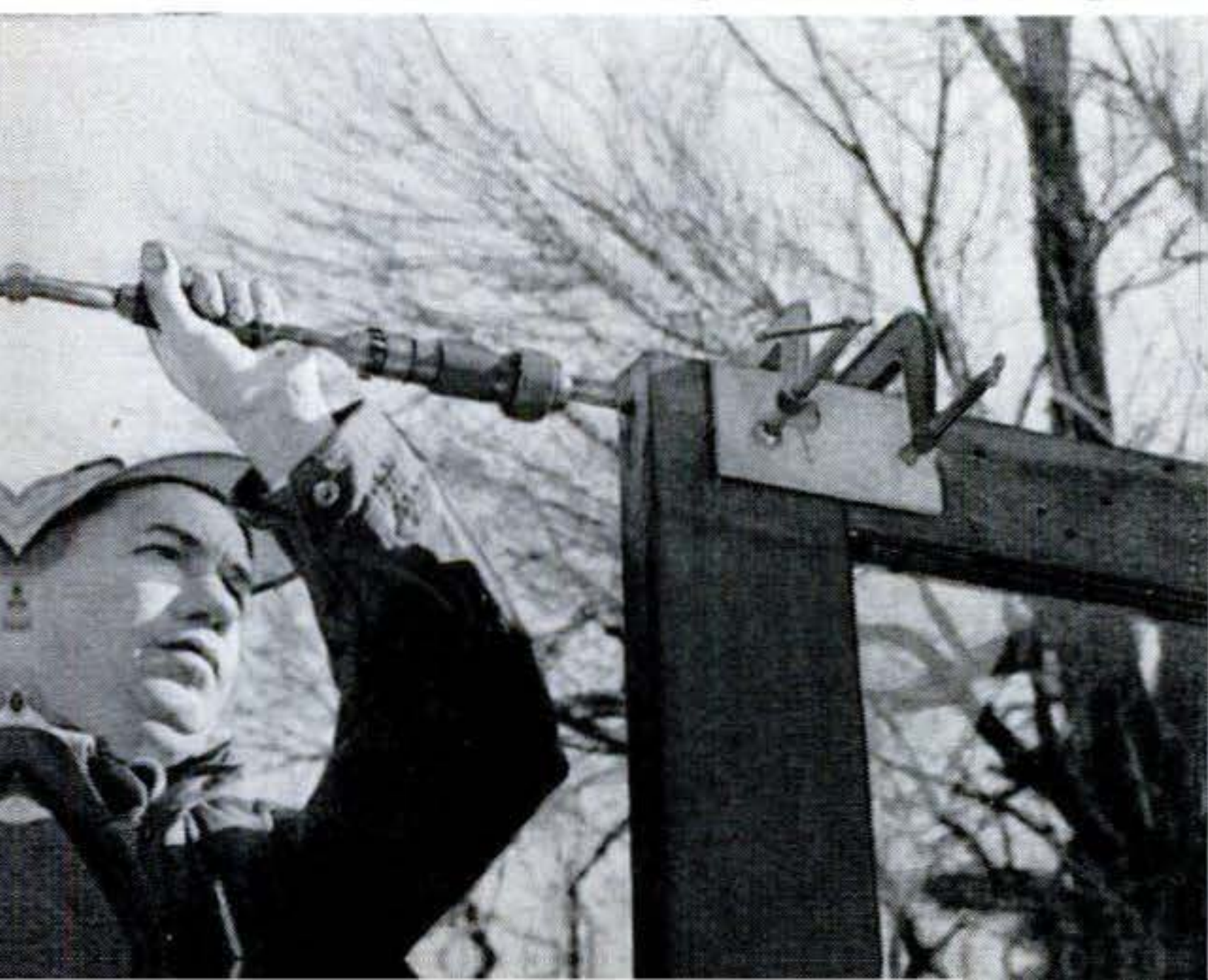
Broken joint was clamped as shown to align the faces, the stile being raised by a wedge at
