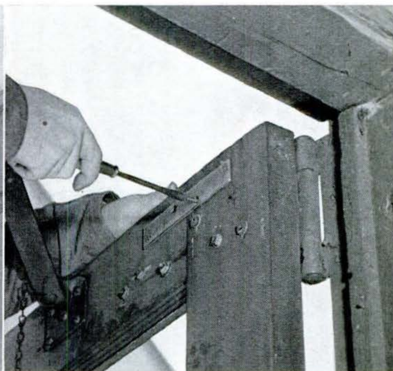
right through hinge and rail (left). Flathead bolts were inserted, and the nuts were tightened over washers on the inside of the rail. Then a metal mending plate was put on the inside of the door to help hold the joint together.
