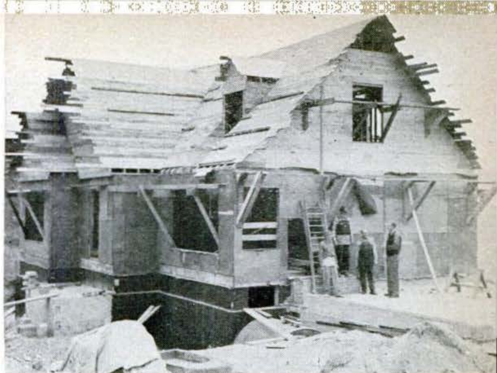
House that Auto Surplus Built: The materials for this unusual home came from surplus stock of an automobile factory. Page 130
