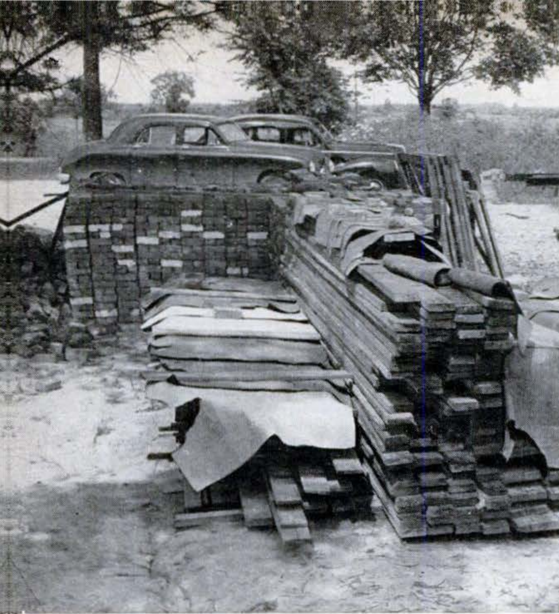
Five-member family spent weeks removing mortar from reclaimed bricks (background) and nails from lumber. Owner Barenow and son Dick, 23, did much of the heavy construction.
