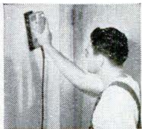
Repairs—Fitting screens, smoothing plaster patches.
