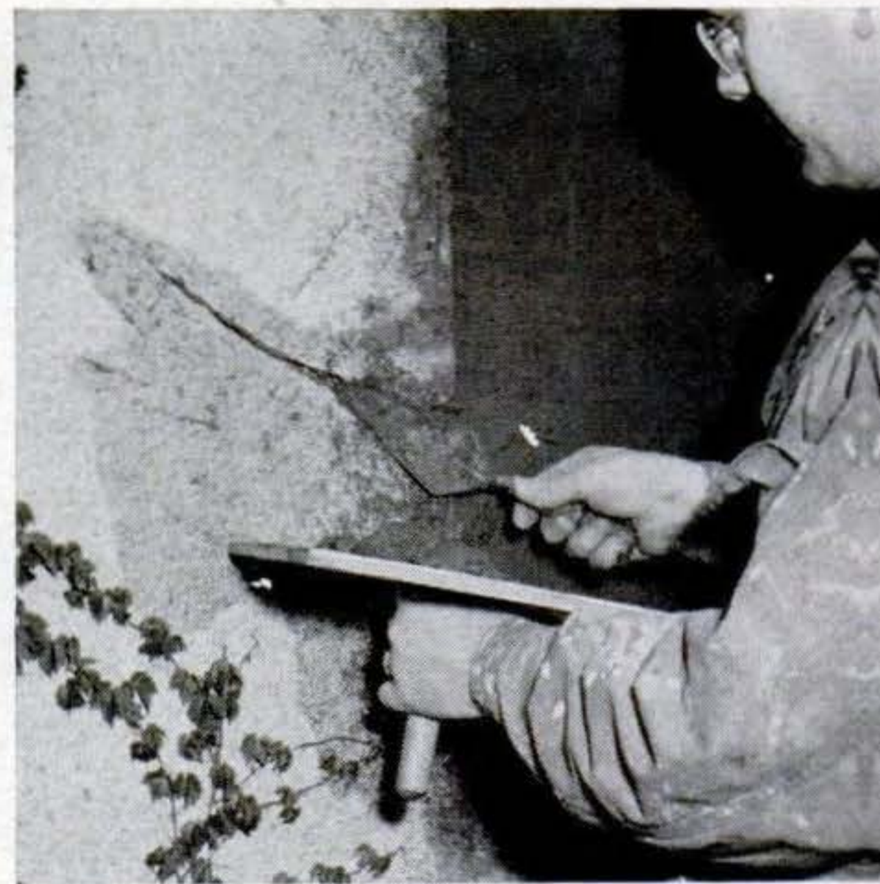
Fill crack, packing mortar in tightly with a small trowel. Deep cracks that expose lath should be filled with two coats of mortar.
