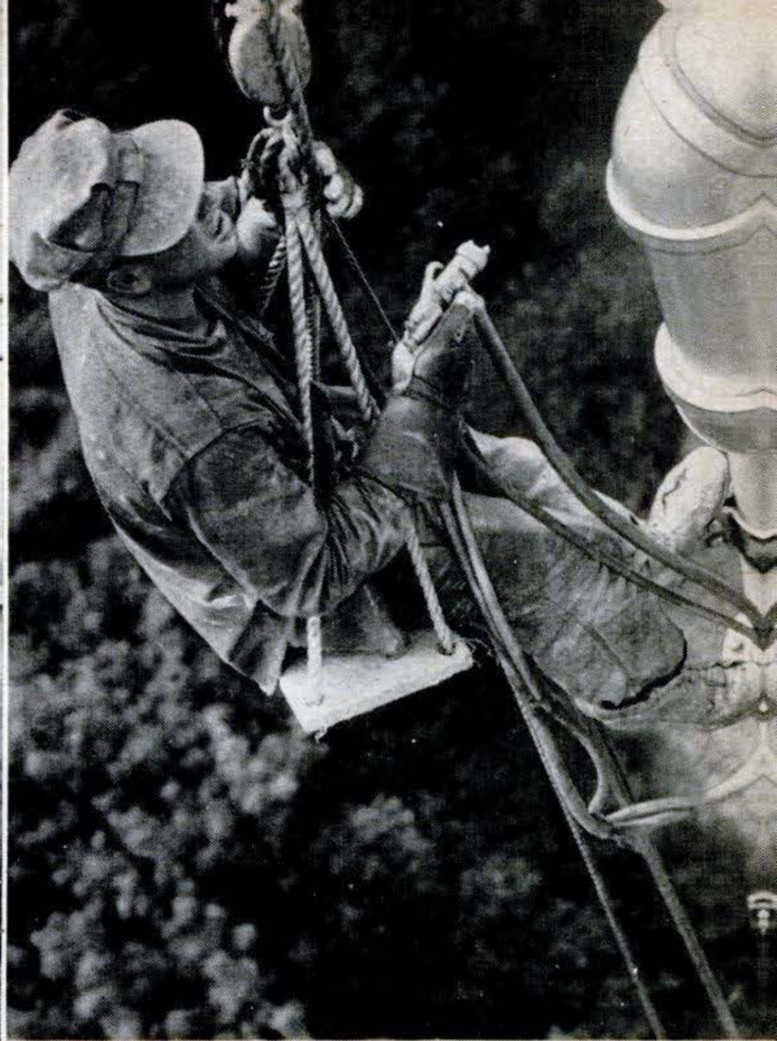
Painter above the treetops. Secure in his bosun's chair, and holding a spray gun attached to several hundred feet of hose, he starts down the legs of a tank. To get at hard-to-reach spots, he may have to stand up on his chair.
