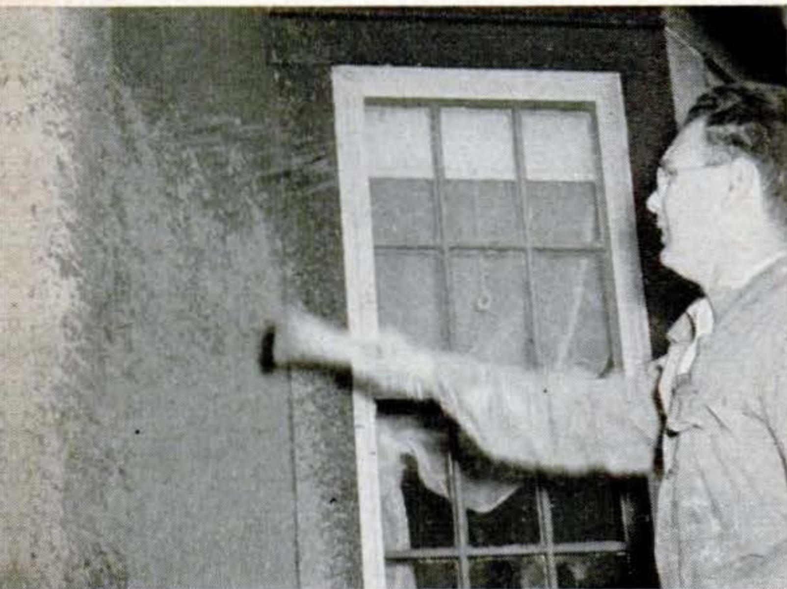
19. Cover hardened second coat with thinly spread mortar. While it is still wet, spatter on the stucco coat with a whisk broom.
