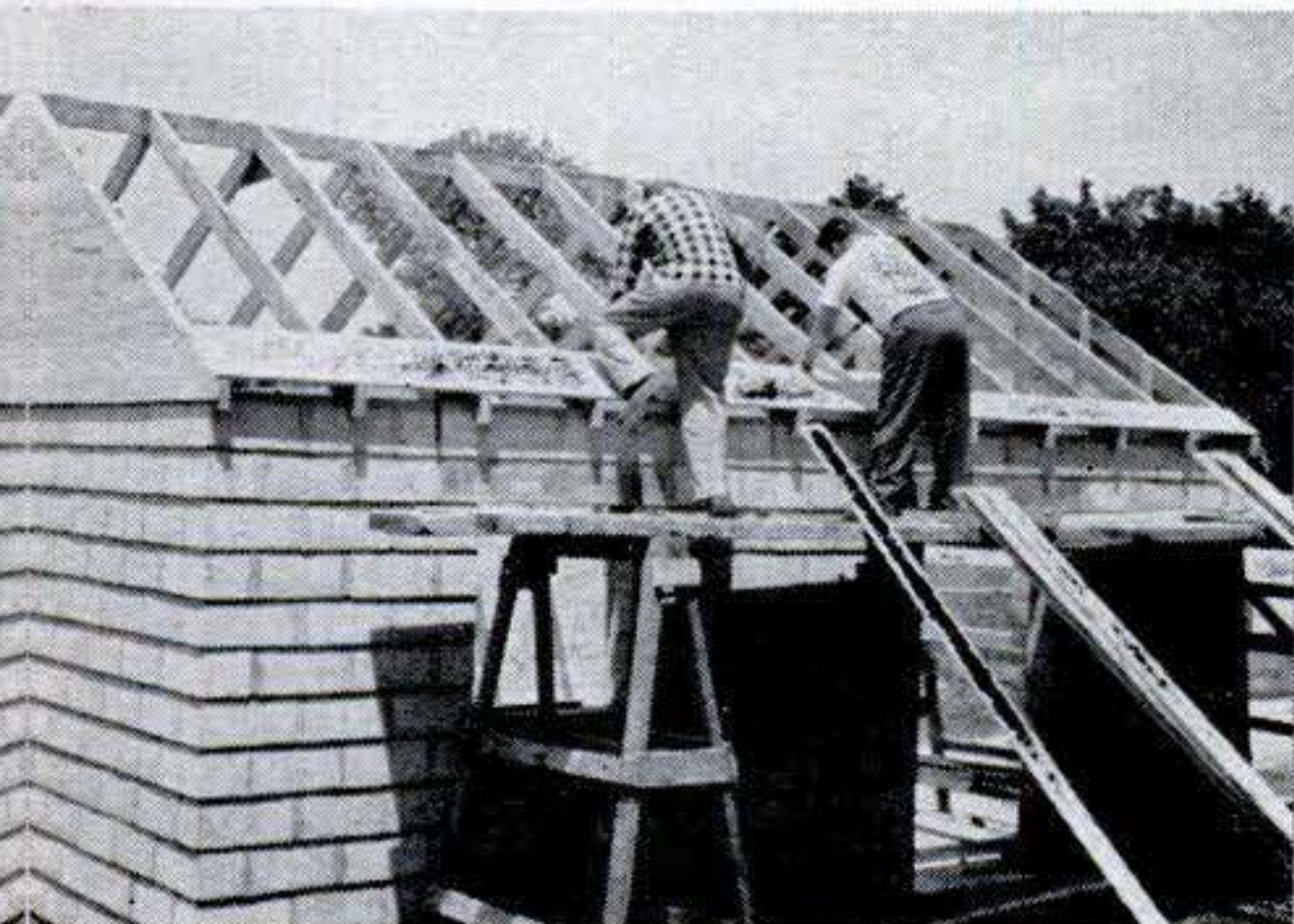
10. Sheathing the roof. Tongue-and-groove sheathing is nailed to rafters (below left). To get tight fit, drive point of old screwdriver into
