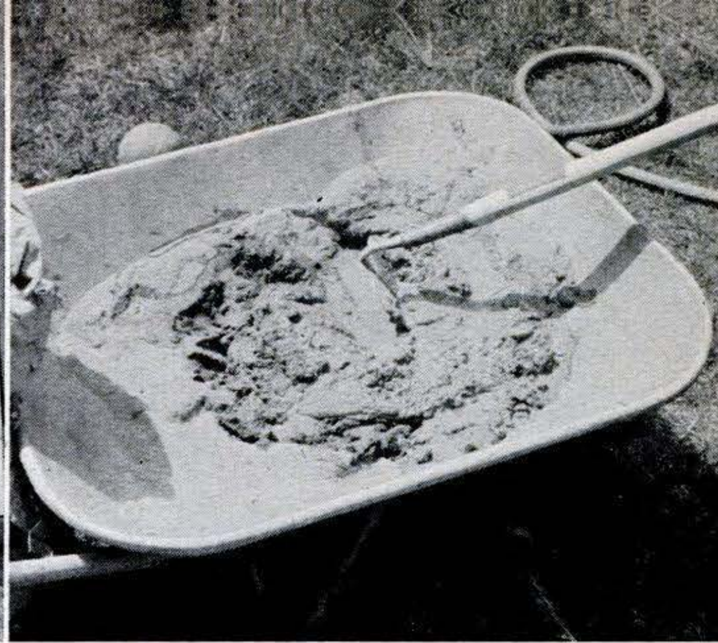
9. Ready-mixed cement and sand —sold at building-supply yards—is your best bet for small jobs. Metal wheelbarrow is good mixing pan.
