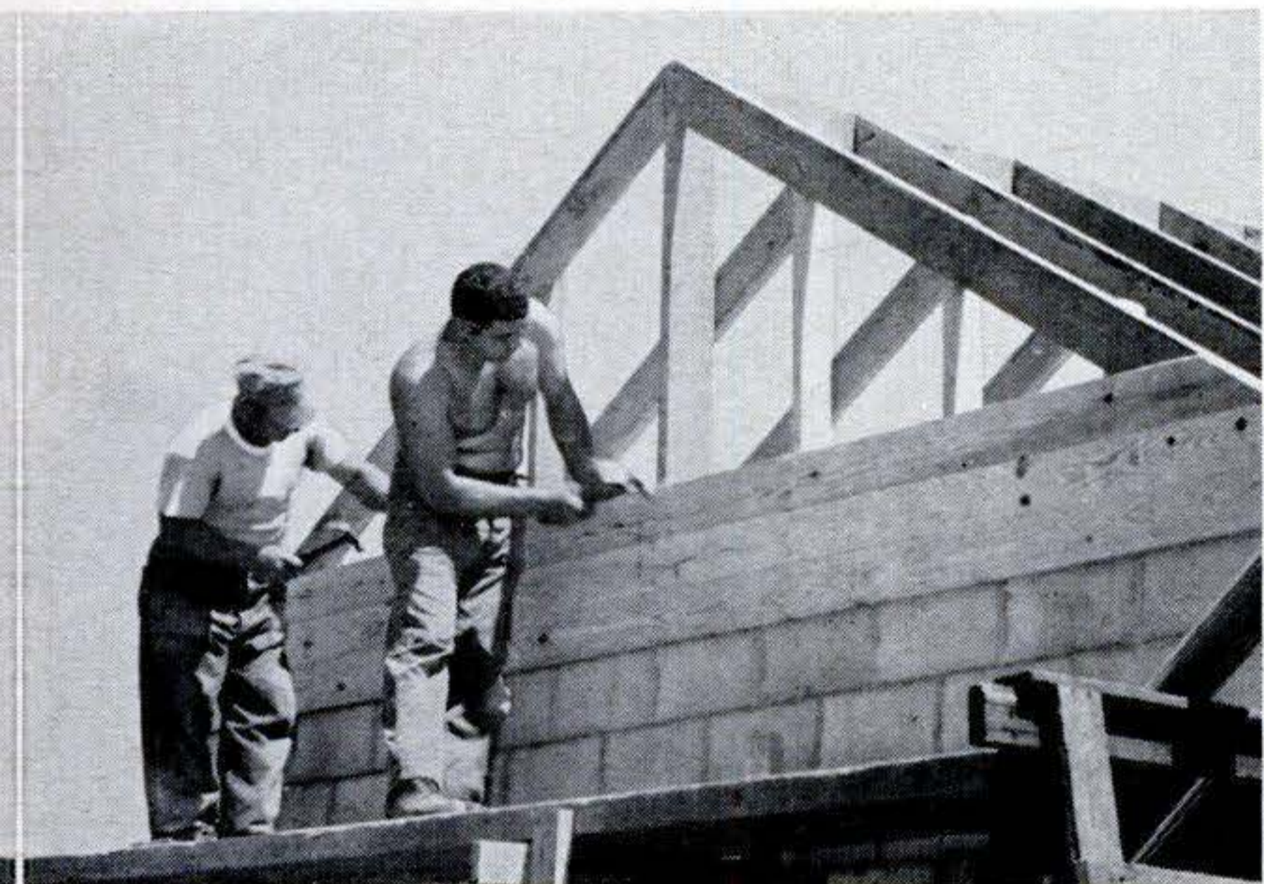
8. Sheathing the gables. Six two-by-four studs are nailed between plates and rafters at each end of garage. Sheathing is nailed to studs and to two-by-sixes that support ridge pole. Sheathing is trimmed flush with end rafters.
