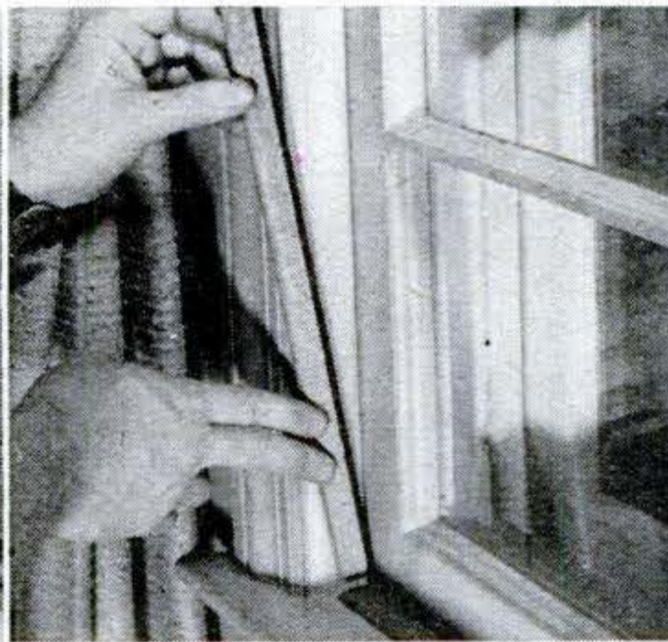
WOOD-FELT type is bradded around windows and doors like molding. Corners should be mitered. This type can be painted to match trim.
