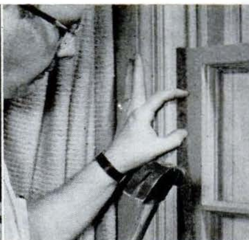
HAIR FELT is tacked to window frame so it presses against sash snugly but loosely enough to permit sash to be raised and lowered.
