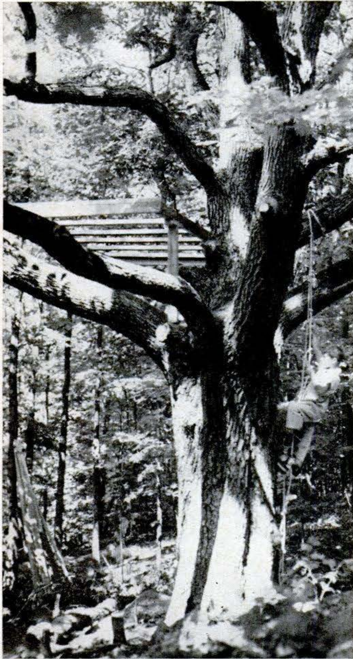
THE BOUGH of this white oak, nearly horizontal, gave Jeremy the tree-hut idea. Dead and injured limbs were trimmed and stumps sealed with paint before construction began.
