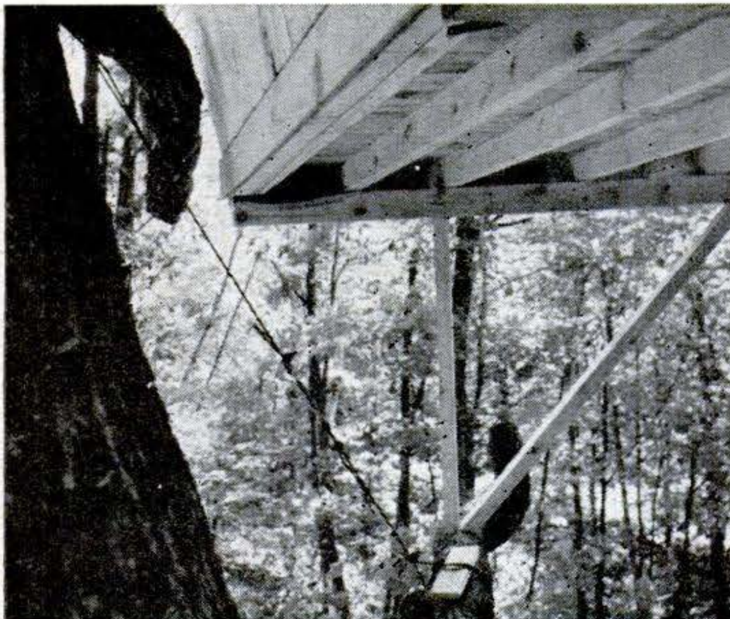
LIMBS are never exactly where you want them; and there are never enough of them to bear the weight. We built up from low branches and dropped cables from high ones.
