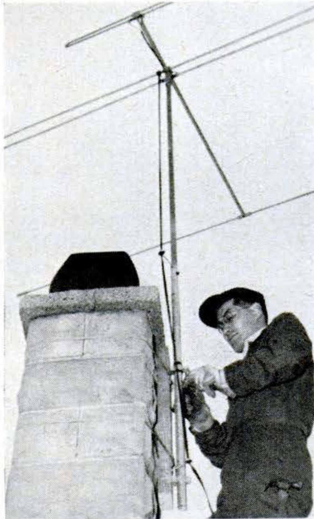
WOOD SHIM makes it easy to mount an antenna mast on a chimney with an overhanging cap. Strap a two-by-four to the chimney first, then fasten on the mast clamps with lag screws into the wood.
