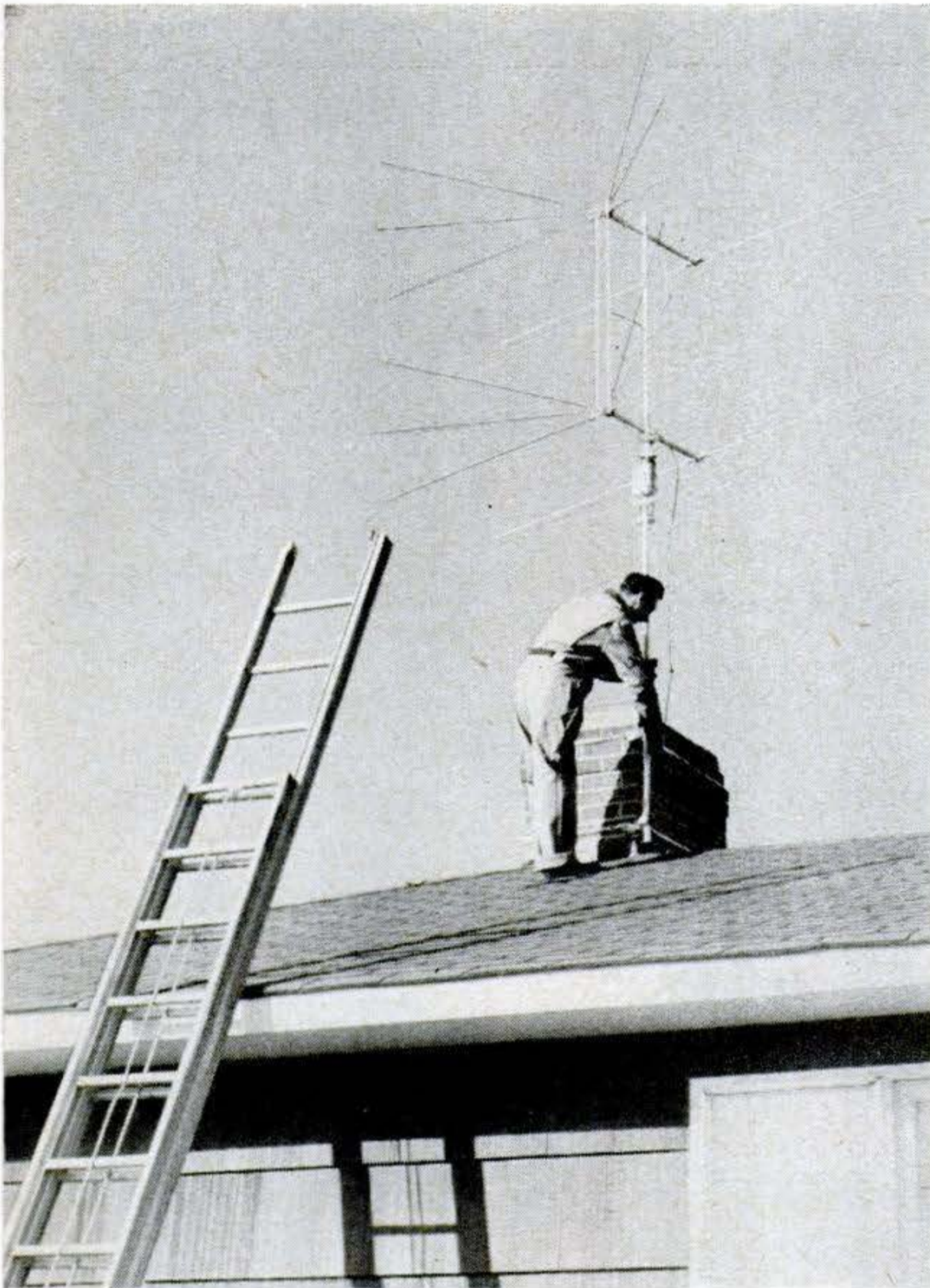
VHF ANTENNA , covering channels from 2 to 13, comes assembled and snaps open in an instant. This conical type, made by JFD, can be used singly in strong-signal areas or in stacks up to three for distant reception.
