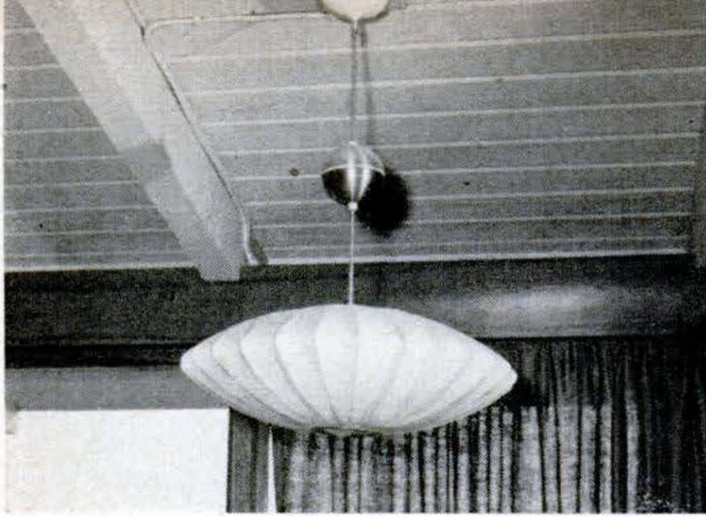
EXPOSED WIRING , painted to match ceiling, is unobtrusive. Nonmetallic cable, permitted in most states, is used. The bubble lamp pulls down for dining and Junior's homework stint.
