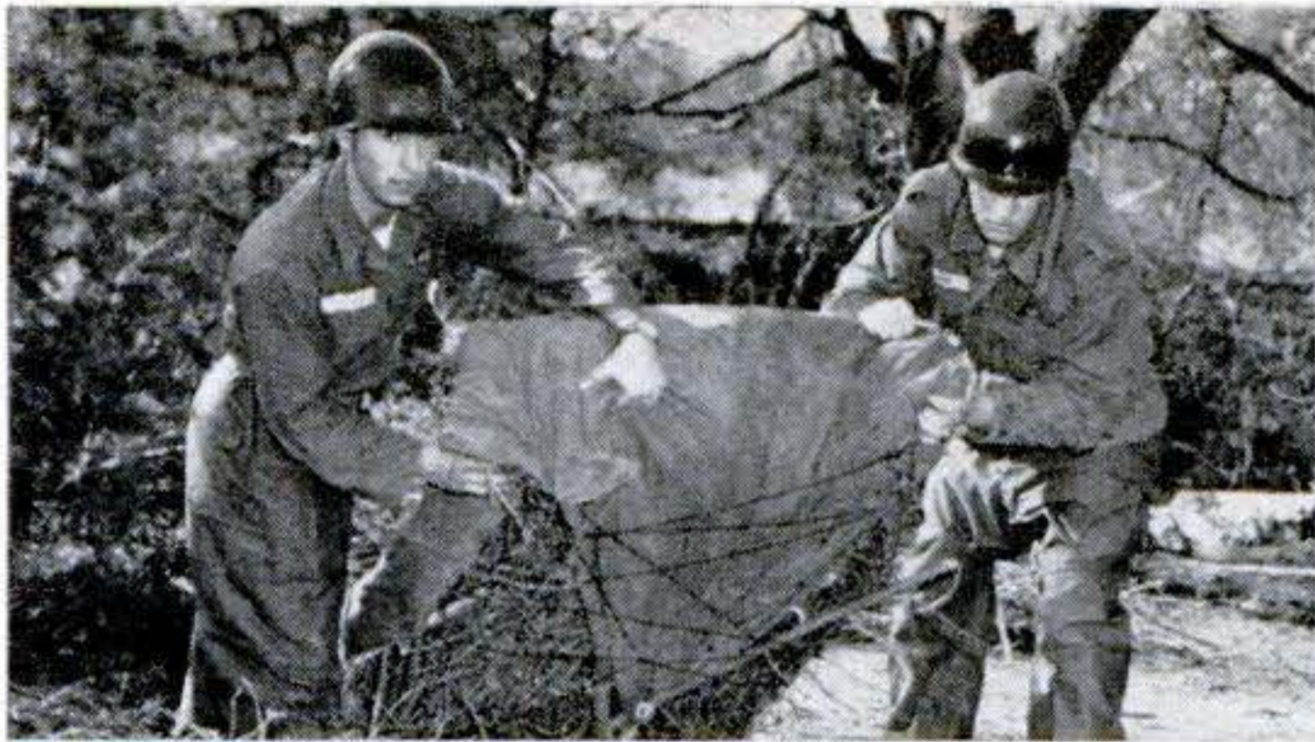
MAKE-DO BRIDGE. GIs in field training at Fort Hood, Texas, improvise from what they have. Above a pontoon is made of sticks lashed in pup-tent halves; at right rope and sticks make the tread.
