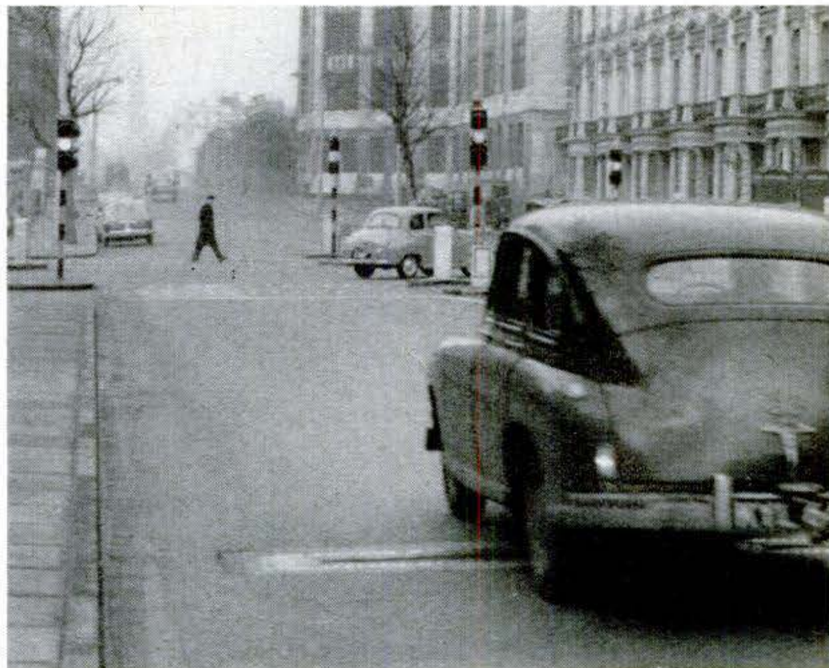
RED-LIGHT BEATER. A car's speed is electronically measured as its wheels cross these twin channels—to hold the green signal and let the car get by. The system is being tested in London.
