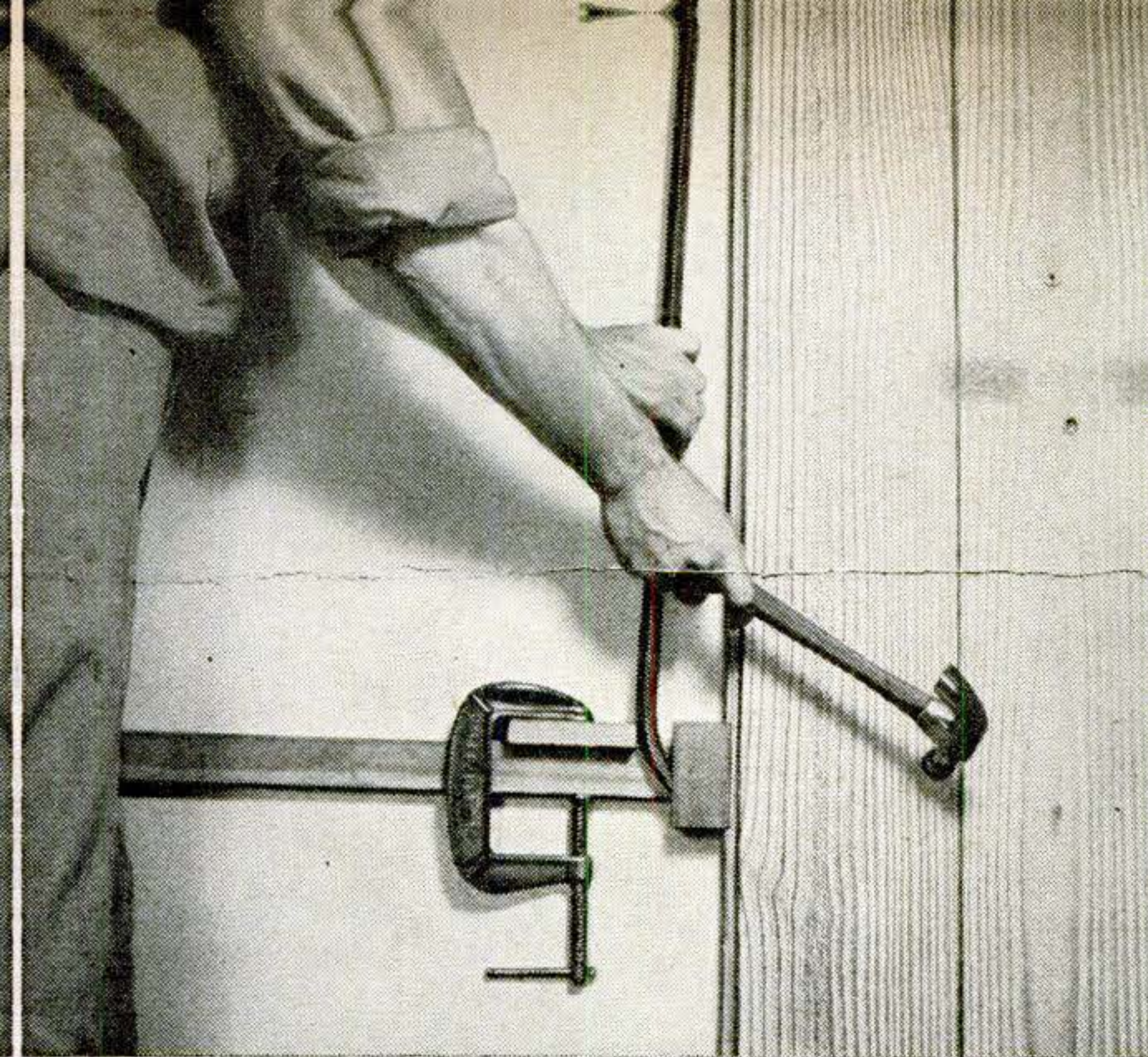
NUDGE STUBBORN PANELS into place with this setup. Wood block clamped to the furring strip makes an adjustable rest for the crowbar.
