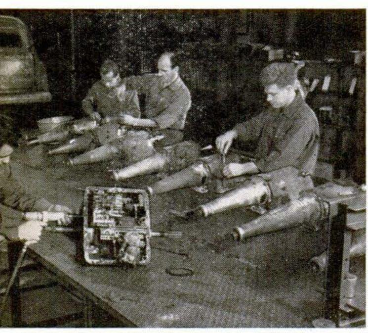
EIGHT FORDOMATICS are about to become a basketful of parts. This disassembly bench is the only dirty spot in the shop. The old units are dismantled here prior to cleaning.
