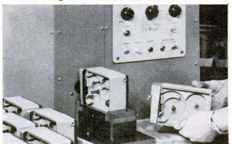
ELECTRONIC FRAME-COUNTER checks film travel assures movies that move at correct speed.
