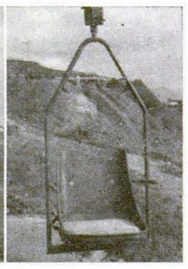
safety feature on the chair's trolley is a spring-loaded cam. If the pulling cable were to snap (an unlikely possibility), the safety cam would automatically grip the load-carrying cable and prevent the chair from speeding down to the bottom of the bluff.
