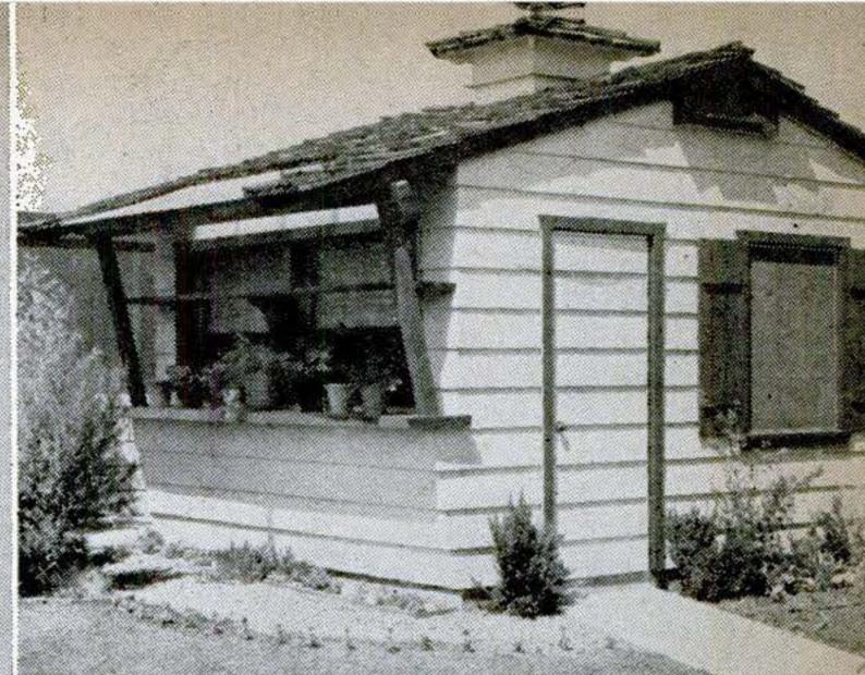
inal was tied into the construction of a garden house at the rear of the home of Mr. and Mrs. A. M. Brook of Los Angeles. It's provided with a skylight of corrugated plastic, notched into the pro-
