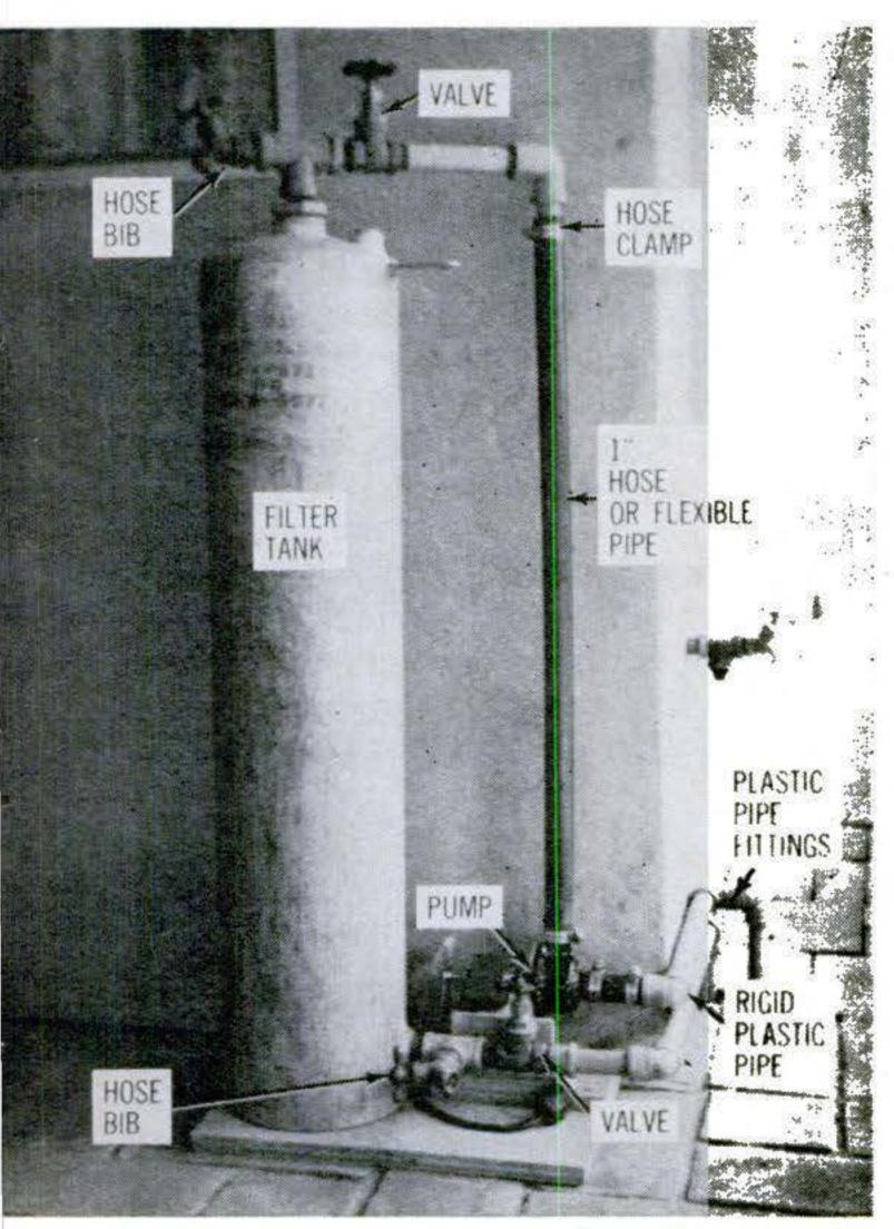
connections may vary, depending on the type of tank used, but the basic arrangement illustrated above should be followed. Filter and pump are mounted on a plywood platform. A removable plywood cover, shown below, has vents for air circulation around the pump motor.
