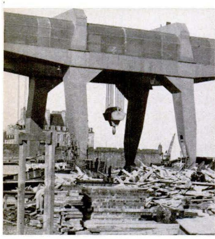
GIANT SEA CRANE. This big frame, straddling dock facilities like a huge sawhorse at St. Malo, where it was recently installed, is a major addition to the French port. The new traveling hoist has a lifting capacity of 235 tons.
