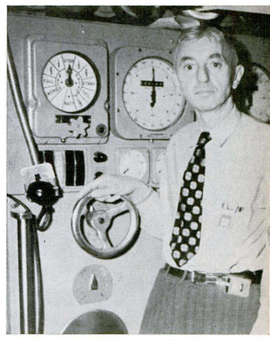
Hand on the throttle (it's a real sub throttle), Rickover gets the feel of atomic power the day Mark I engine is first started up.
