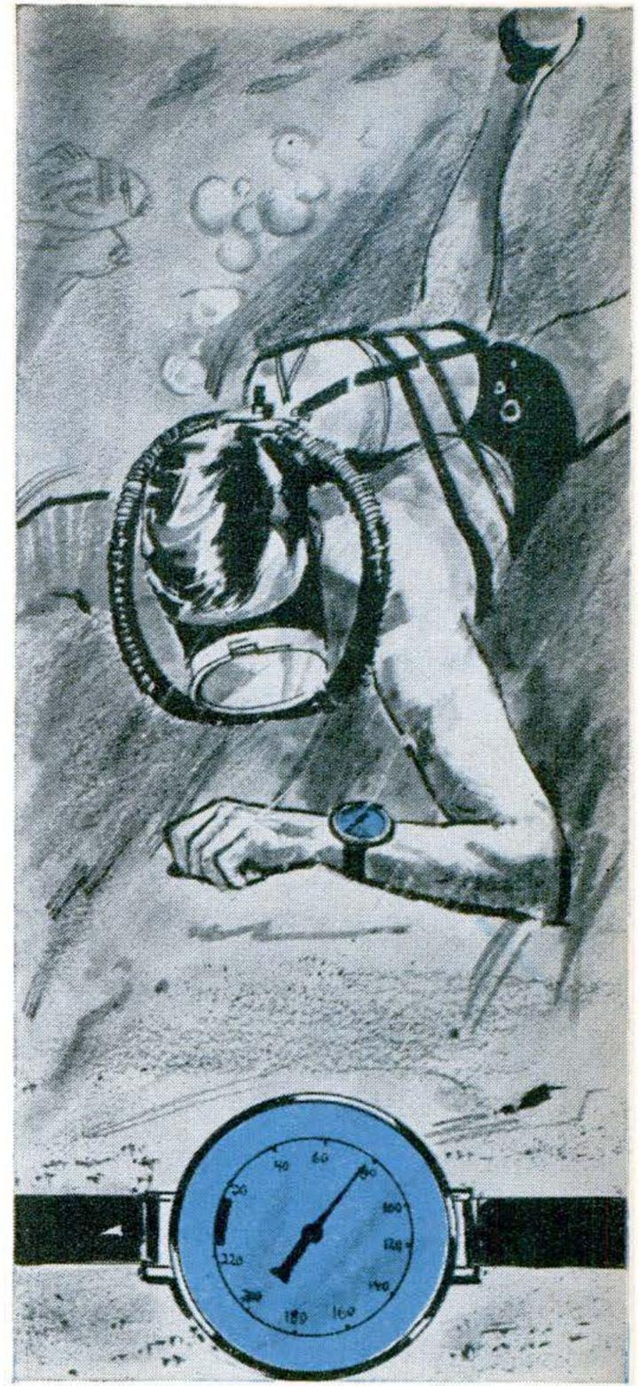
Gauge Shows Diver's Depth. This wrist gauge, using a new principle, has its Bourdon tube encased in oil. The oil transmits water pressure on a flexible membrane outside to the tube inside. Deflection of the tube, in response to pressure, would move a dial pointer.
