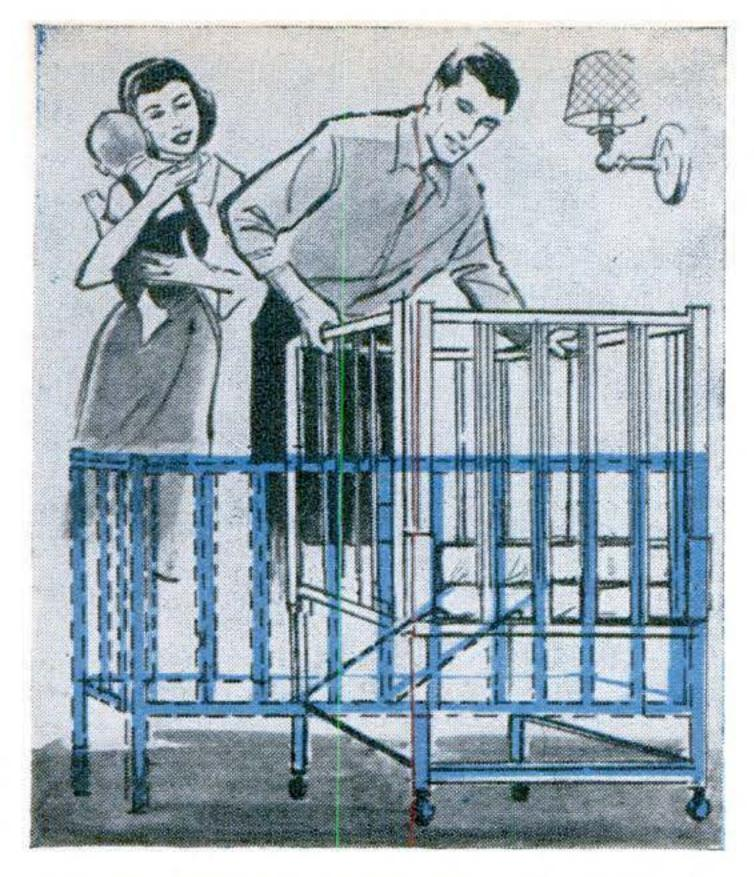
Crib Unfolds into Play Pen. You'd need less space for baby's basic furniture if he could sleep and exercise in one combination unit. To convert this play pen into a crib, you'd fold in half two hinged sides and the base. The legs would extend to bring the unit to crib height.
