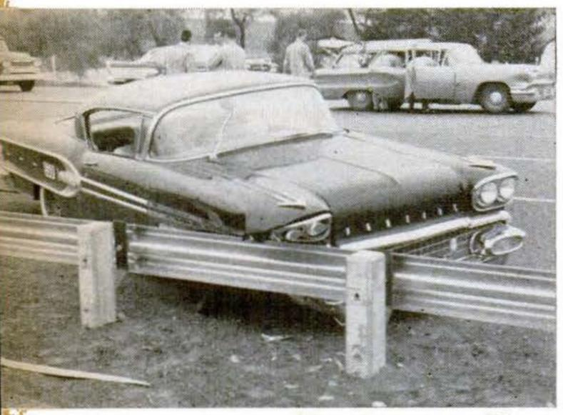
**STRUCK AT 35 M.P.H.**, this spring-mounted beam rail guided car to a safe halt with relatively little damage to either car or fence.
