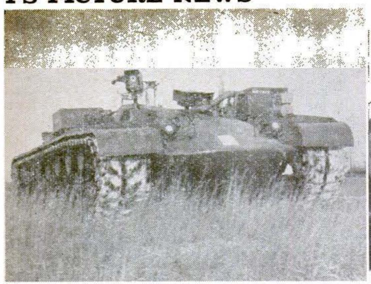
TV CAMERAS and power equipment are mounted on top of a medium tank for testing. In actual combat they would be inside the vehicle.
