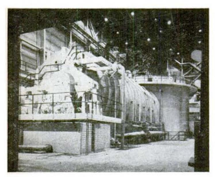
The landlocked sub: stern in foreground, then long engine room, with atomic boiler in tank behind.
