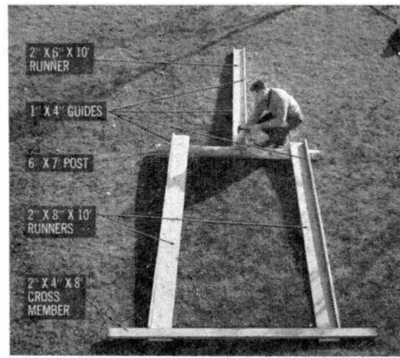
TO ASSEMBLE RAMP, drive bolts into holes drilled in runners and cross members. Wheel runners are spaced to fit wheels of trailer. Tongue runner is centered. Edge guides keep wheels and tongue from wandering off the ramp.
