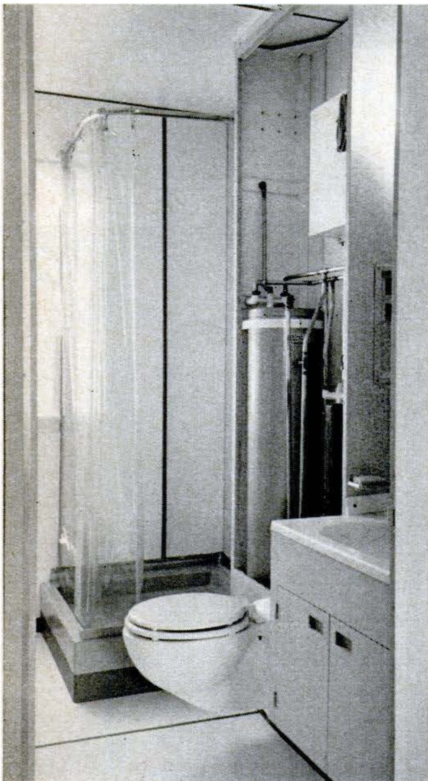
Compact utility core packs all plumbing in a cabinet 3' wide and 1' deep. All kitchen and bathroom cabinets fold flat, so they can be easily collapsed and reerected on a new site. A structural wall of Loc-Pac panels through center of the house supports the roof panels.
