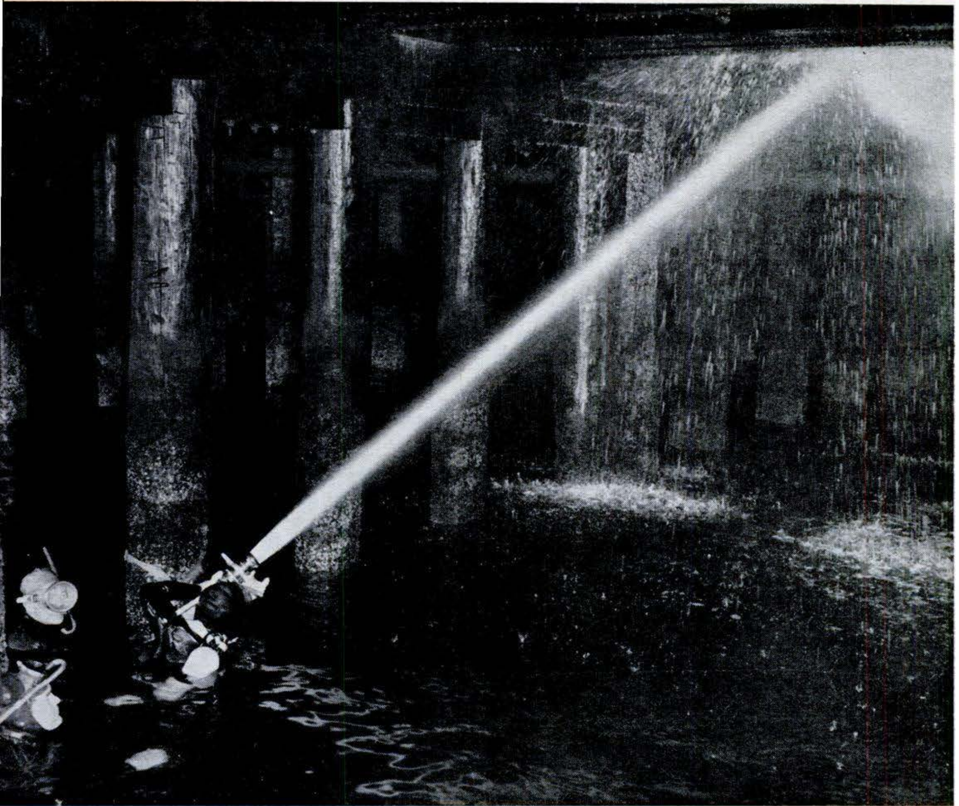
Streams of water poured in from under dock penetrate complex of tar-soaked and creosoted timbers.
