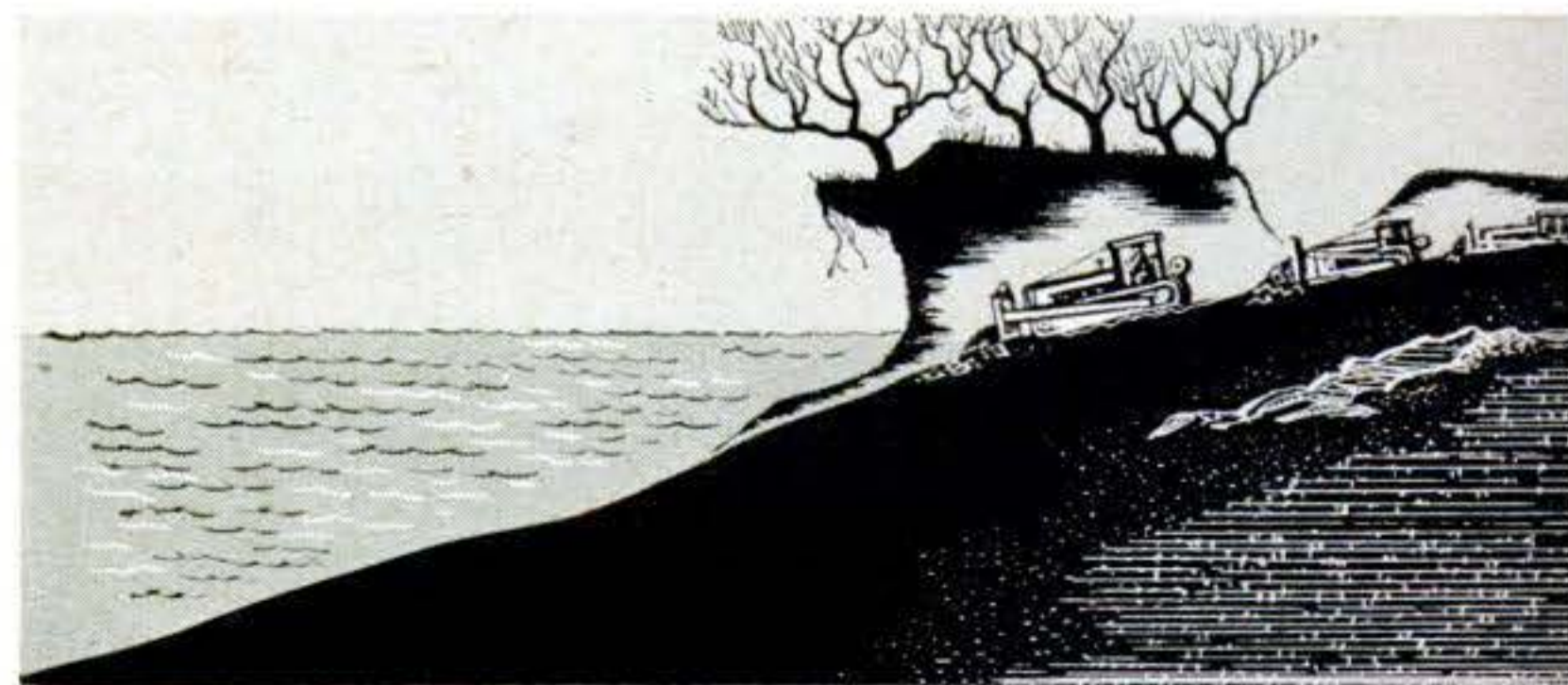
D-6 dozers begin smoothing down torn bluff, pushing piles of dirt down for the garmouth.
