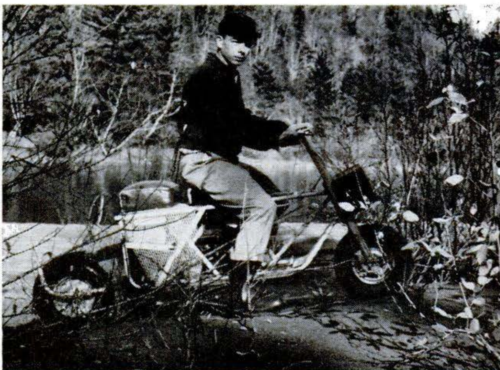
2. Extra traction of third wheel and track lets Tote Gote zip through mud and loose sand.
