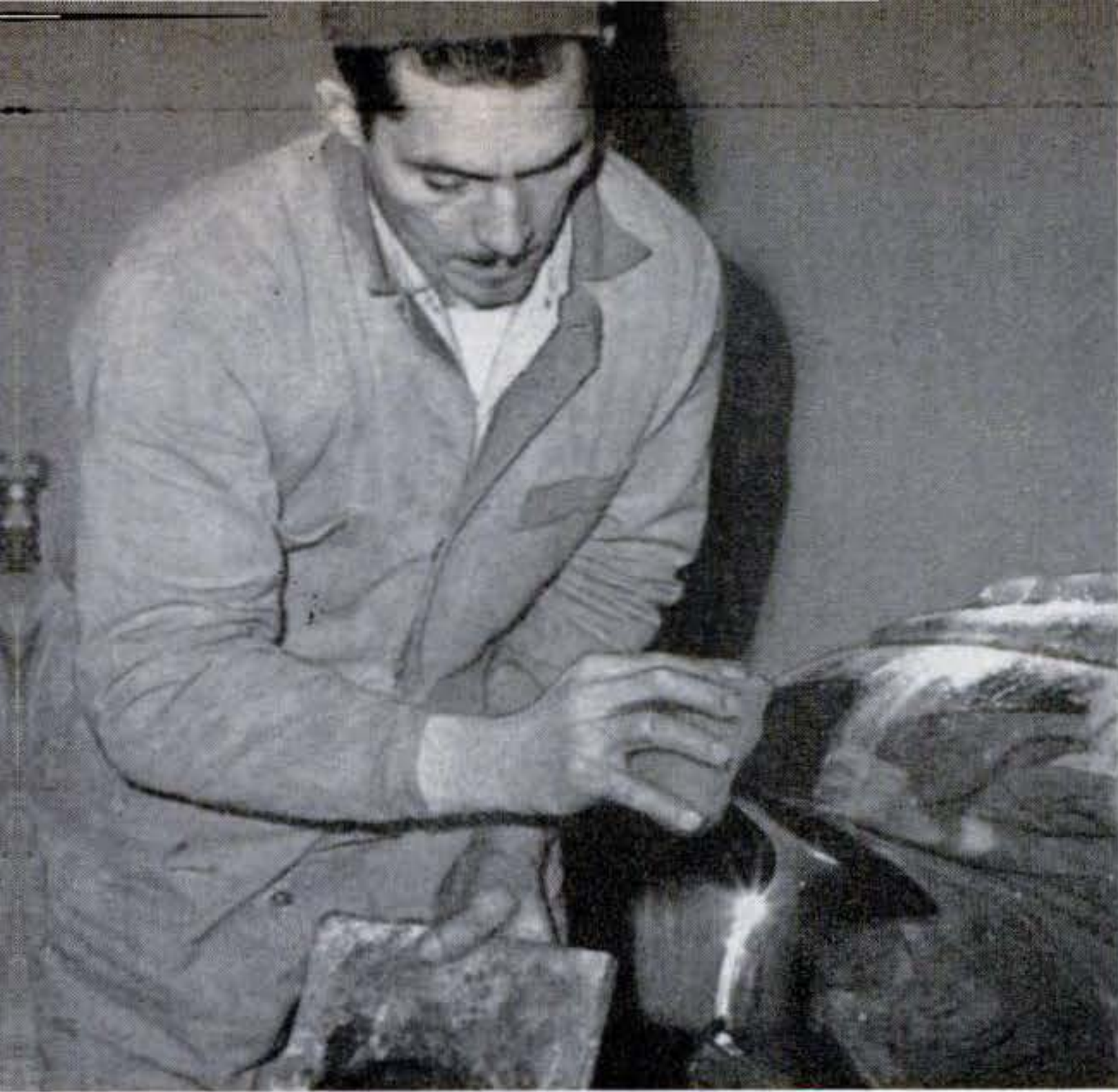
To cover small scratches, this mechanic is applying a thin coat of plastic filler. Some good body men insist that plastic usually should not be more than \frac{1}{8} or \frac{1}{16} of an inch thick.
