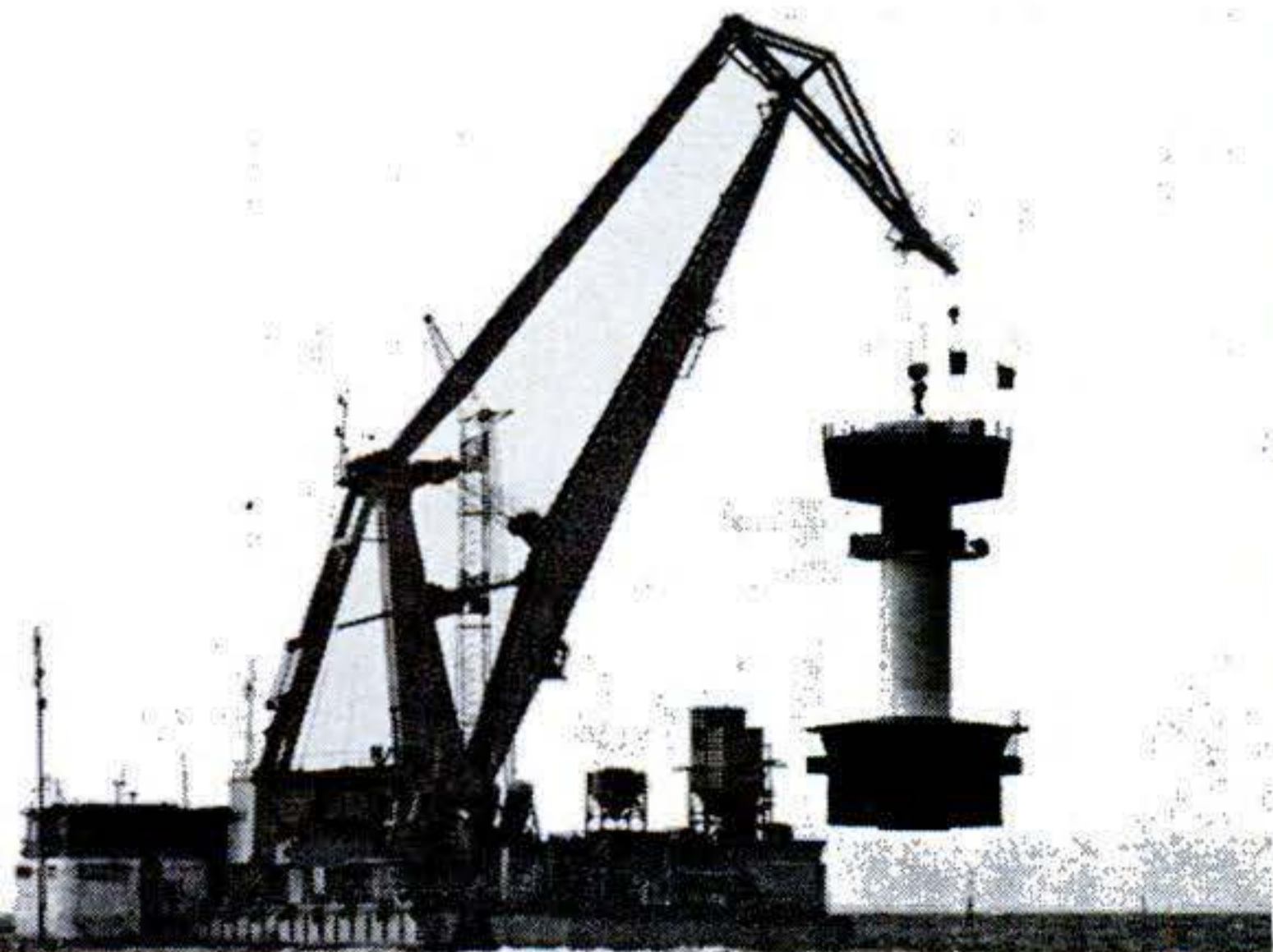
Giant floating crane raises assembled 100-foot-tall lighthouse to carry it to concrete-island base.
