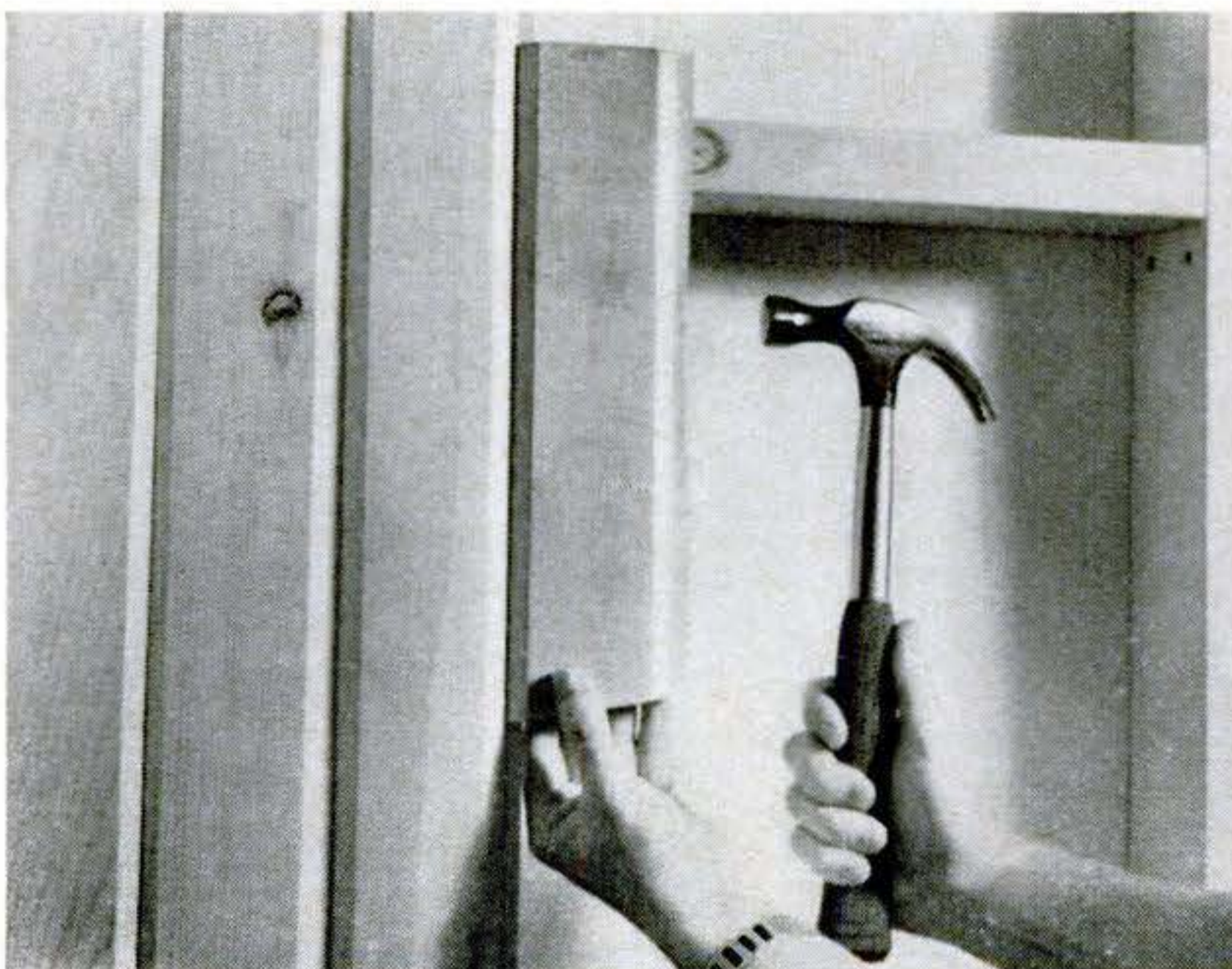
Warped or tight-fitting paneling may need a little help to make snug joints. Use a scrap piece over the tongue and pound it tight. Hold and nail.
