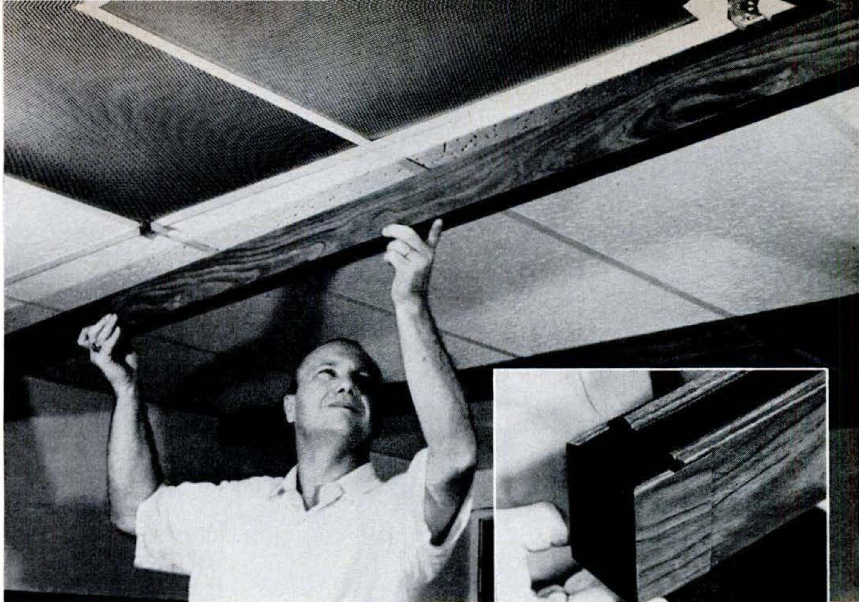
Celotex Snap-Fast vinyl-surfaced metal beams with walnut wood-grain finish go up on any ceiling. Metal clips support the beams. The clips lock onto suspended-ceiling grid members with a twist. Metal splicer (right) joins sections.
