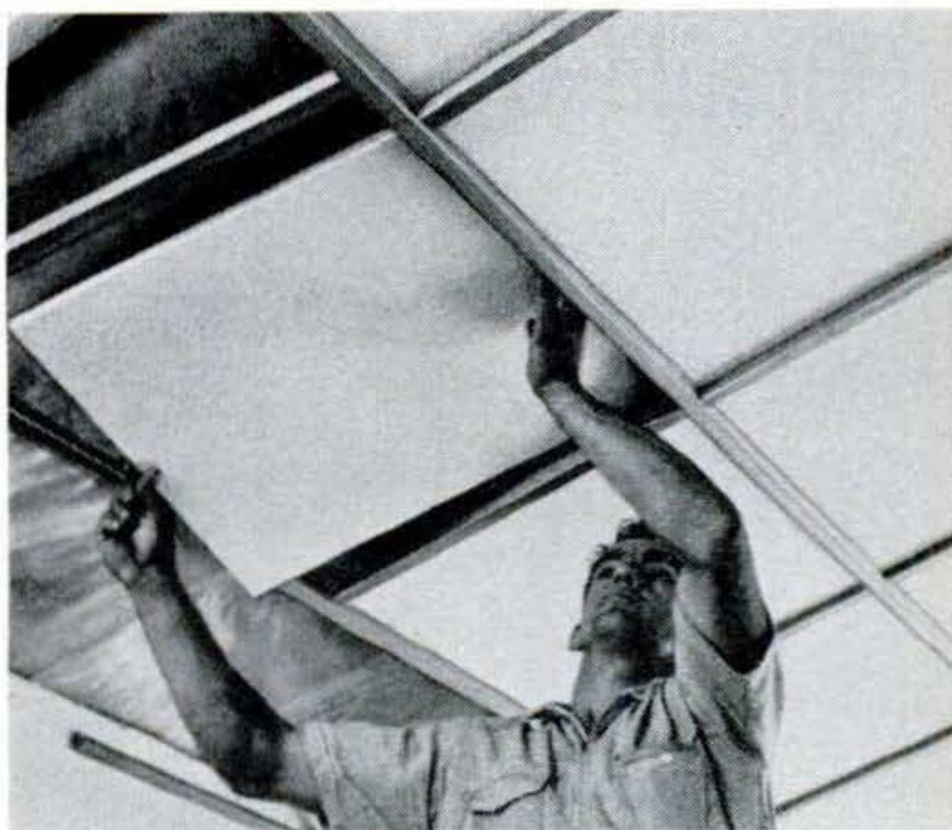
Precut redwood ceiling beams add elegance to a new do-it-yourself suspended-ceiling system made by Simpson Timber Co. Hanger straps nailed to ceiling joists support the beams. Ceiling boards fit solidly between the grids.
