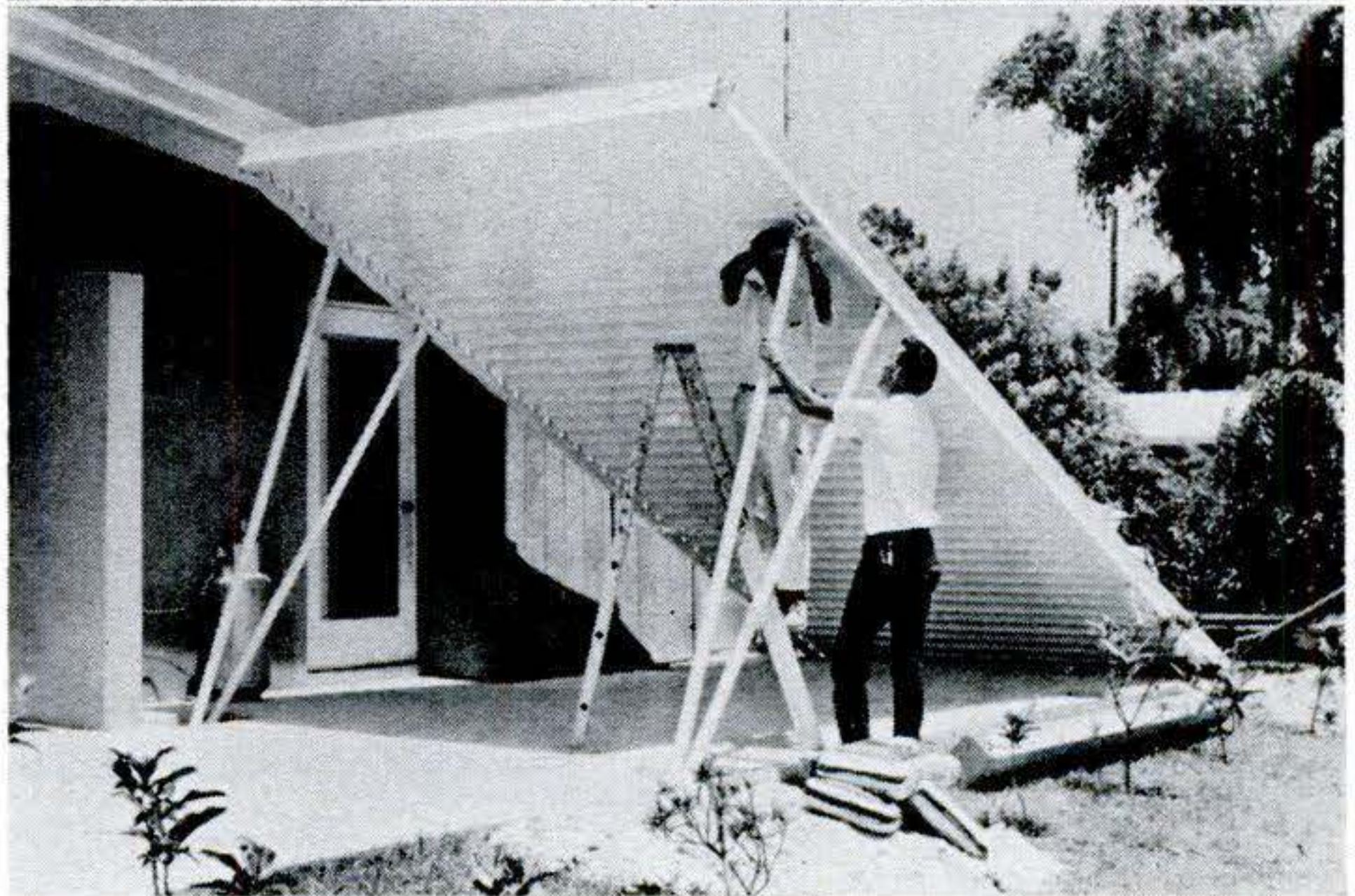
Flexalum Portiko gives you a carport or a patio roof fast. It comes in three sizes and can be erected free-standing or attached to a house. An integral gutter system can be drained at any point.
