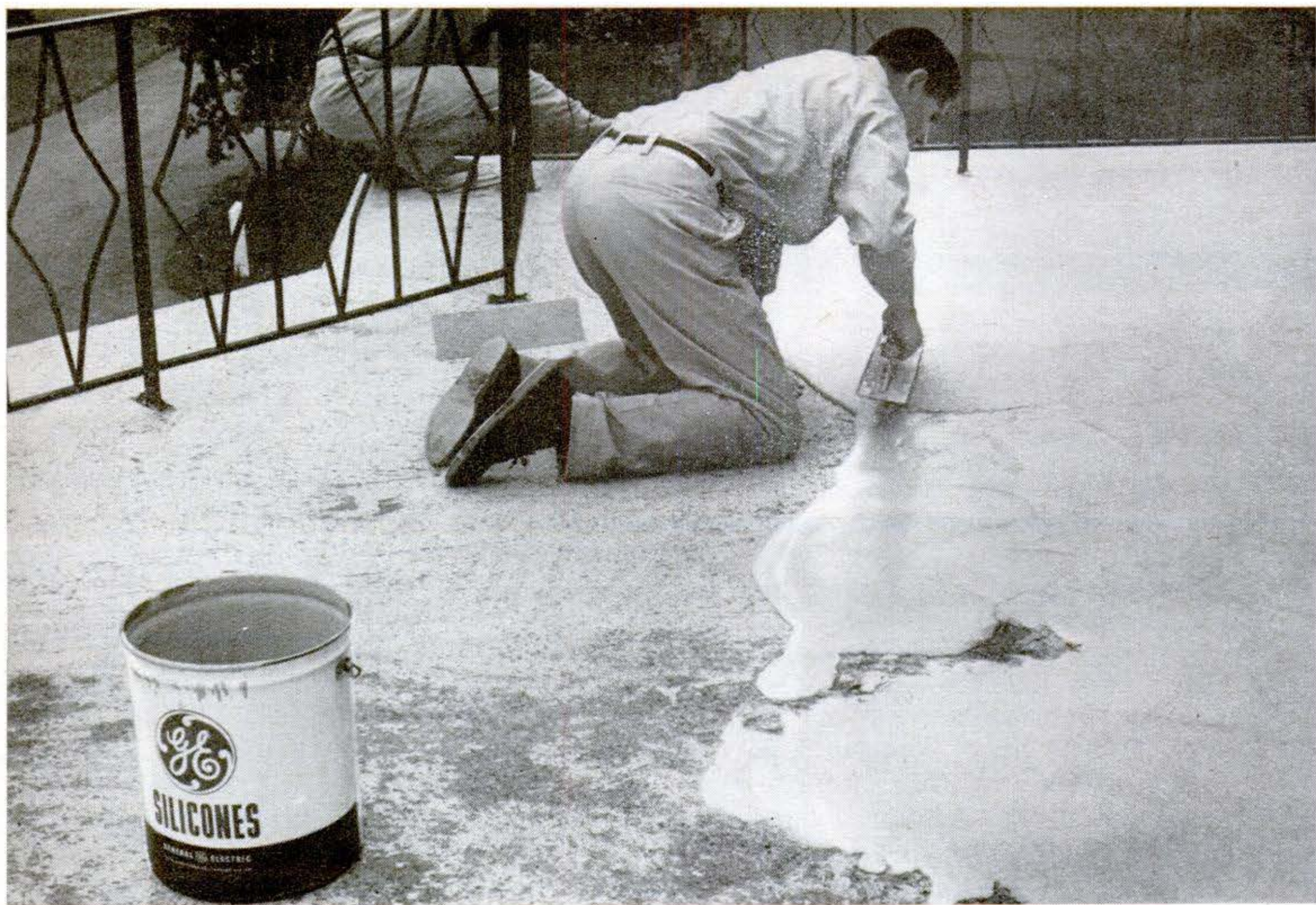
Repair your driveway or sun deck: GE's Traffic Topping, a silicone material mixed with grit, comes in
