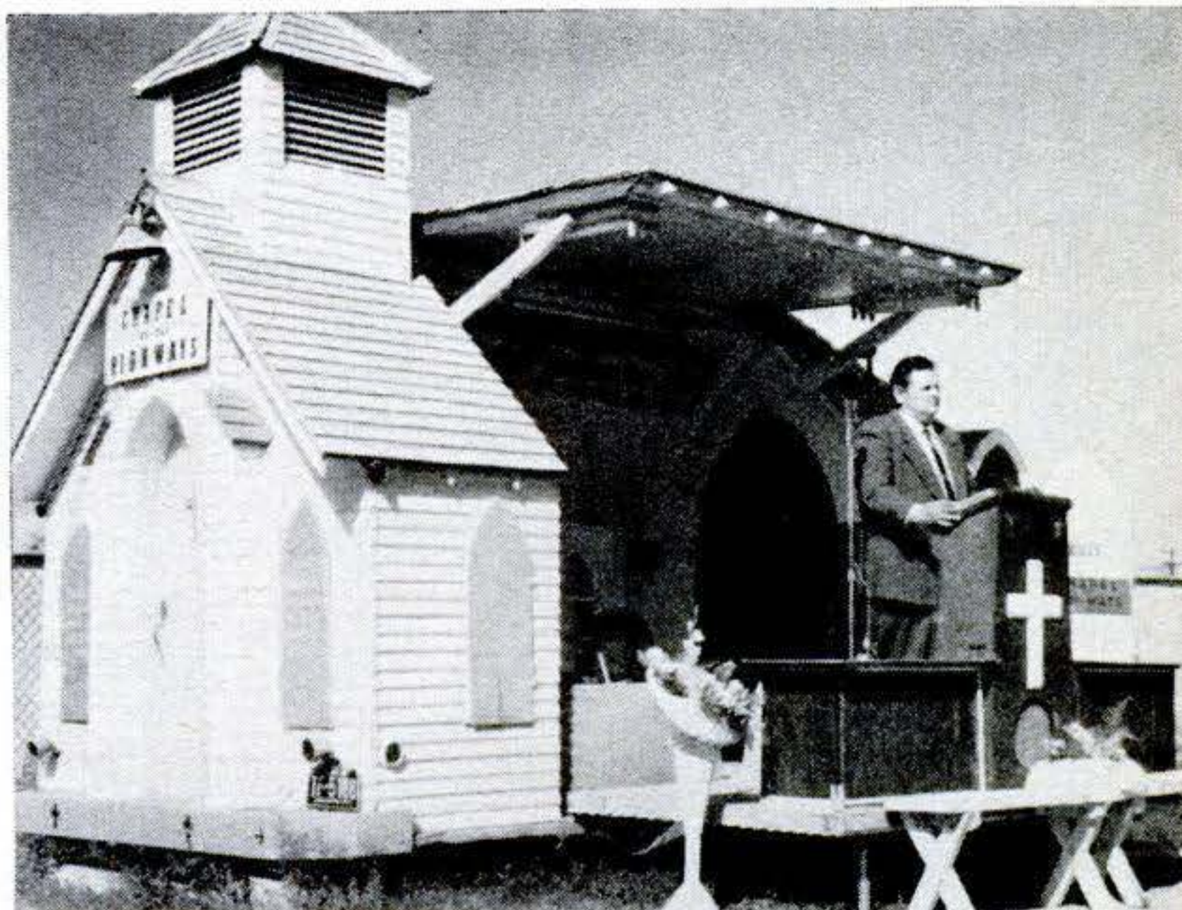
Trailer chapel resembles small country church when lowered to ground by jacks.
