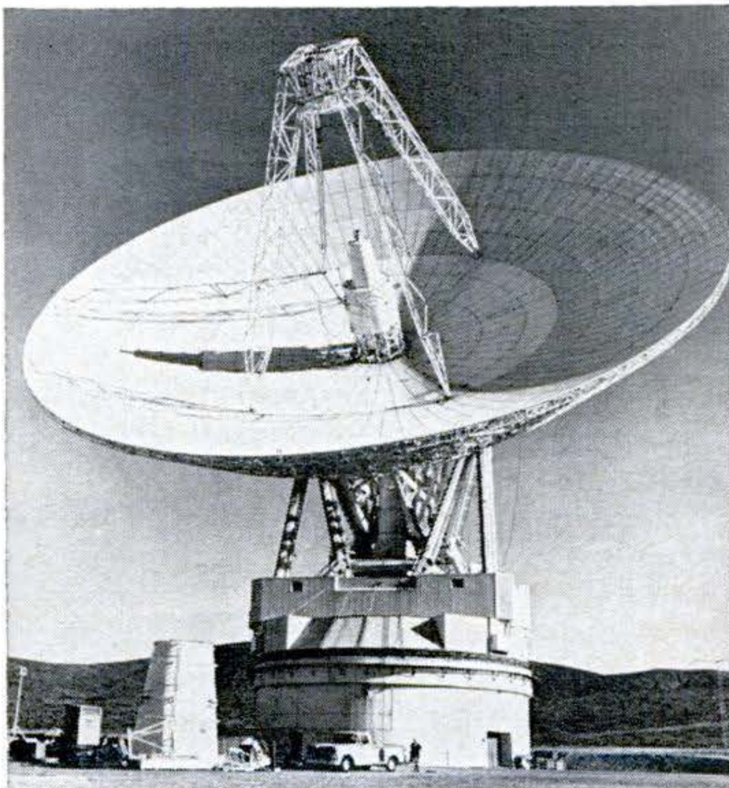
Photos from Orbiter, radioed across 240,000 miles of space, were picked up by huge antennas including this 210-foot-wide dish at Goldstone, Calif.
