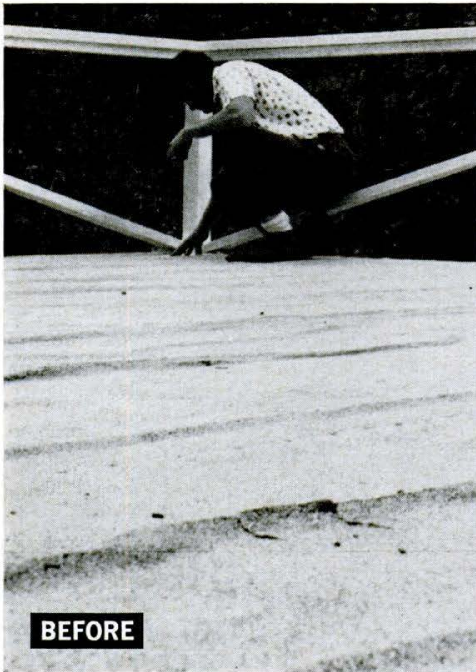
Old mineral-paper roof was buckled and leaking, but after the new material had been troweled
