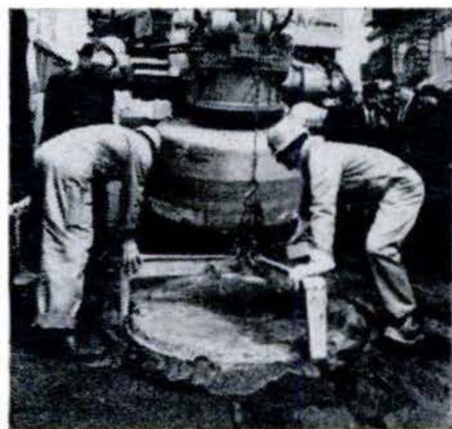
Workmen apply clamps to section.
