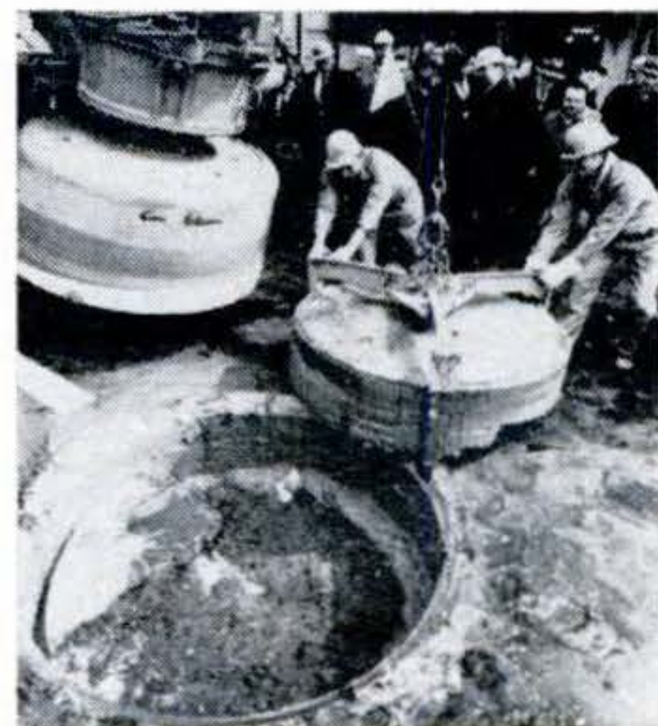
Huge slab is easily lifted out.
