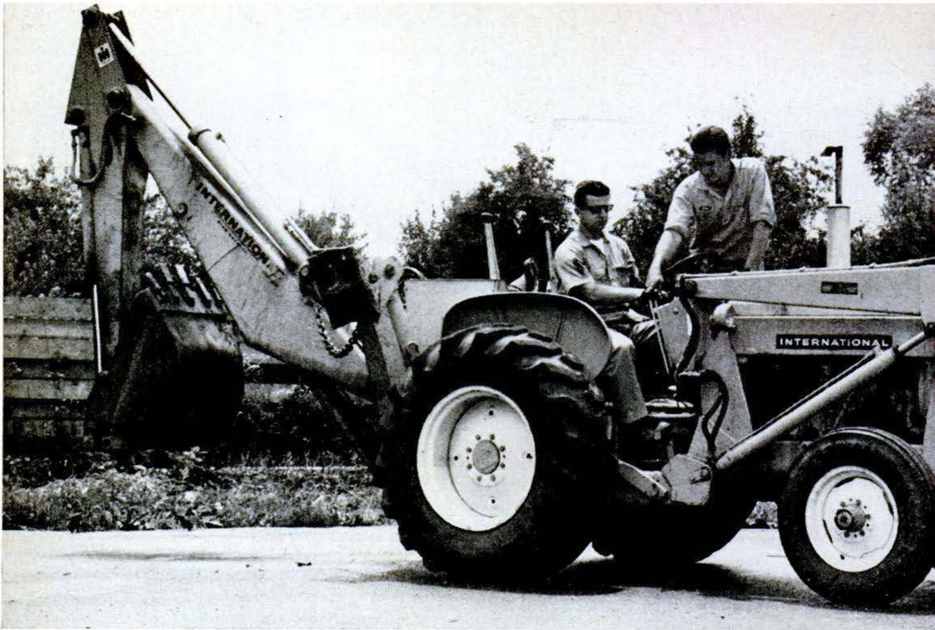
The author learns how to run a backhoe right on the rental dealer's lot. Brief instruction and
