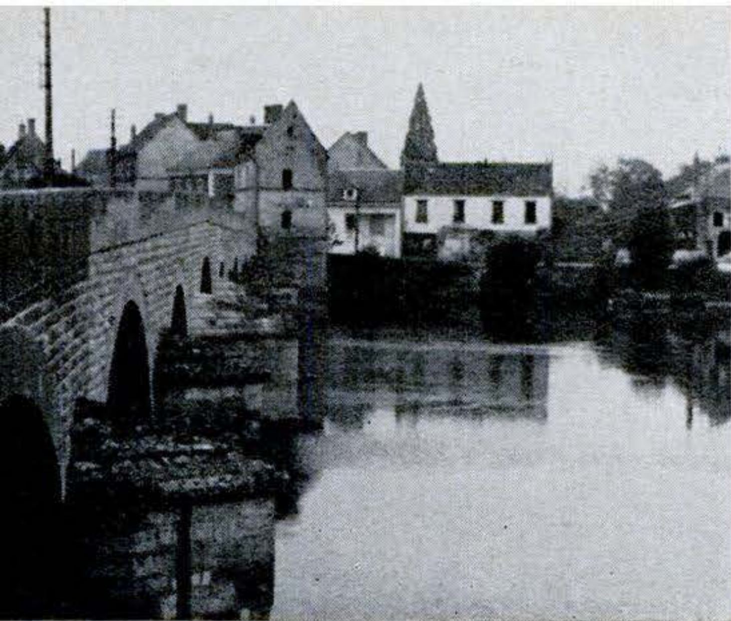
Effect of depth is created by bridge leading off into distance. Reflections on water help any picture.
