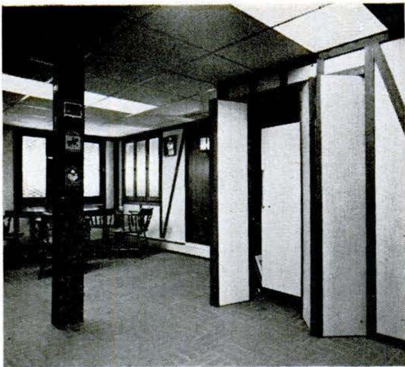
Rustic contrast is supplied by textured hardboard panels and walnut-stained pine battens filed and gouged for hand-hewn effect. Lally column is sheathed with similarly treated one-by-eights.
