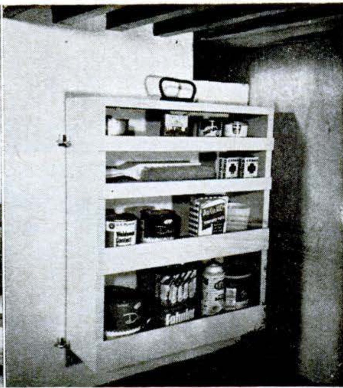
Portable swing-out shelf mounted on cabinet side gives storage for small items. For more storage, sacrifice portability; install several on slide-out track instead.
