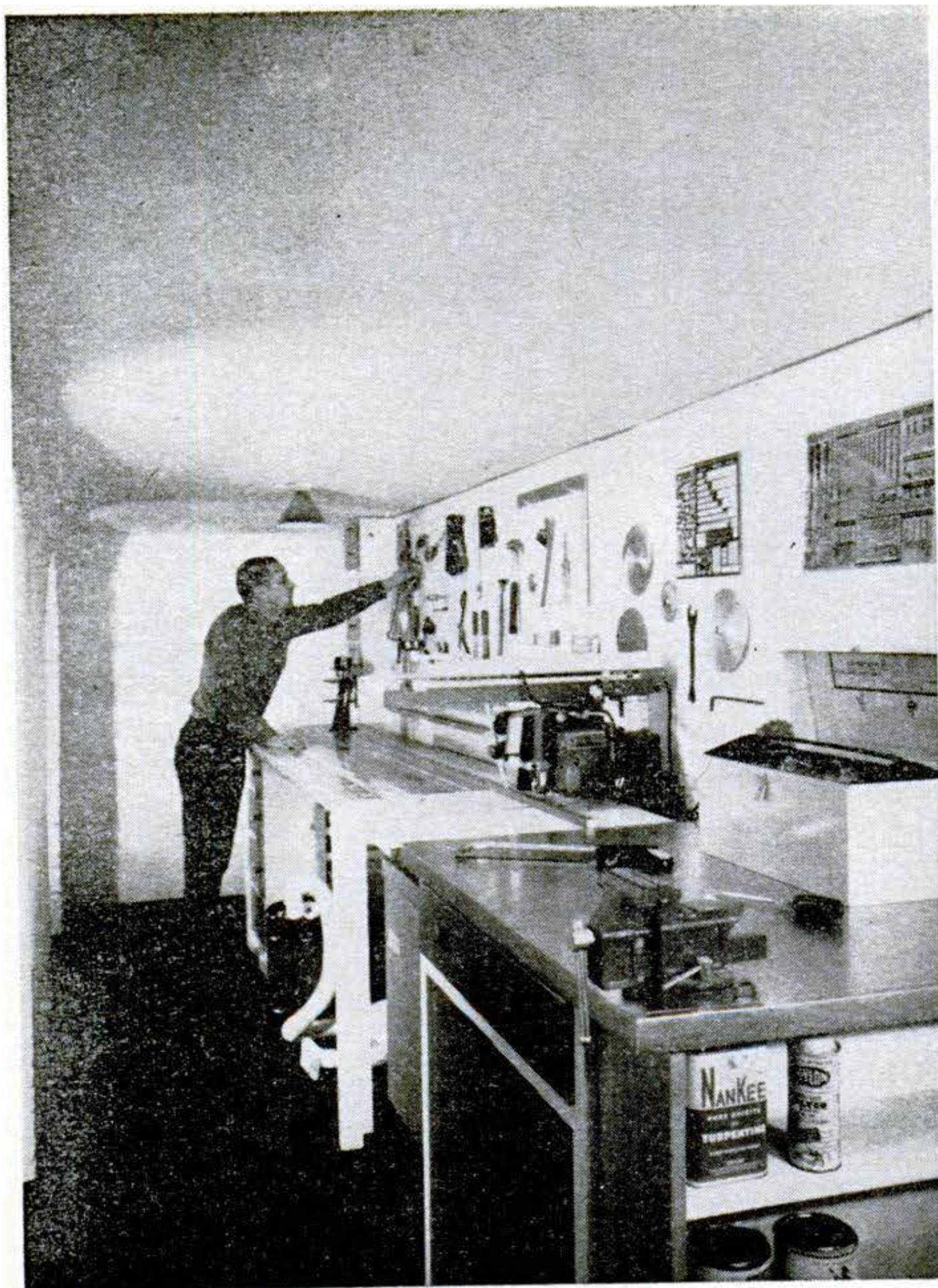
Narrow shop at left has plenty of worktop, ample storage. Drawers in cabinet (above) are built half-depth (see sketch at right) to limit their projection into walkway. Storage shelves are accessible from the side to utilize space behind the drawers.
