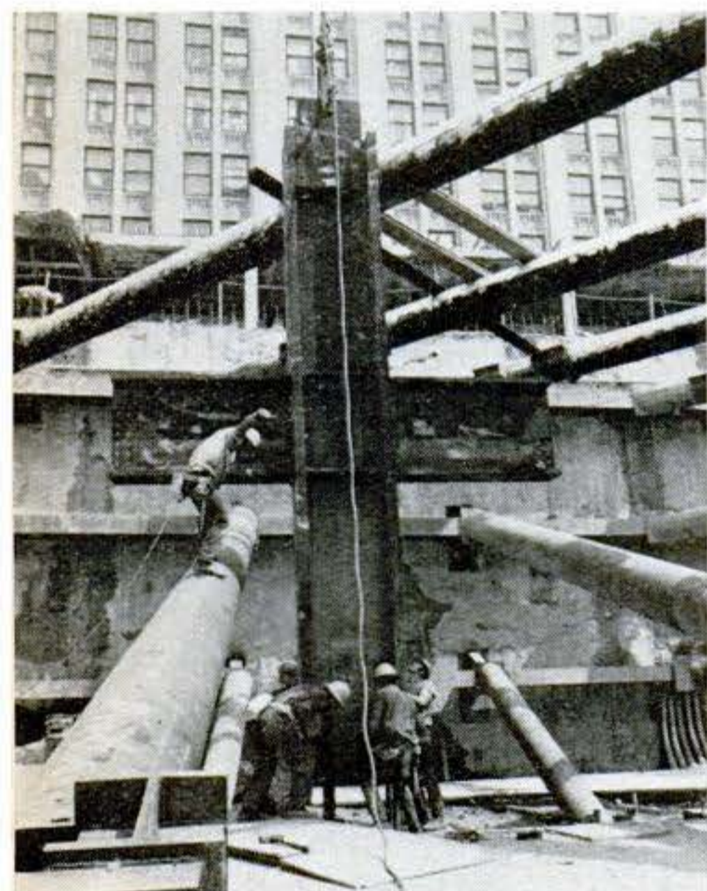
"Christmas trees"—the familiar name for the prefabricated columns—are erected by 40-foot stiff-leg creeper derricks, which climb inside walls of the steel framework.
