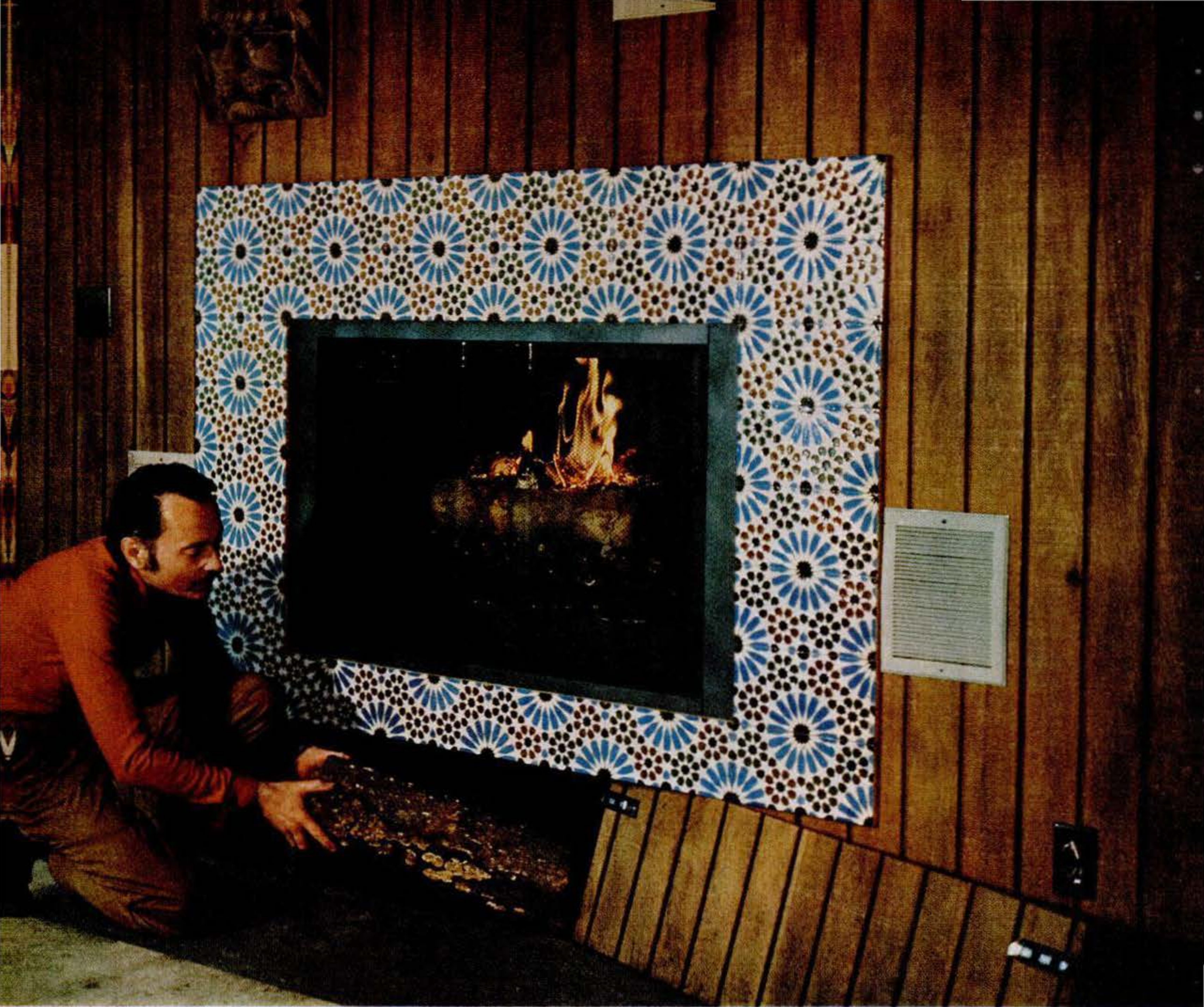
Platform installation let us tuck big woodbin under metal firebox. Raised hearth makes fire tending and grill cookery handier, too.
