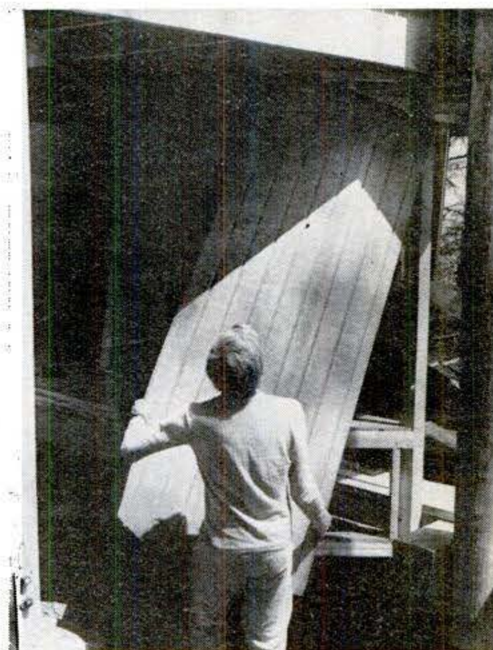
Same siding used on house encloses chase. It's Texture 1-11 plywood, Non-Com-treated by Koppers, Pittsburgh, to be fire-resistant.
