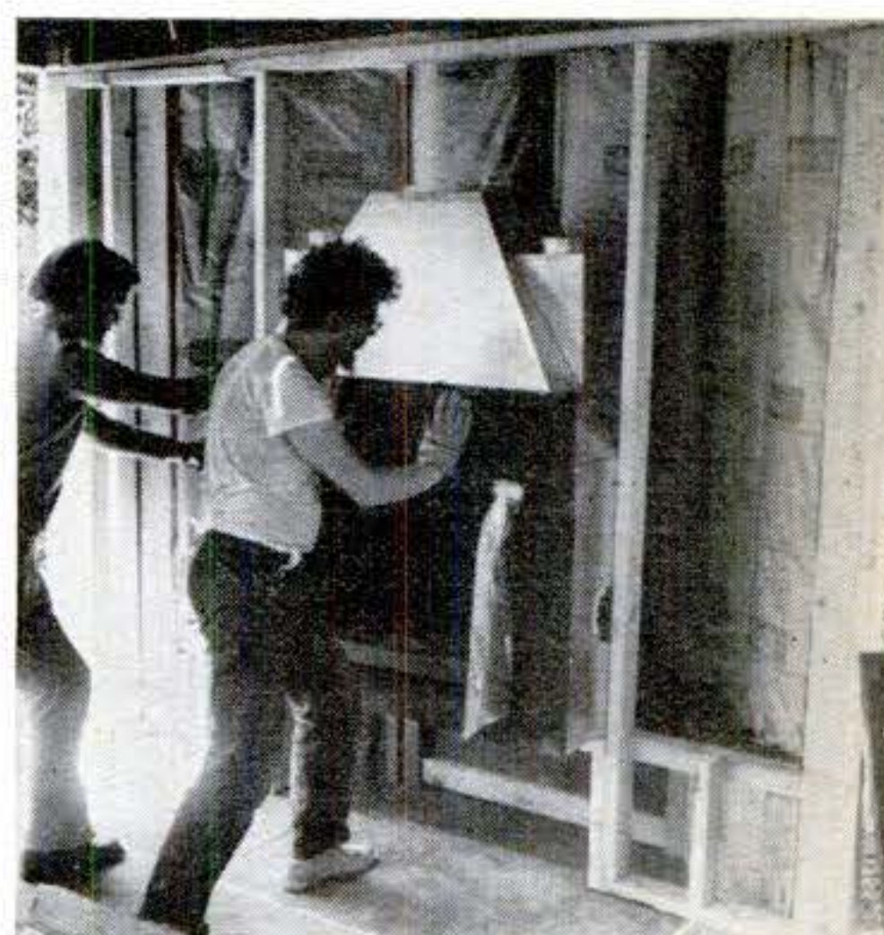
Metal firebox slips into place on platform. Note pre-scored side hole for inlet duct has been punched out at both sides.
