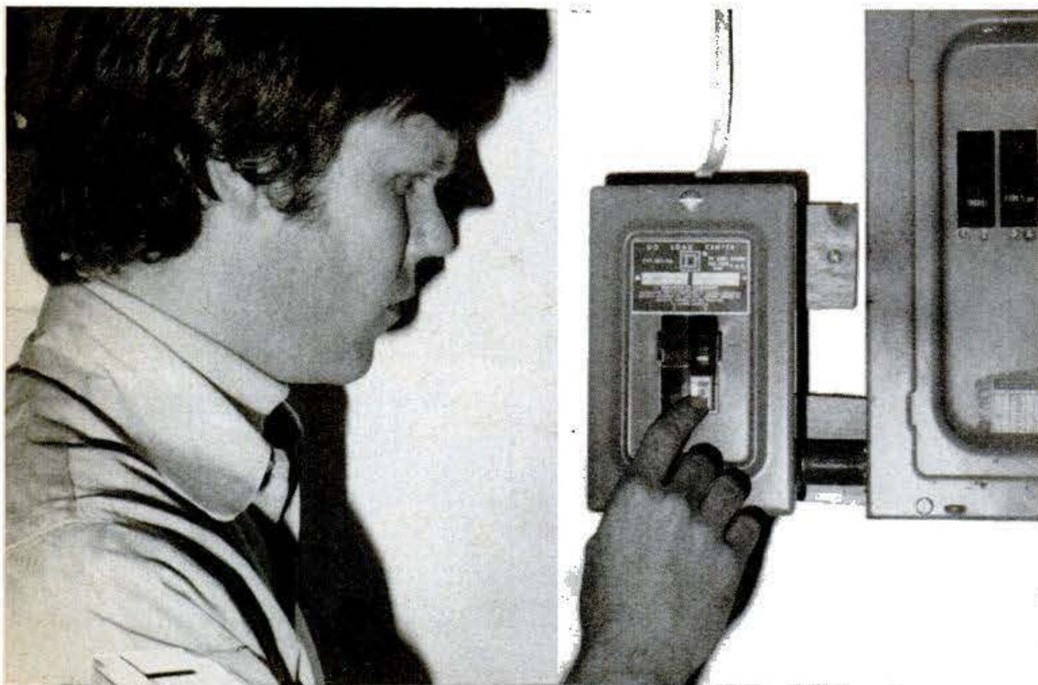
Quik-Gard from Square D replaces conventional circuit breakers. Test button simulates ground-fault condition, causing the breaker to open and indicator lamp to light.
