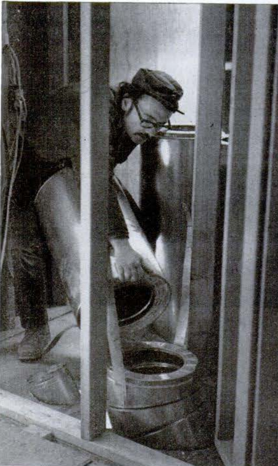
Chimney sections stack—and lock with twist—to extend upward from offset/return, which has support straps for nailing to adjacent studding. Smaller pipe to left is double-wall duct for upstairs heat outlet.
