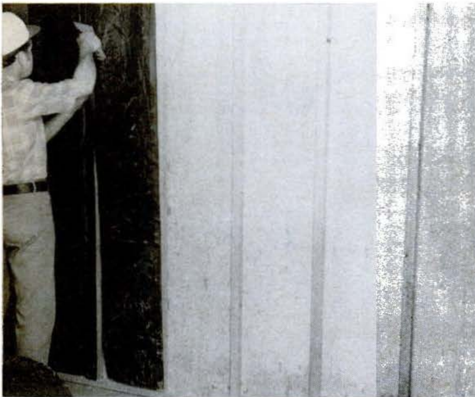
Special insulation batts for furred walls are stapled between two-by-two studs on outside walls—assuming masonry is sealed.
