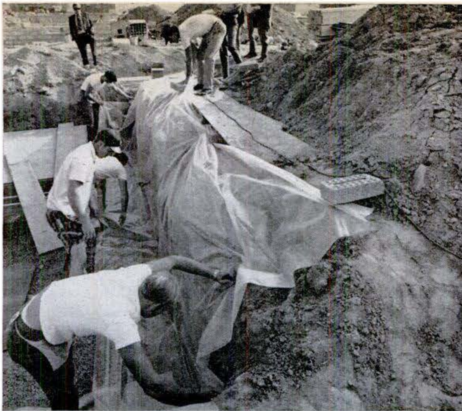
Polyethylene moisture barrier covers entire excavation floor and runs up sides of the hole, too. It prevents water seepage.
