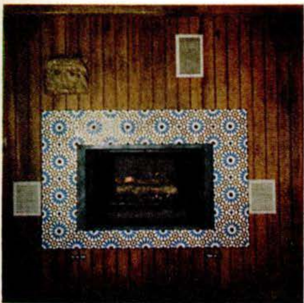
Platform installation let us tuck big woodbin under metal firebox. Raised hearth makes fire tending and grill cookery handier, too.
