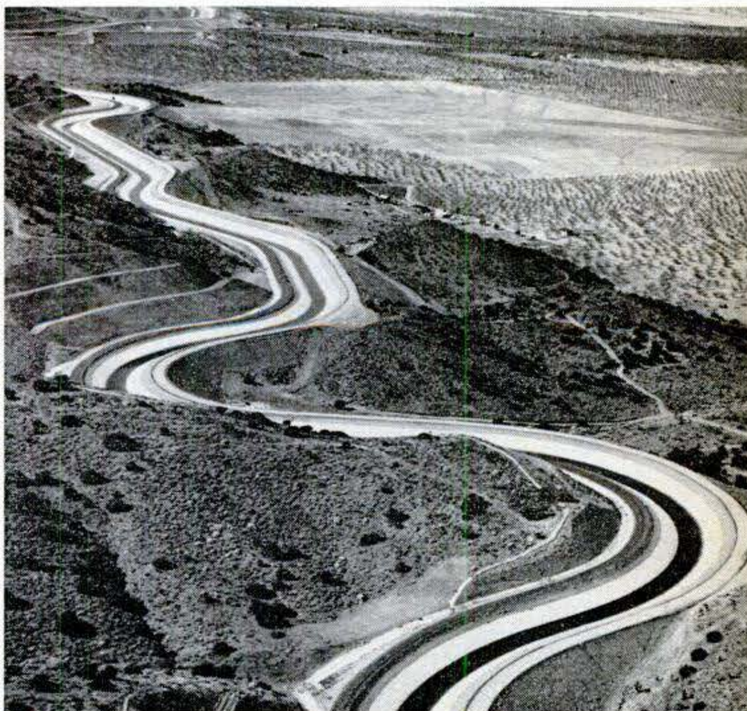
Aqueduct twists through Antelope Valley in Southern California.
