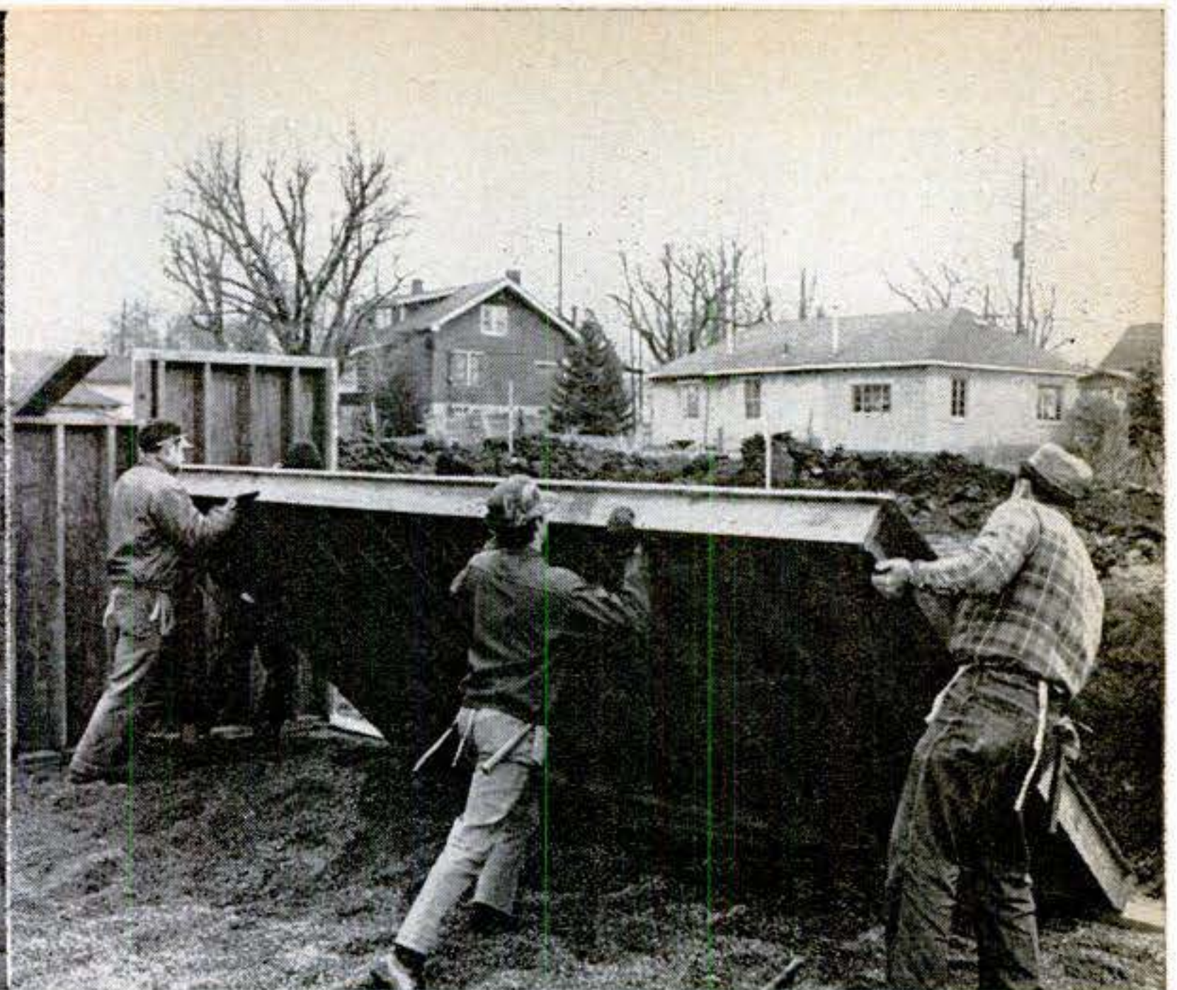
Foundation panels are assembled flat; then you lift them onto the footer plates and nail in place. All joints are caulked.
