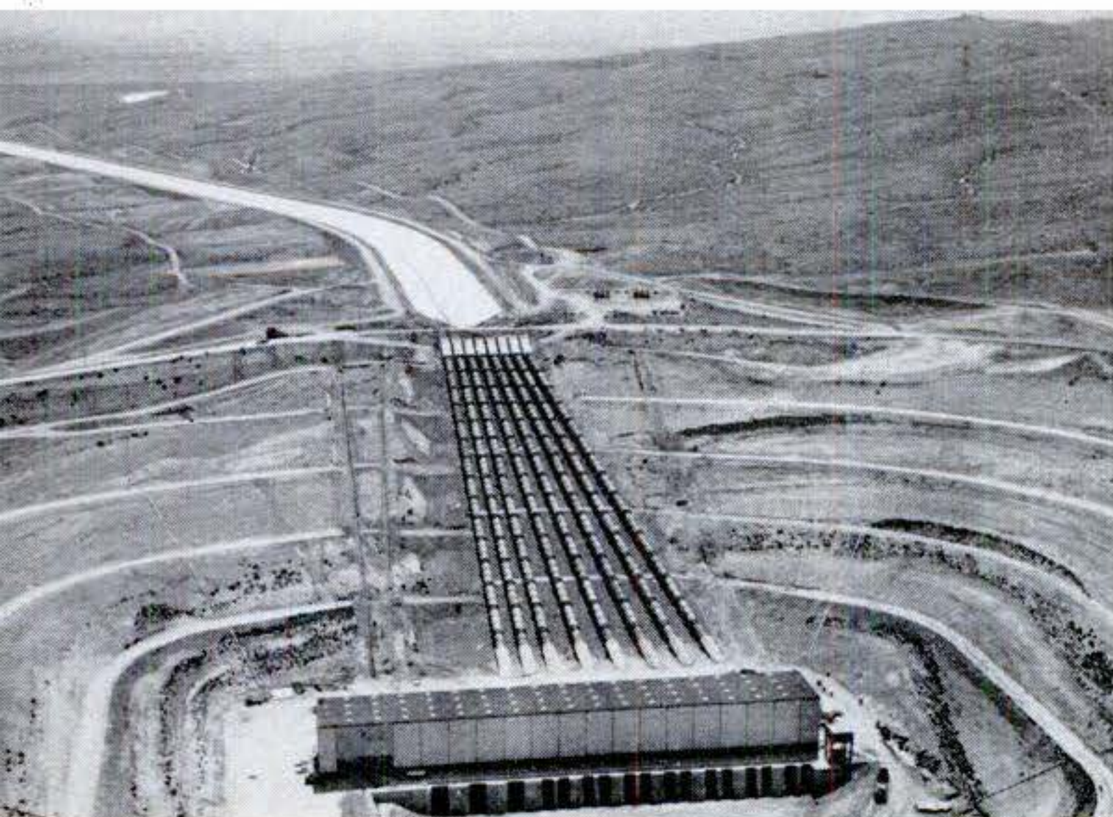
Discharge lines at Buena Vista station empty into aqueduct.
