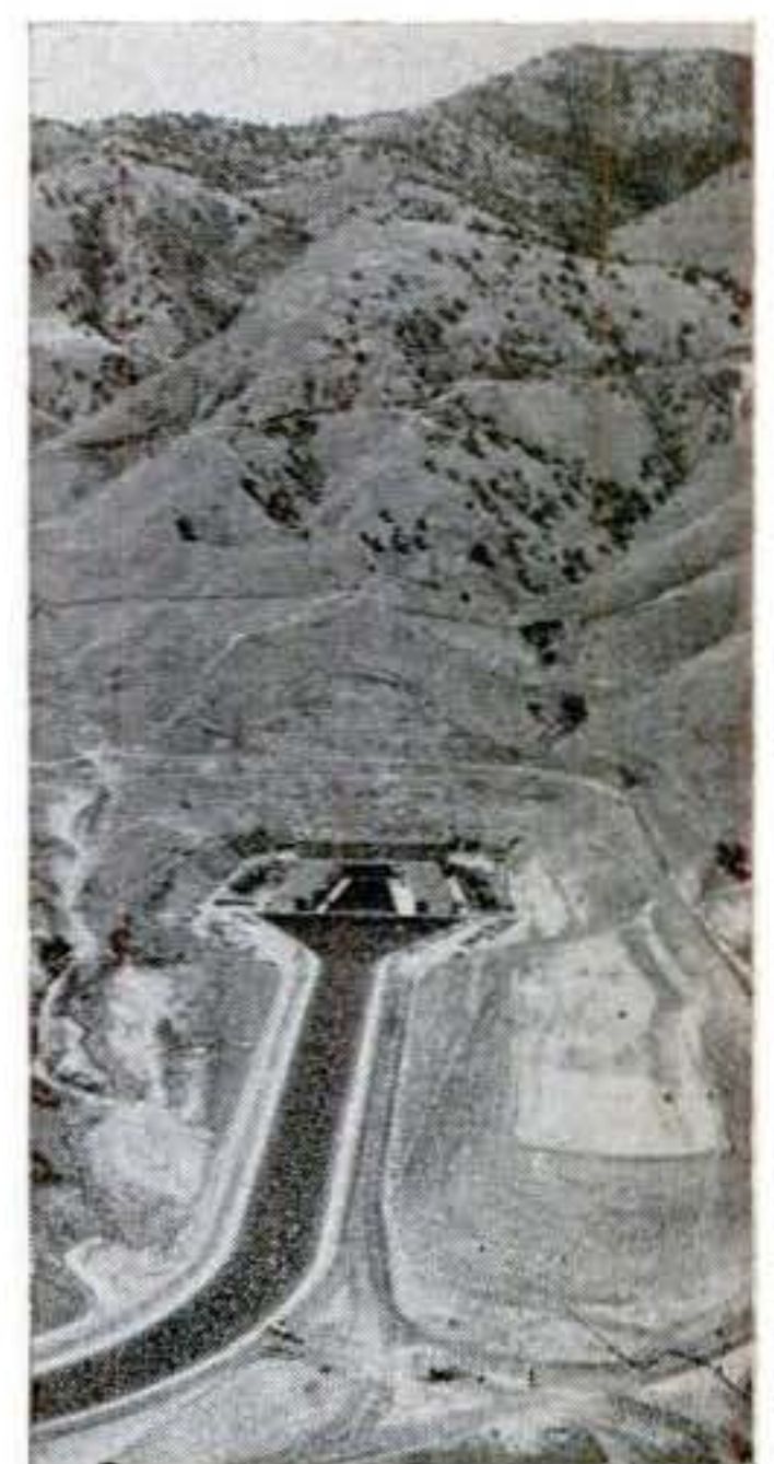
Link to Southern California along 444-mile-long aqueduct is U-shaped A. D. Edmonston Pumping Plant. Tehachapis loom over plant.
