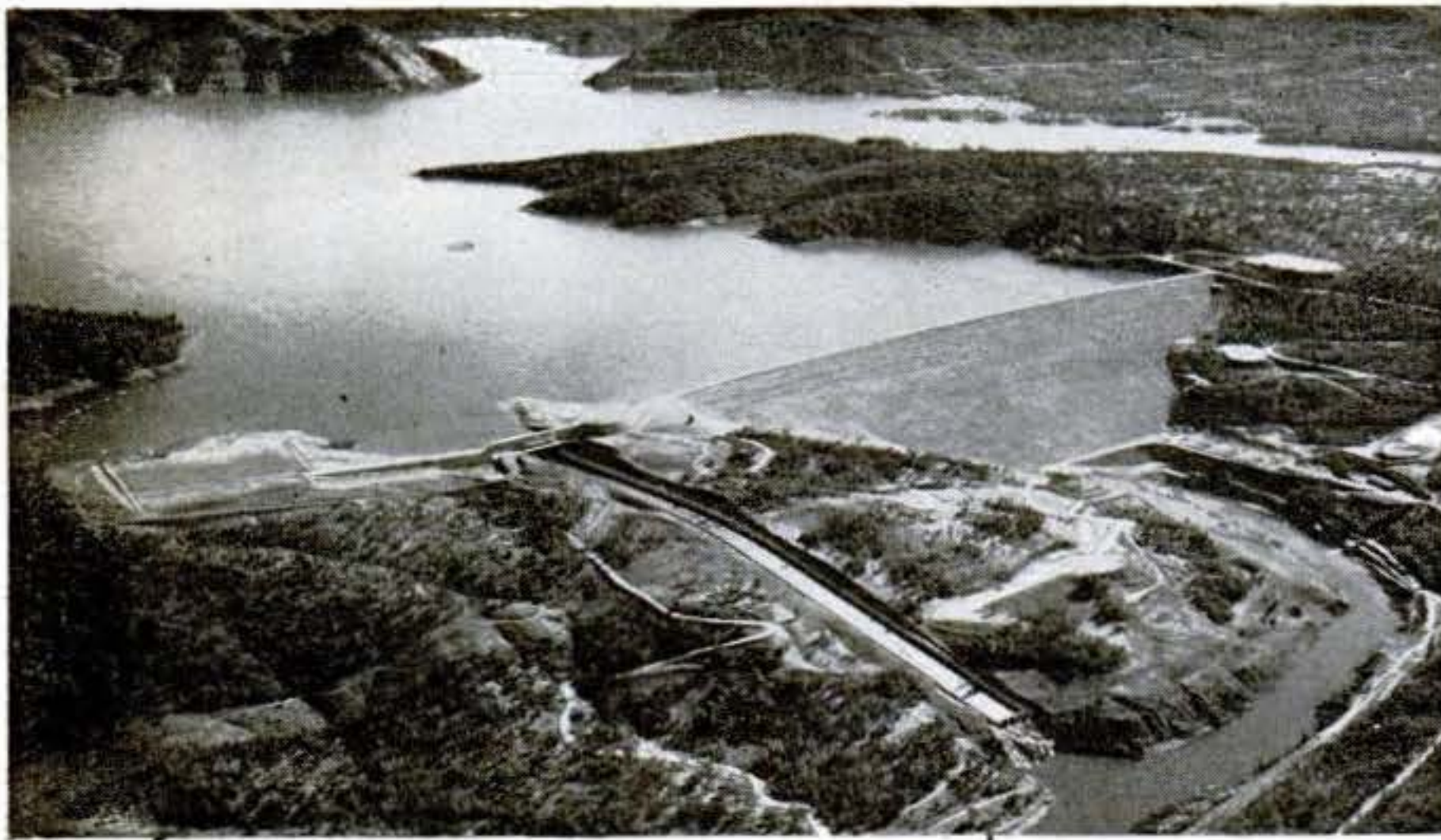
Northern reservoir for water is 15,800-acre Lake Oroville. At center: spillway for 770-ft.-high dam.
