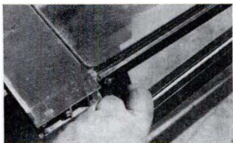
Remove metal edging —sides first, then top and bottom. You may need to tap them gently with a mallet and wood block. Peel off the gasket and keep for reuse.
