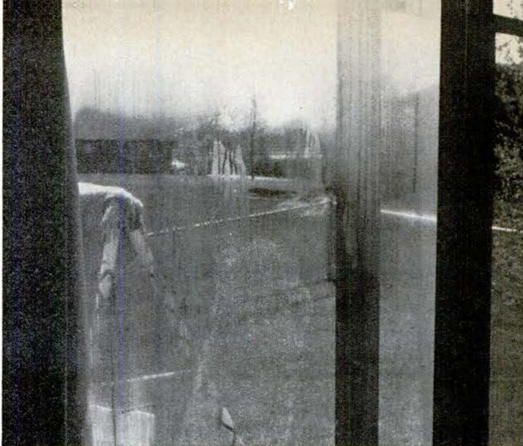
Unightly condensate between the panes of double-glazed patio doors can usually be cured with a low-cost home remedy.
