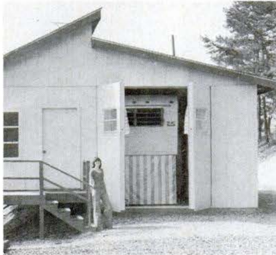
support the heavy doors. To preserve the illusion of an unbroken exterior, the knobless door opens only from the inside.
