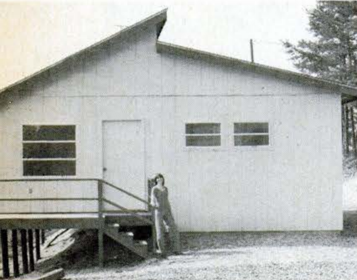
Hidden doors blend into house wall (above) but swing smoothly open (right) for RV exit. Specially designed hinges
