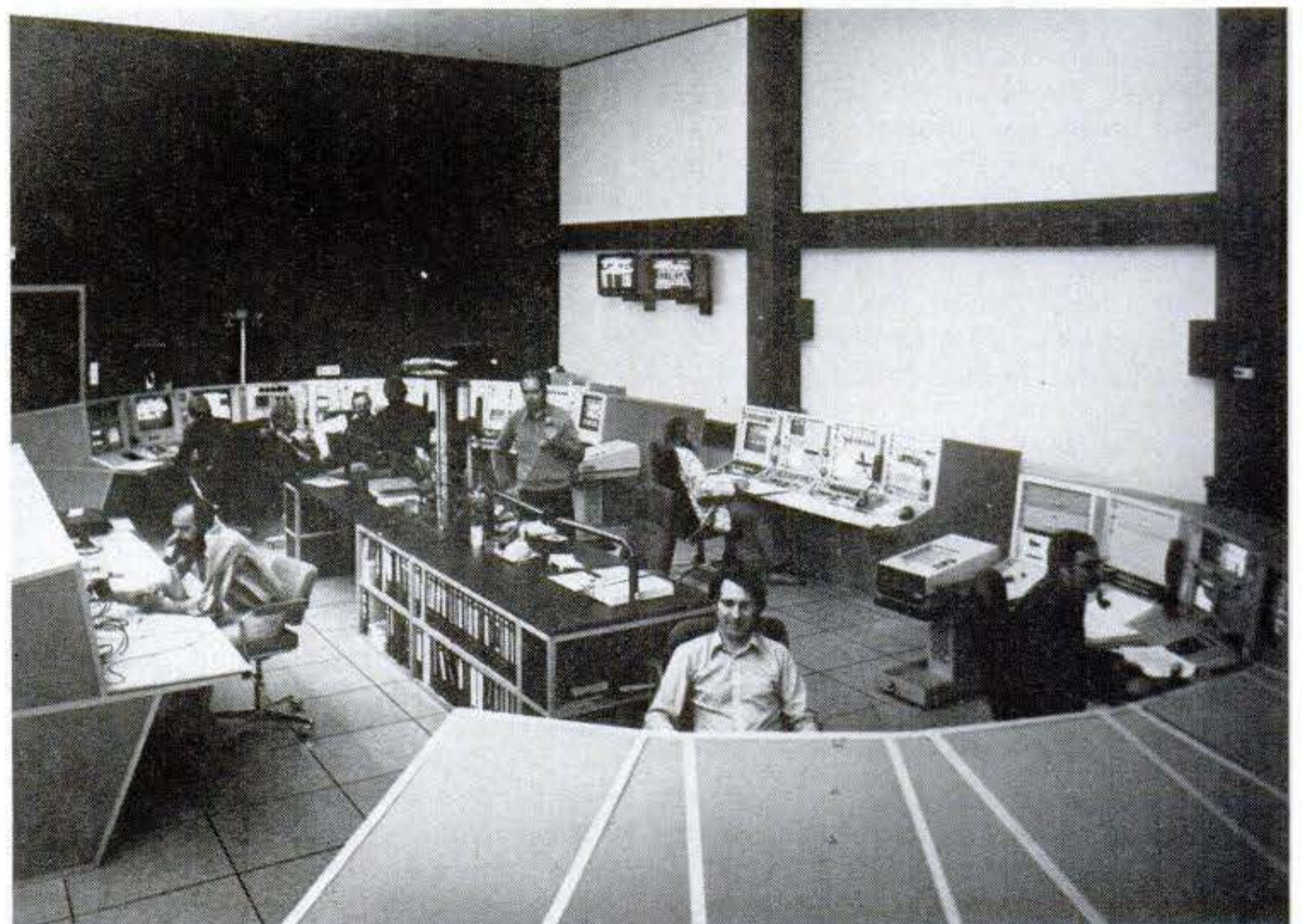
Control rooms at the Super Proton Synchrotron CERN installation in Switzerland
