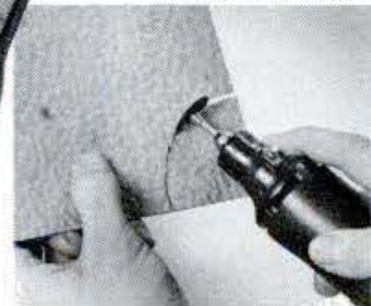
Cut floor tile.
