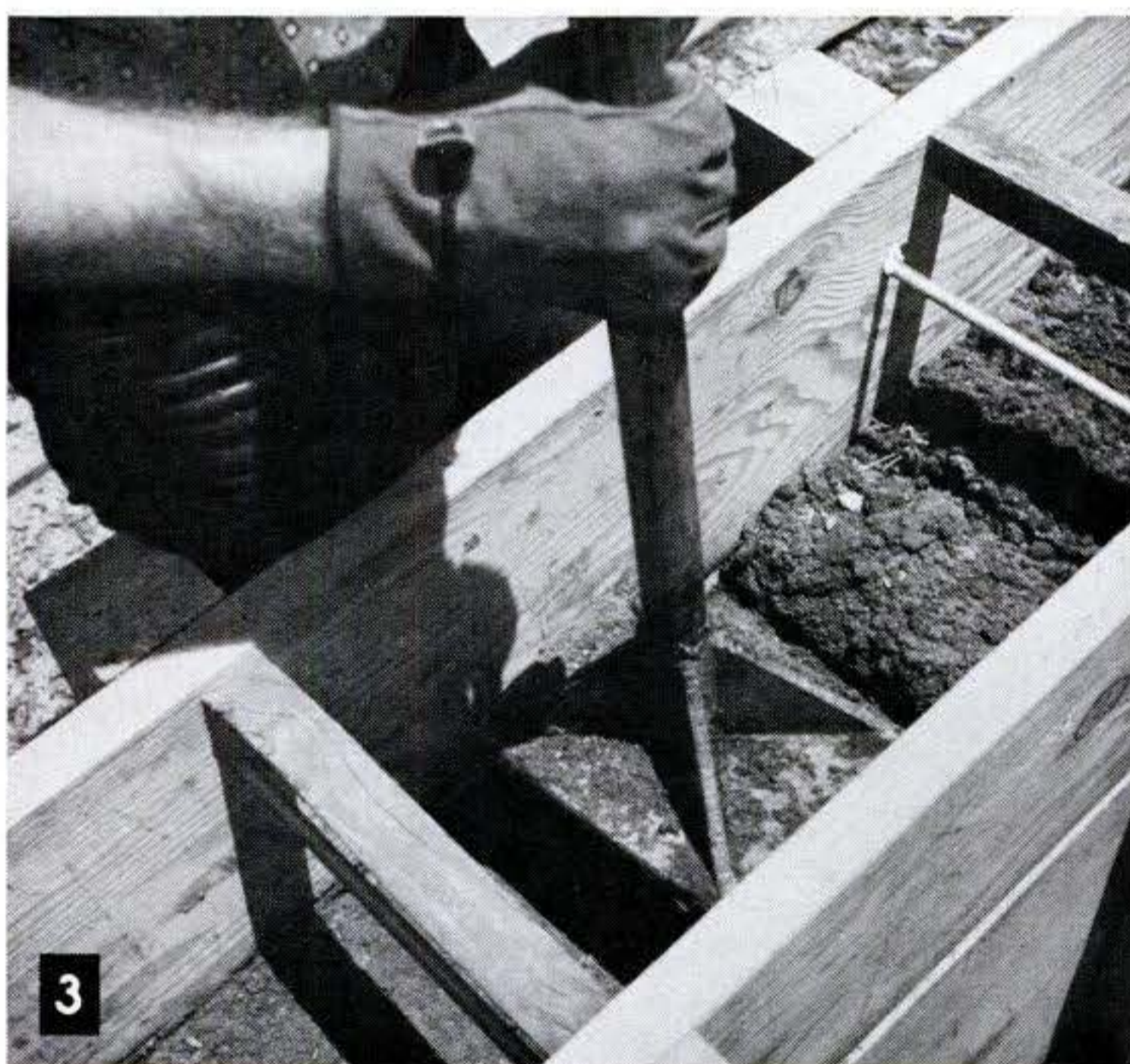
Steps in rammed-earth-wall construction: Form is built atop a concrete foundation (1); loose soil at optimum moisture content
