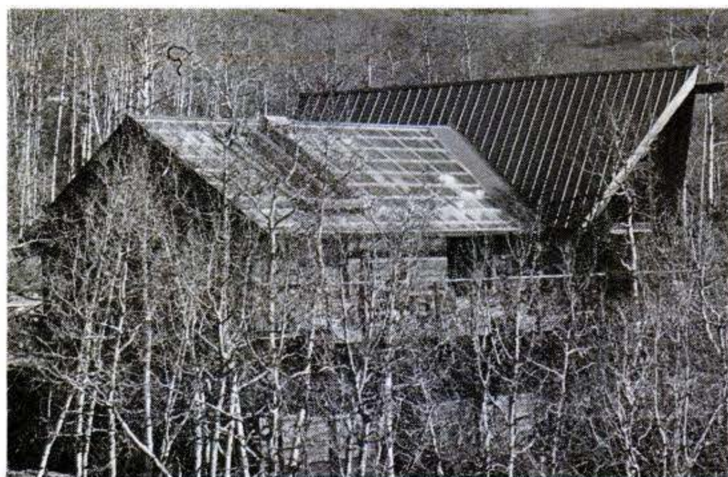
Roof collector is south face of one wing of this mountain home, covered with corrugated FRP. Hot air in space beneath is pumped into rock storage bin and distributed to living areas.
