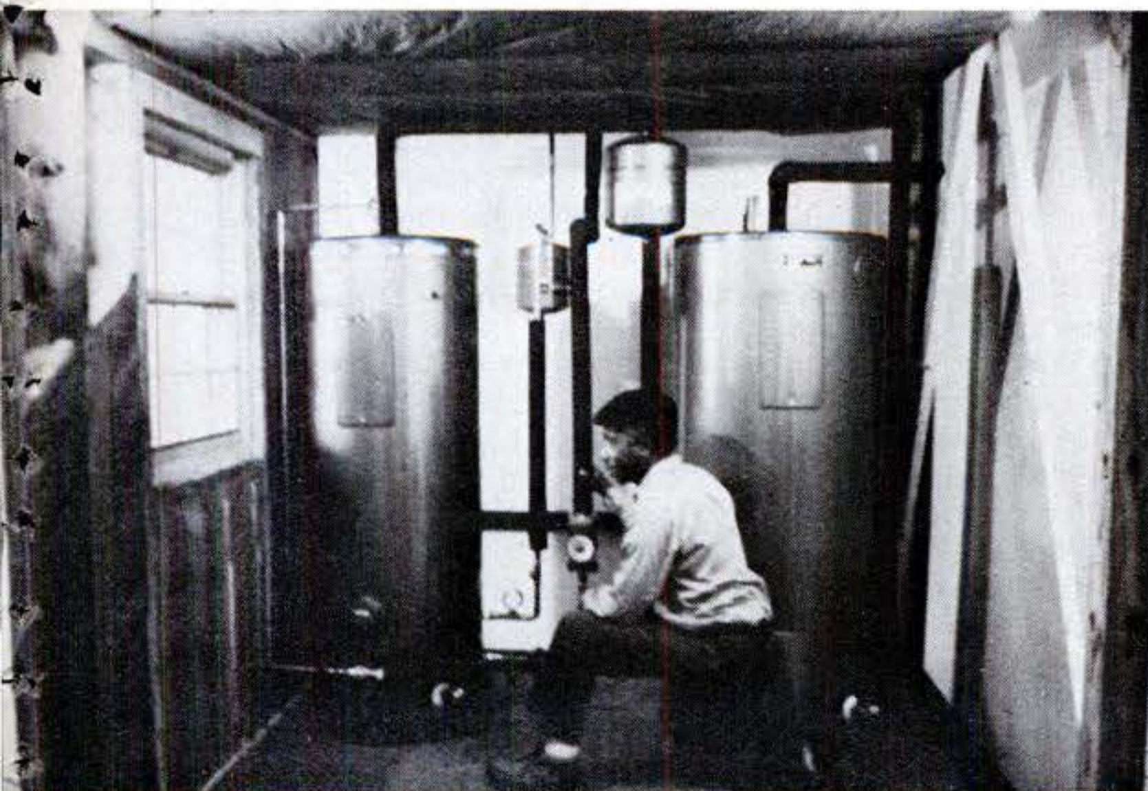
TVA's secret: two storage tanks. To shave grid peaks, timer prevents daytime electrical charging of backup tank. Second tank
