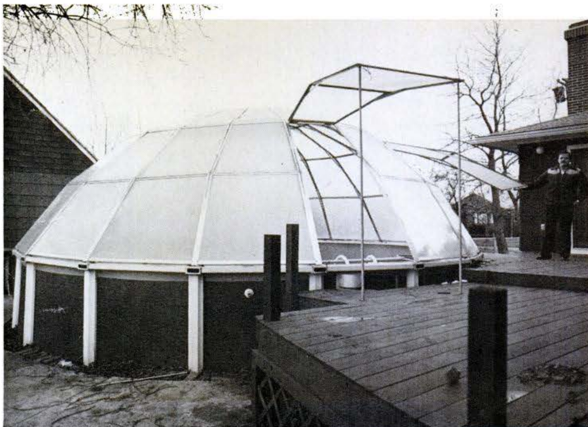
Pool dome, supported by shroud assembly of aluminum angles, has two hinged
