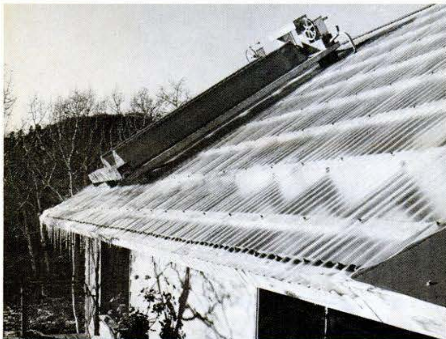
Roof collector is south face of one wing of this mountain home, covered with corrugated FRP. Hot air in space beneath is pumped into rock storage bin and distributed to living areas.
