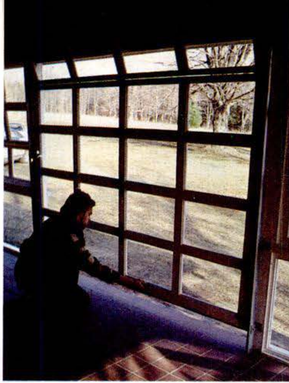
Central entry span is glazed with overhead door that tracks up under the roof. Flanking it: tri-fold windows that store along eaves (end-wall type, right).
