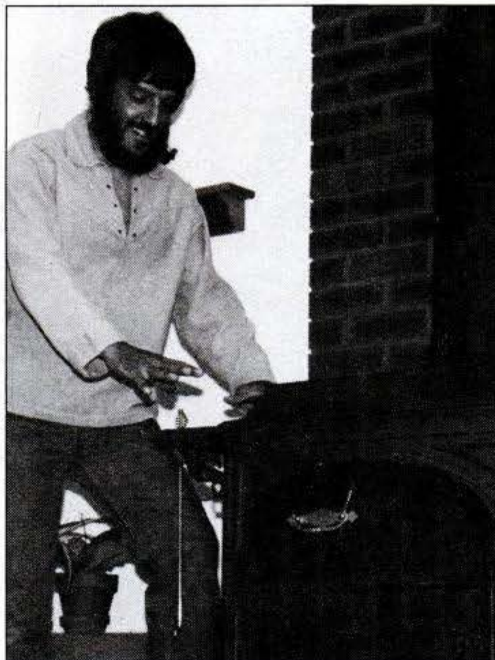
Heat from Pina's wood stove (above) flows through gas furnace's ducting.
